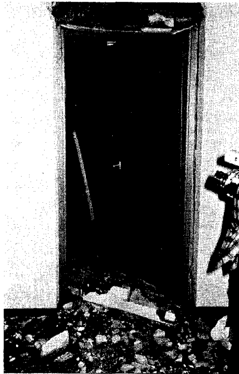
Fig. 67. Lintel over Door Racked by Shearing Forces
