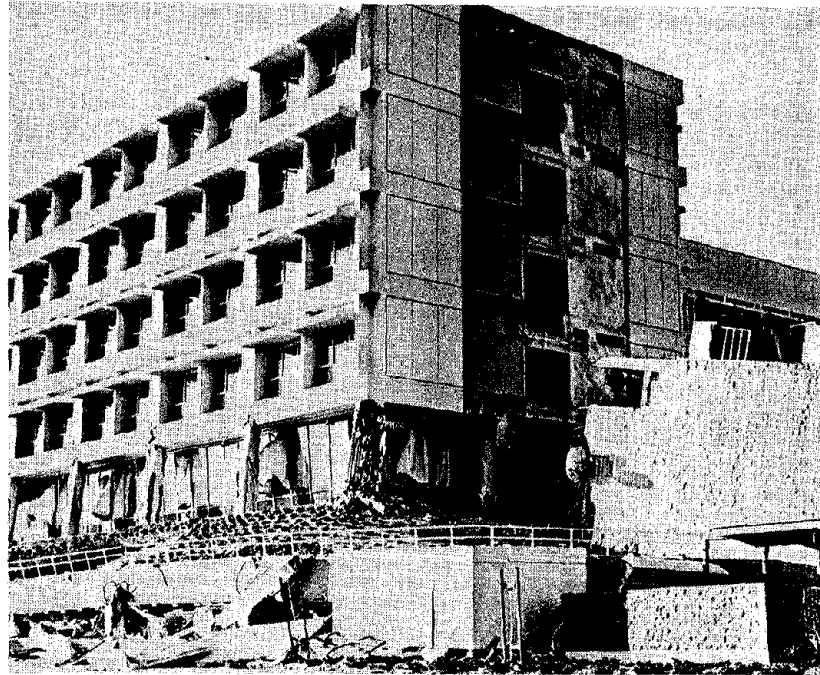
Fig. 53. "Open First Story" Failure; Columns Crushed
