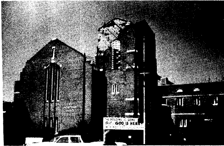
Fig. 72. Failure of Brick Veneer
