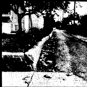
Fault Creep Hollister, Calif.
