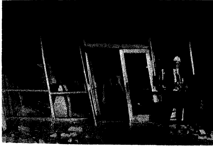
Fig. 80. Racked Glazing Frames
