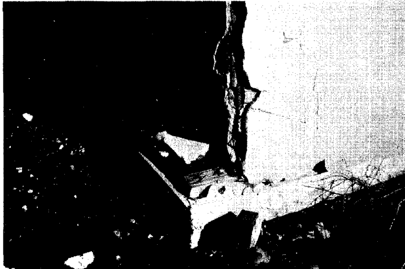
Fig. 61. Inadequate Anchoring of House to Foundation
