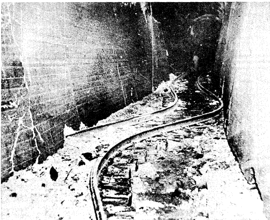
FIGURE 3—This railway tunnel in southern California passed through the fault zone of the 1952 Tehachapi, California, earthquake of July 21, 1952. Rock movements produced by faulting shattered the tunnel.
