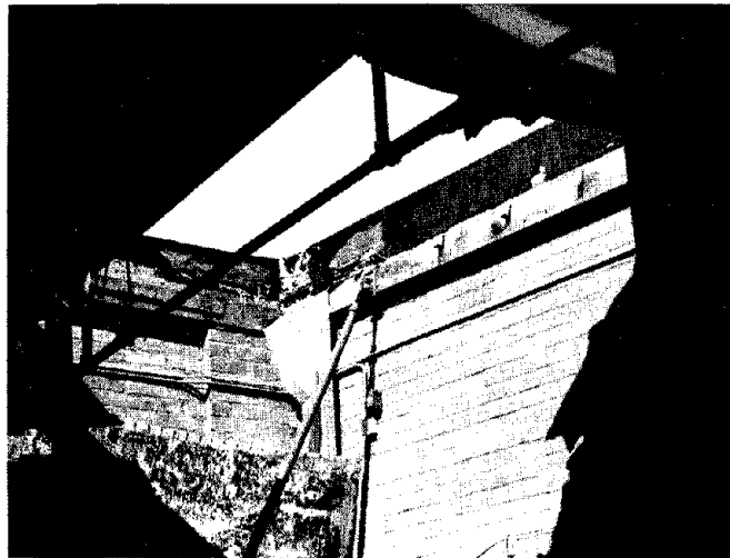
Figure 8 The influence of the corners of masonry walls on the performance of horizontal diaphragms should be examined.
