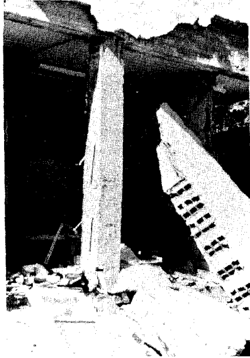
Fig. 17 Detail of Sylmar building showing spalling at top of column.
