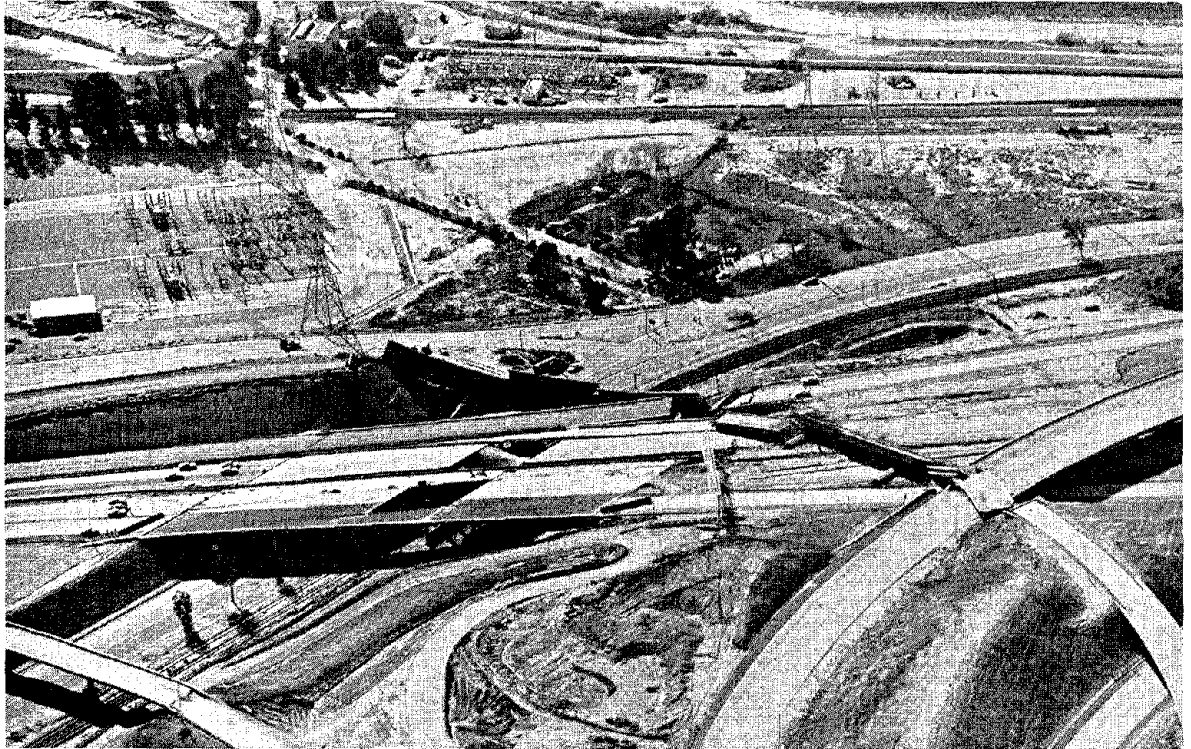
Figure 16. Collapsed freeway overpasses and freeway interchange bridge in Sylmar following the San Fernando earthquake. The estimated peak ground acceleration was approximately 0.5g. The design criteria for these structures were inadequate for such strong ground shaking.
