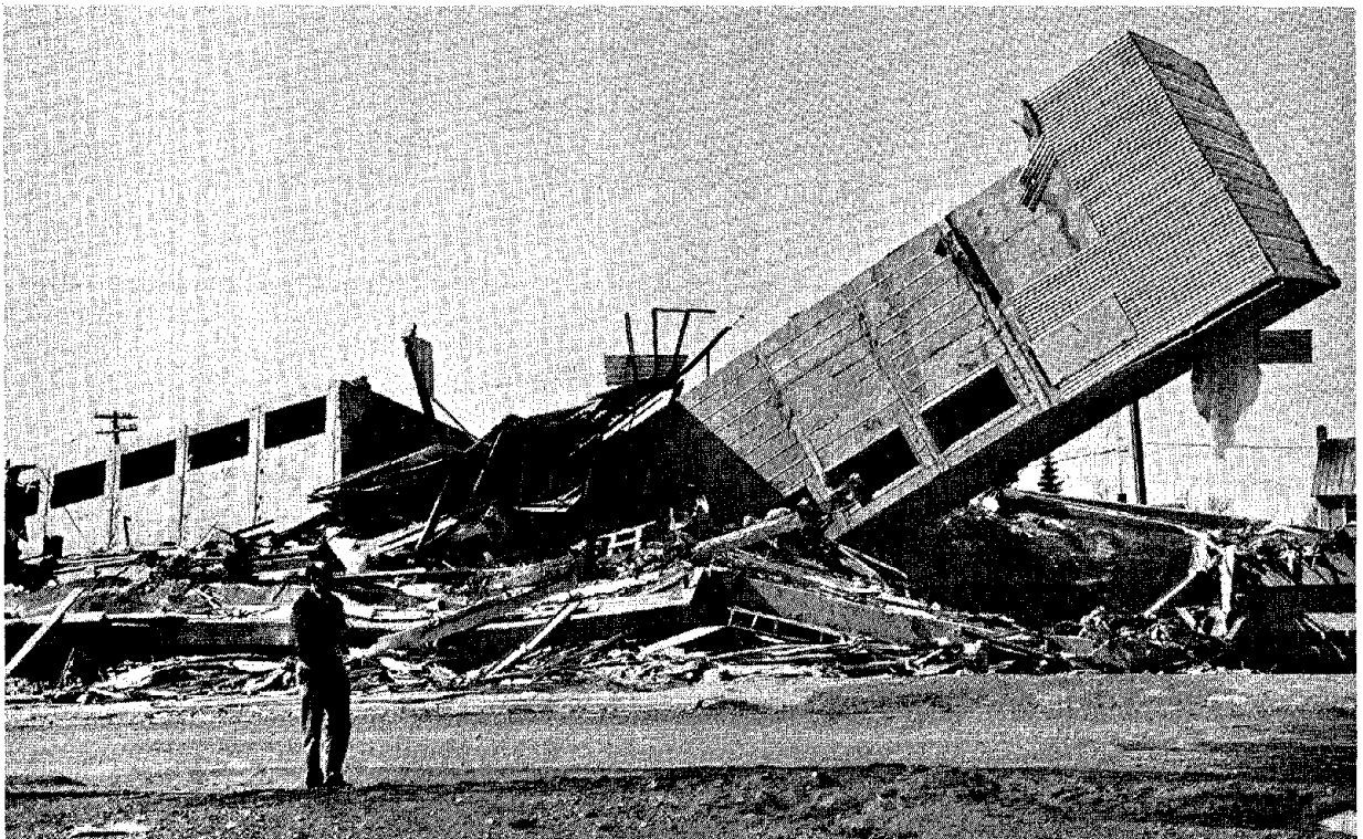
Figure 15. Six story lift-slab Four Seasons Apartment Building in Anchorage following the 1964 Alaska earthquake. It is estimated that the spectral acceleration of the ground motion was approximately 0.4g at .5 secs. and 5\% damping. Lateral resistance was provided by the two towers but their connection to the footings was deficient, lapping of bars 20 diameters, and failure occurred at approximately one-half of the bending capacity as determined by the area of the reinforcing bars.
