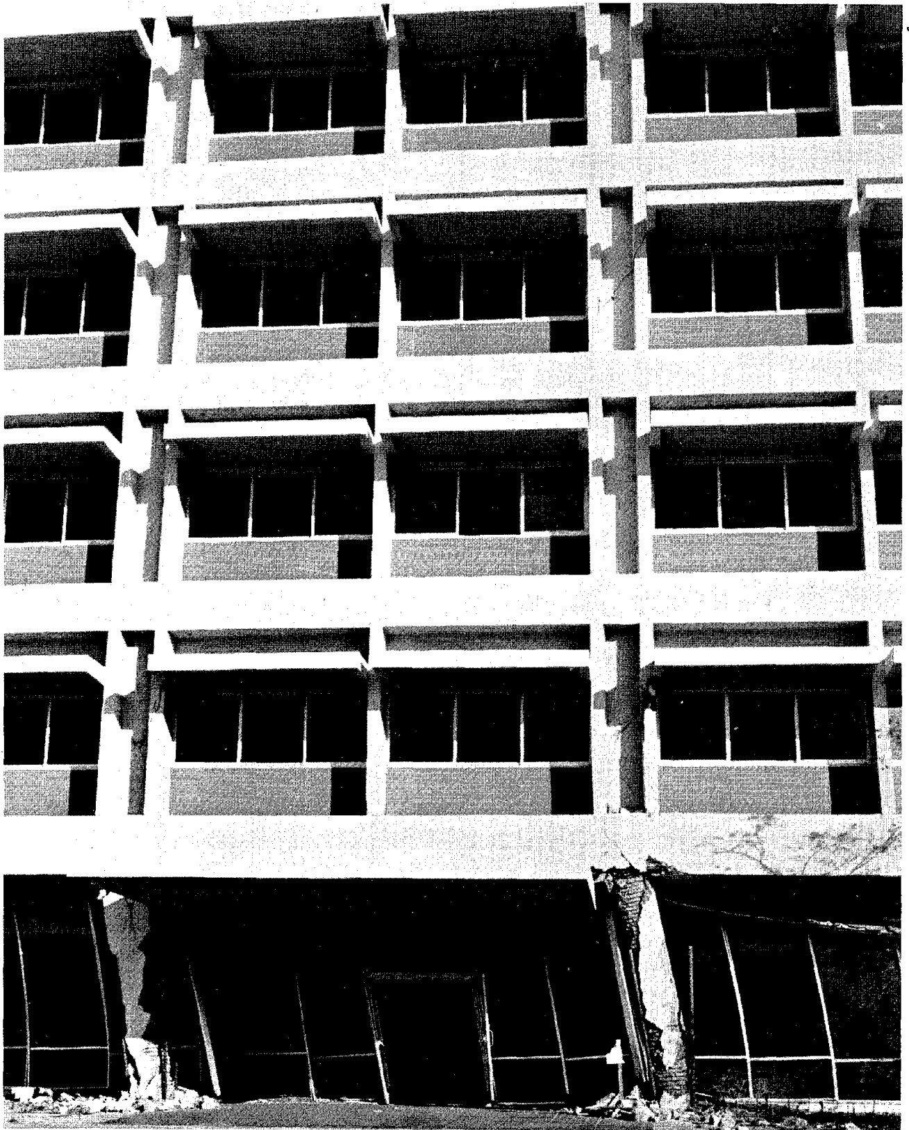
Figure 11. Olive view Hospital after the San Fernando earthquake. The spirally reinforced columns were severely deformed with interfloor displacements of 50 or more times the yieldpoint displacement. Estimated peak ground acceleration was approximately 50\%g and the corresponding elastic response spectral acceleration is 1.2g for 0.5 sec period and 5% damping; the corresponding first-mode base shear during the earthquake was governed by the maximum yield moment of the columns.
