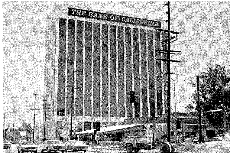
Figure 6. The 12-story California Bank Building after the San Fernando earthquake. This concrete frame building experienced appreciable cracking of beams and columns. The peak ground acceleration during the earthquake was .23g and the maximum base shear in the first-mode was 3.2 times larger than the nominal code value of base shear. (N 11° E motion)
