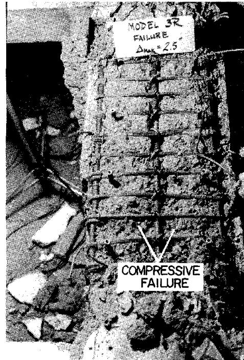
FIG. 3.21 COMPRESSIVE FAILURE AT END OF MID-DEPTH LONGITUDINAL CRACK IN MODEL 3R (1 IN. = 25.4 MM)
