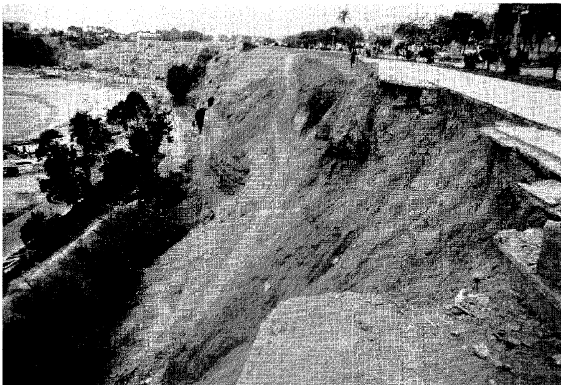
Landslide in dry slightly cemented silty sand in steep cliffs at Lima, Peru.
