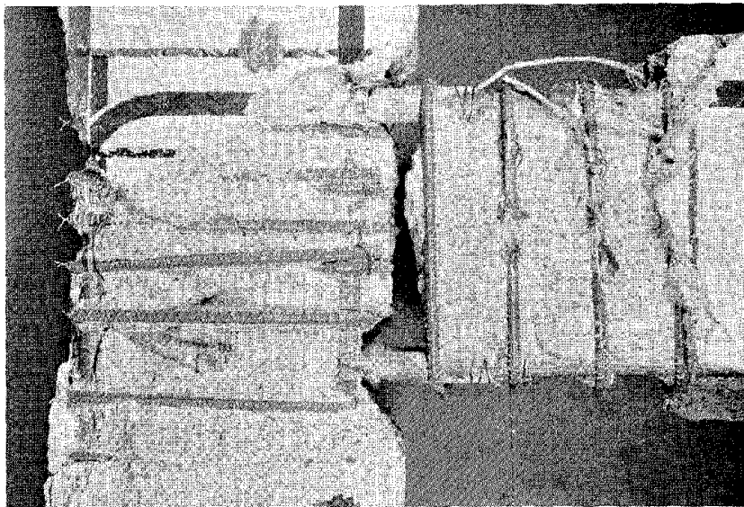
Fig. 3.25. Specimen 7 after Removal of Loose Concrete.
