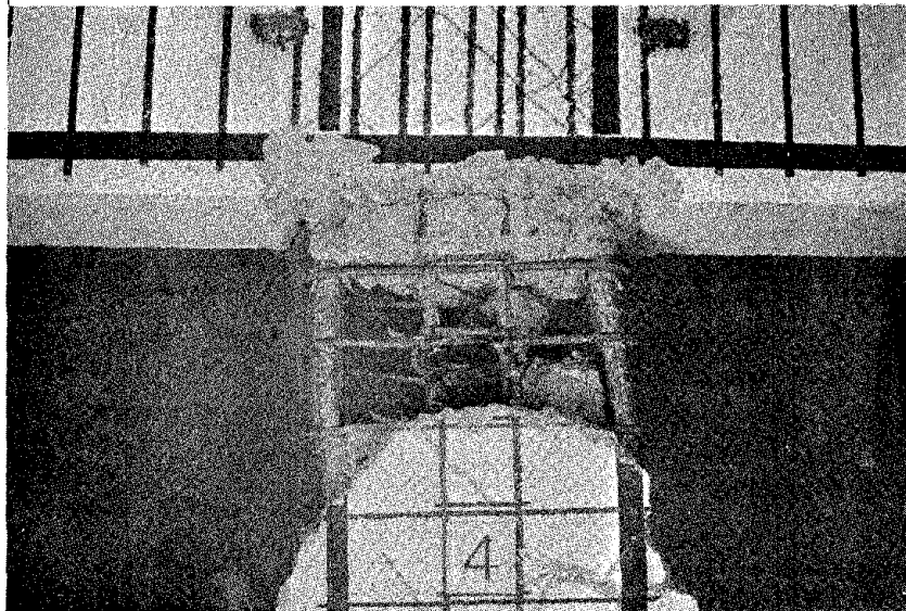
Fig. 3.17. Hinging Region of Specimen 4 after Removal of Loose Concrete.
