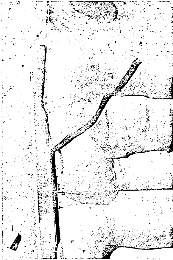
Fig. A-15. Diagonal Crack Across End Cell of Ceiling Number 2.
