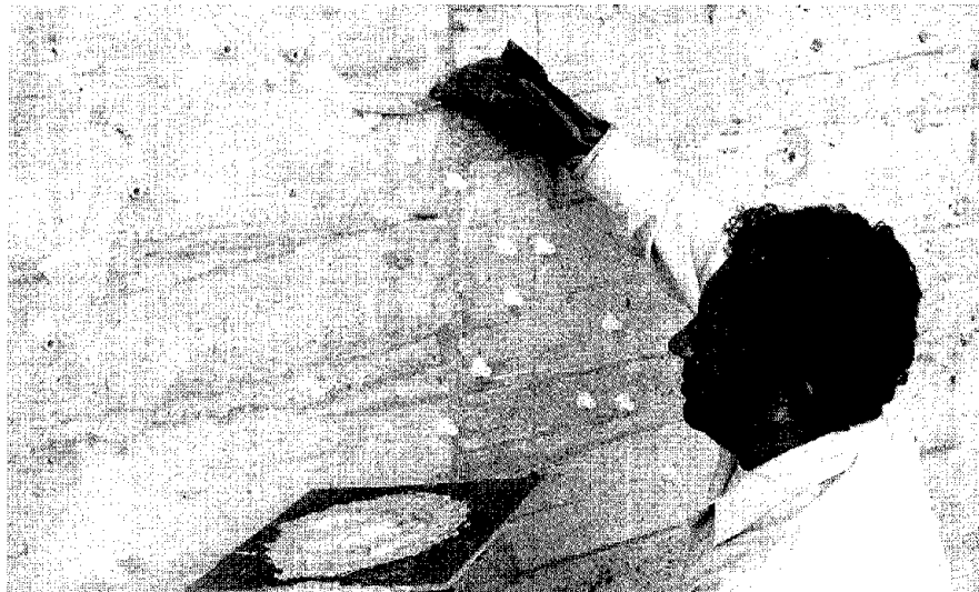
Figure 1 - Sealing cracks and installing plastic injection ports using thixotropic epoxy resin material.
