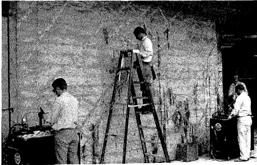
Figure 5 — Epoxy injection utilizing refrigerated pressure pot equipment.
