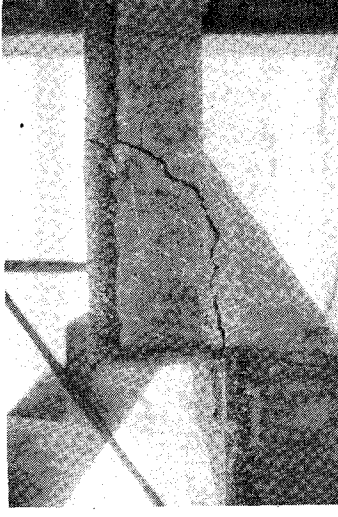
Fig. 26 Side of Stairwell Landing between Levels 0 and 1 after EW Tests
