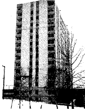
Fig. 2 Coupling beams of a 14-storey building that failed during the 1964 Alaska earthquake [4]
