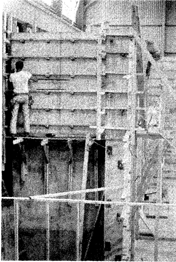
Fig. A16 Erecting second stage formwork for buttresses and walls
