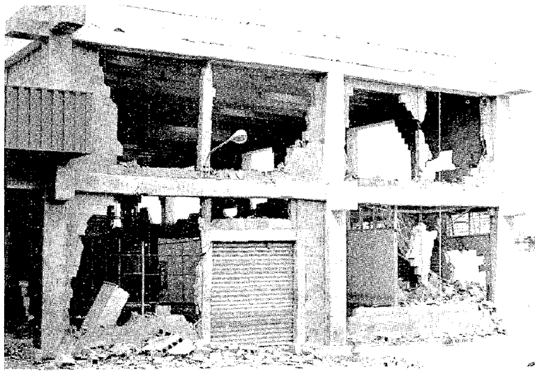
Fig. 10 "Frozen" deformed shape of frame
