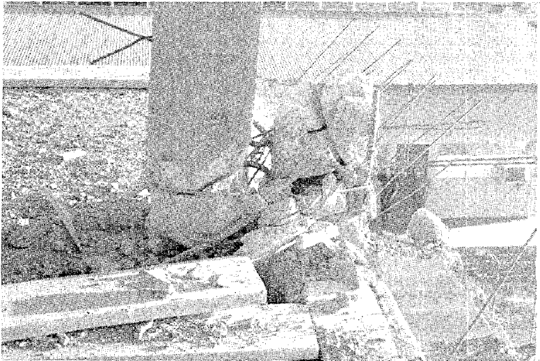
Fig. 3 Sheared off column
