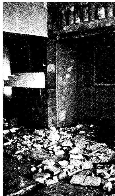
Figs. 4a, b. Spallation in Earthquake Damaged Structures
