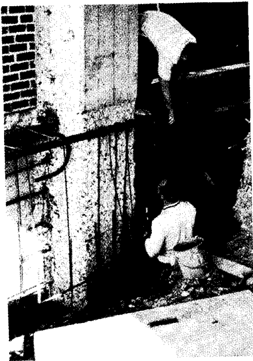
Figure 8 shows the construction work itself. Foundation work was the first phase following demolition. While foundation construction proceeded, holes and chases were drilled in slabs, columns, and brick walls throughout the building. (See Figure 9)
