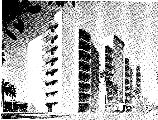
The 8-story San Diego Hilton which utilized 53 different sizes and shapes of concrete masonry units.
