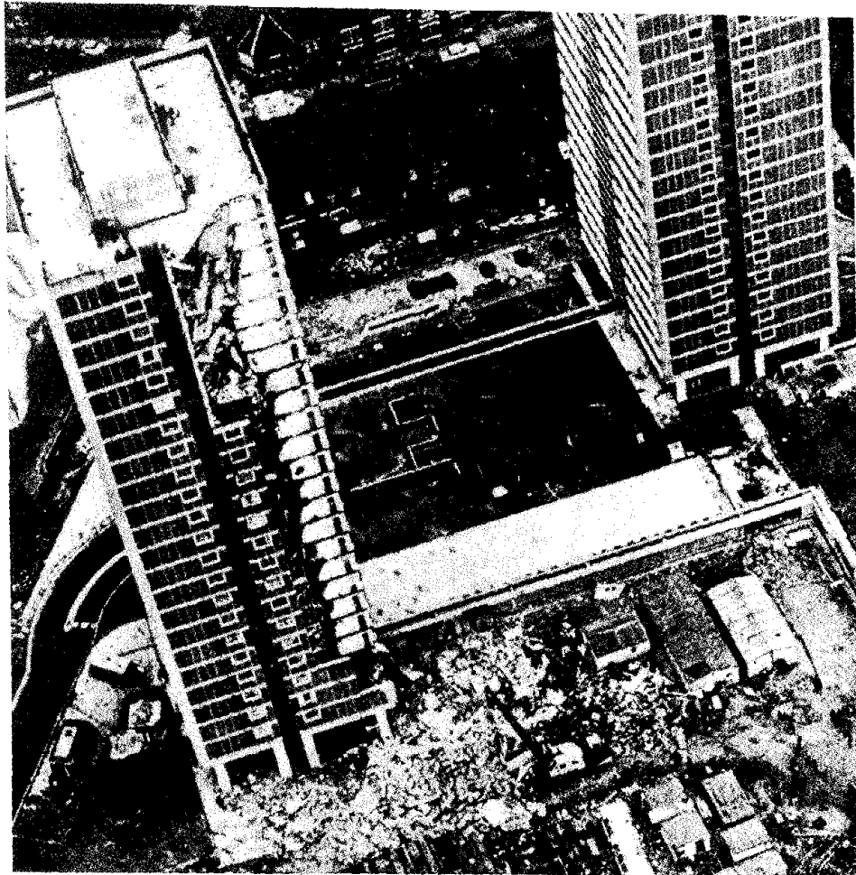
Figure 1. Ronan Point Apartment Building after the collapse, with a second identical building in the background. (Courtesy of London Express News and Feature Services)
