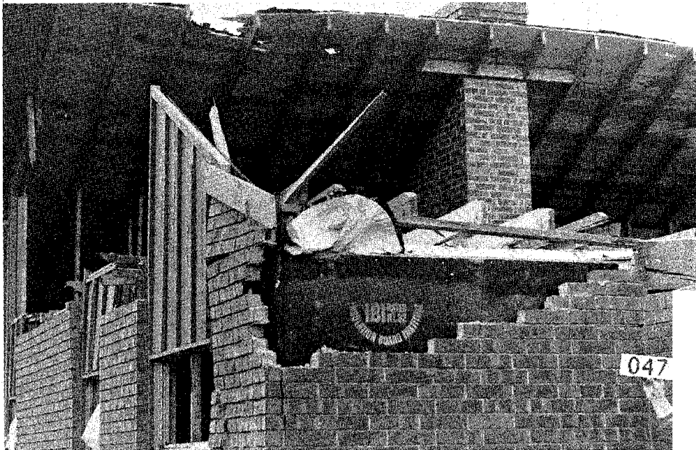
Figure 4 Non-Engineered Buildings Perform Poorly in Extreme Winds; Engine Principles Can Mitigate Wind Effects at Reasonable Cost.
