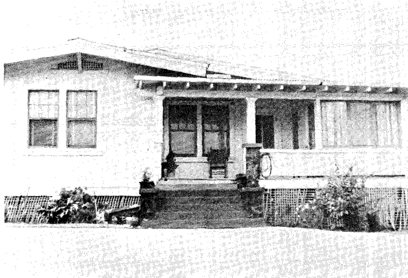
FIGURE 31 HOUSE SHIFTED ON FOUNDATION, NORTH HILO
