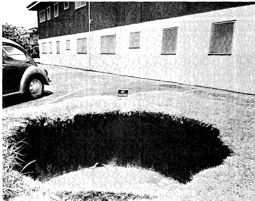
FIGURE 35 CESSPOOL FAILURE, VOLCANIC ASH
