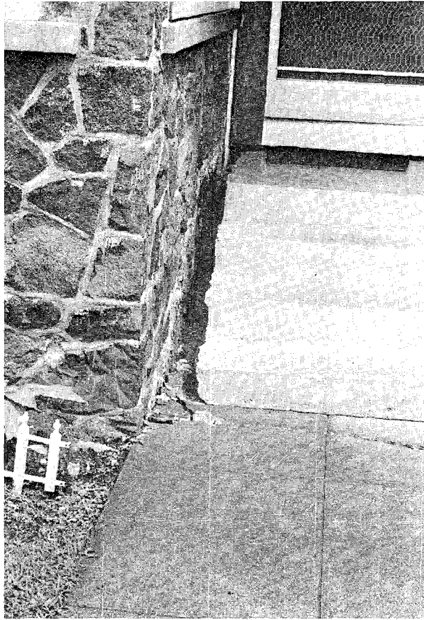
FIGURE 32 HOUSE SHIFTED ON FOUNDATION, NORTH HILO
