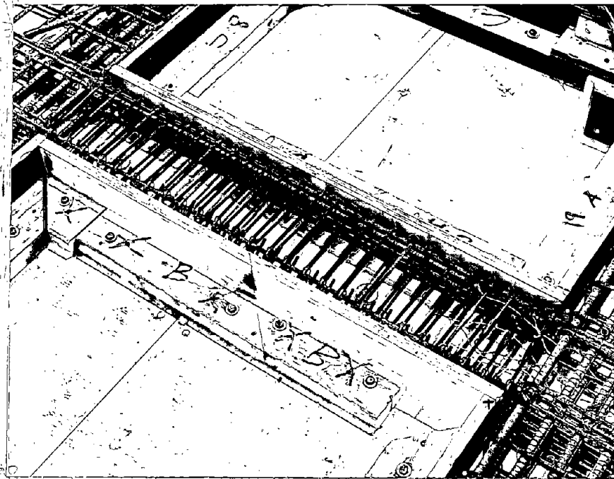
c) Reinforcement Cage
