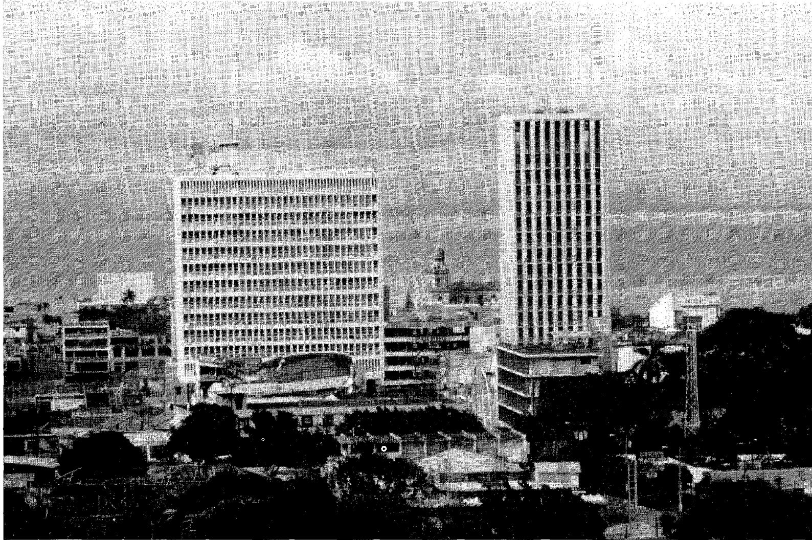
FIGURE II-20 Banco Central and Banco de America Buildings, Looking North.
