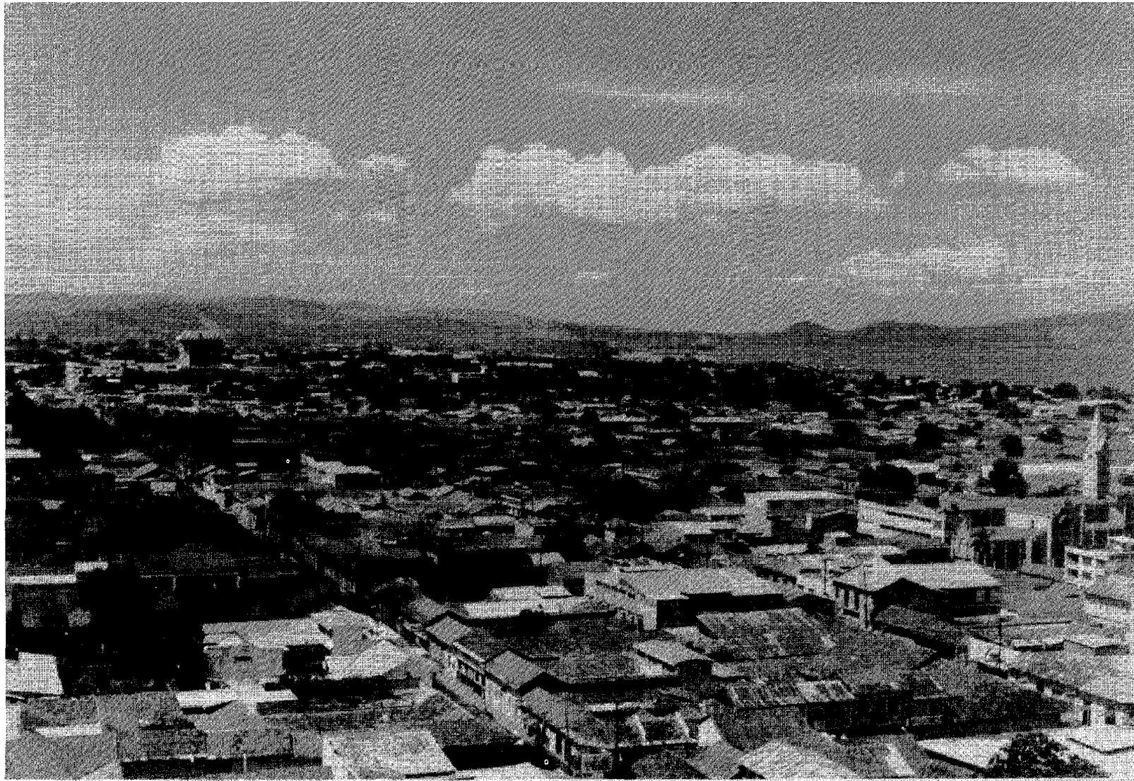
FIGURE II-34 View Before Earthquake, Looking W-N-W from Banco de America Building.
