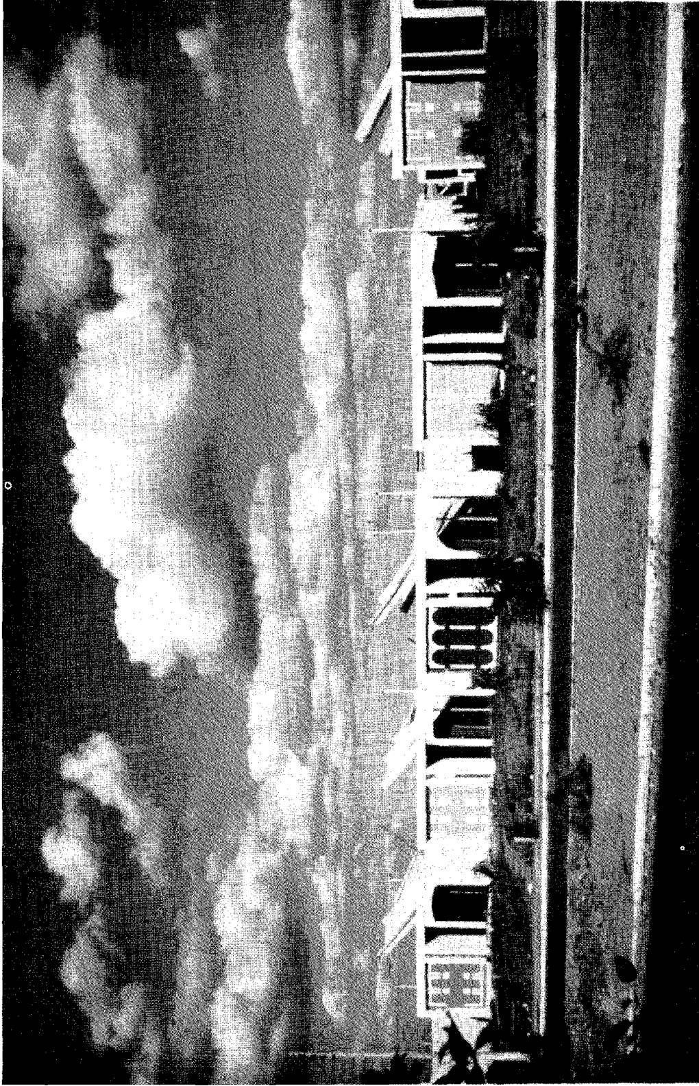
FIGURE II-11 Precast Concrete Roof.
