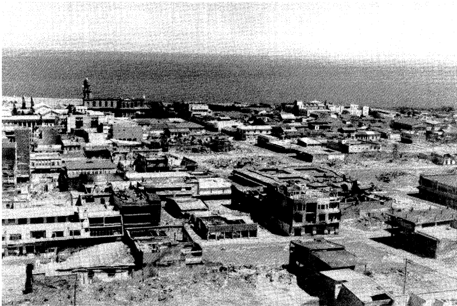
FIGURE II-25 View After Earthquake, Looking North from Banco de America Building.
