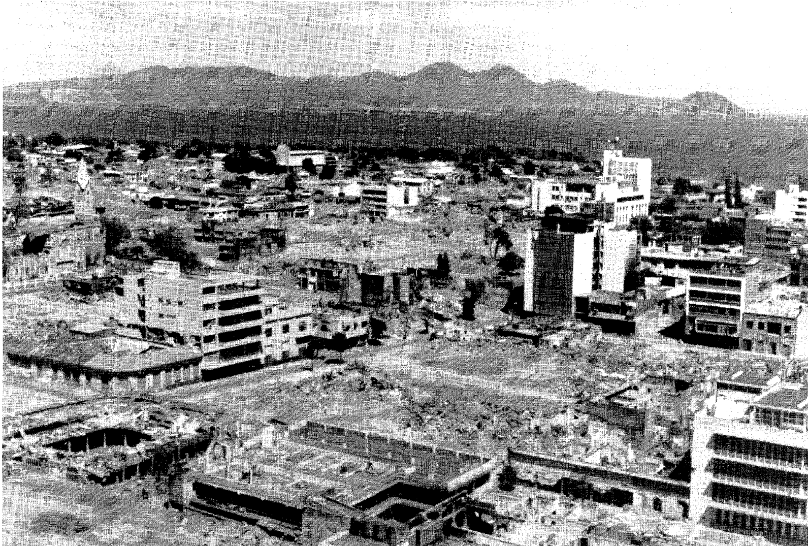
FIGURE II-37 View After Earthquake, Looking Northwest from Banco de America Building.
