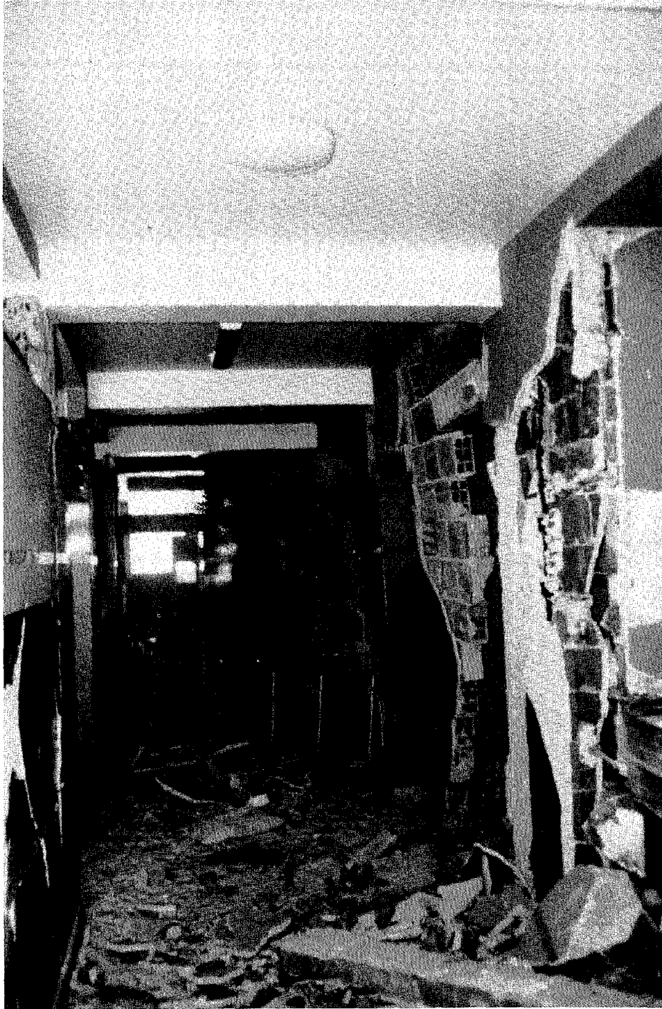
FIGURE II-53 Social Security Institute Hospital, Corridor.
