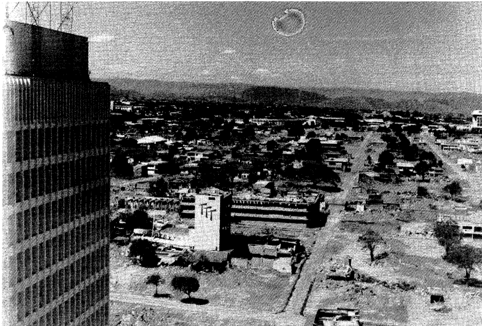
FIGURE II-33 View After Earthquake, Looking West from Banco de America Building.
