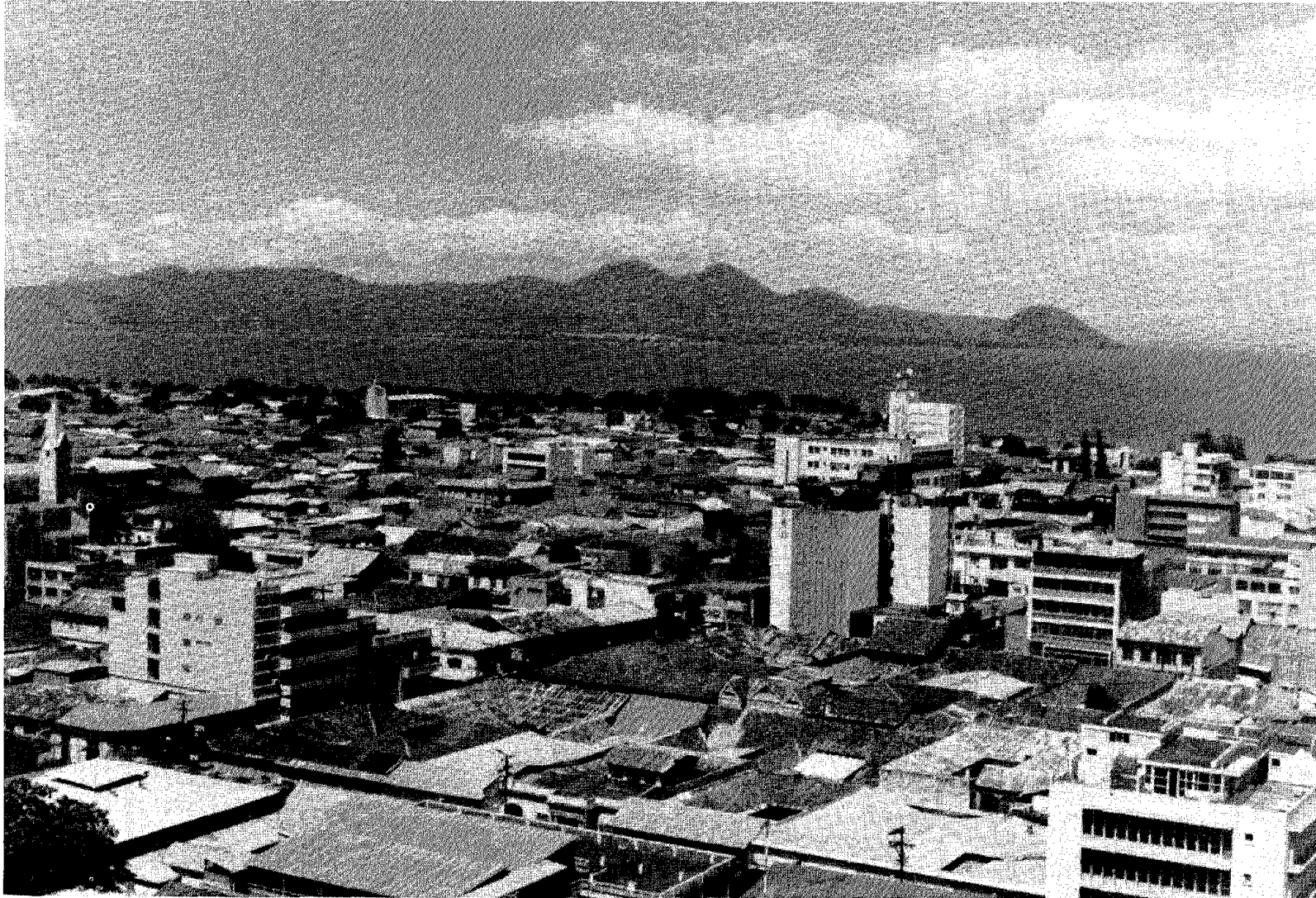
FIGURE II-36 View Before Earthquake, Looking Northwest from Banco de America Building.
