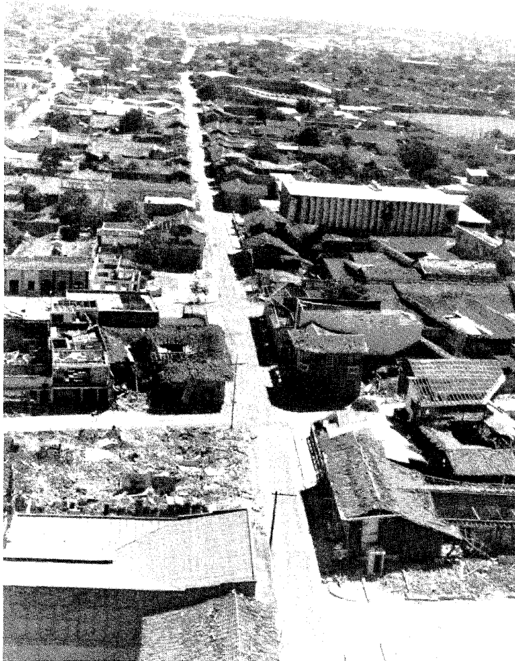
FIGURE II-29 View After Earthquake, Looking East from Banco de America Building.
