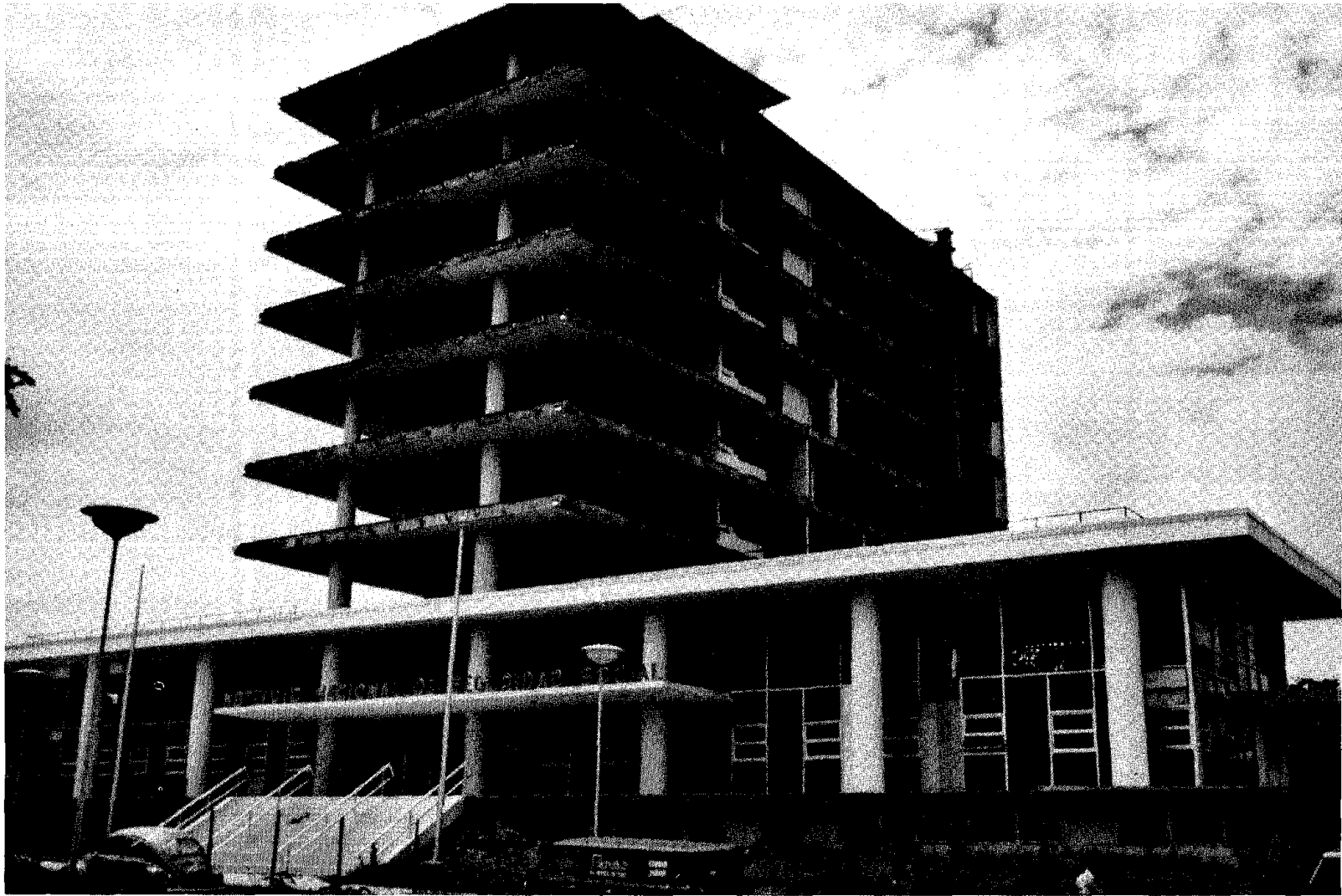
FIGURE II-19 . Social Security Institute Building After Removal of Non-structural Elements.
