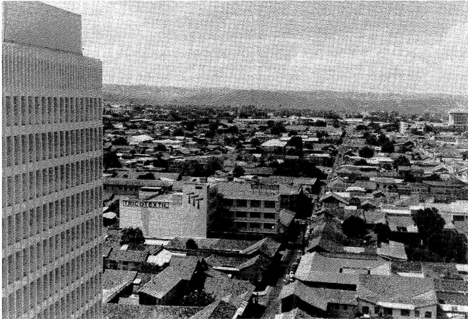
FIGURE II-32 View Before Earthquake, Looking West from Banco de America Building.
