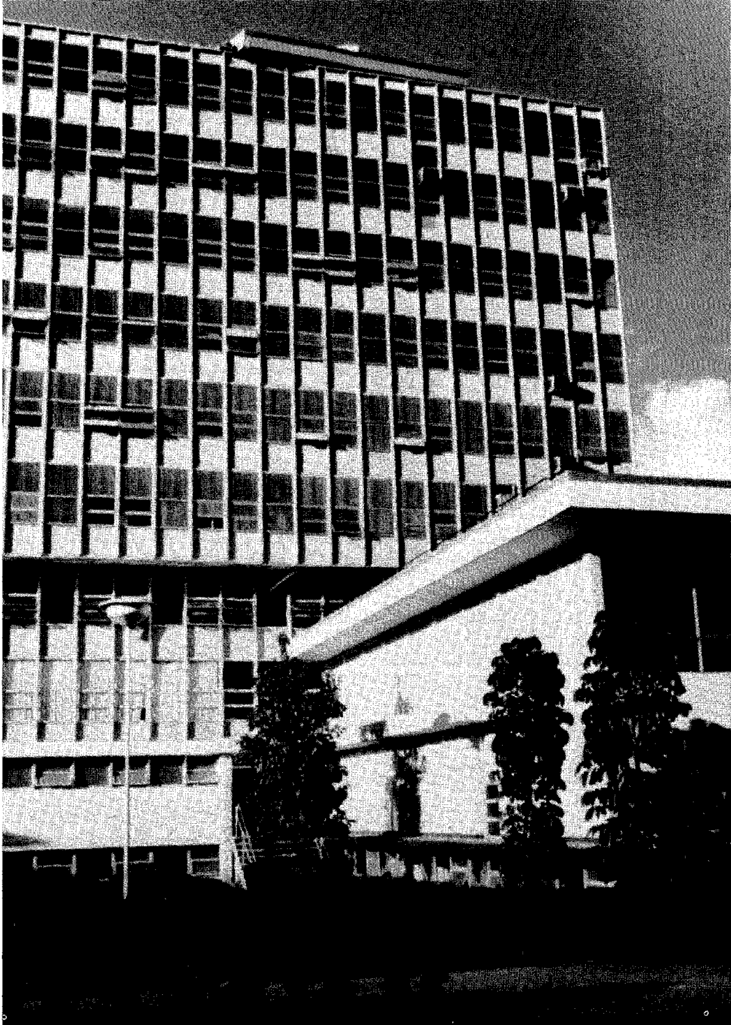
FIGURE II-18 Social Security Institute Building After Earthquake.
