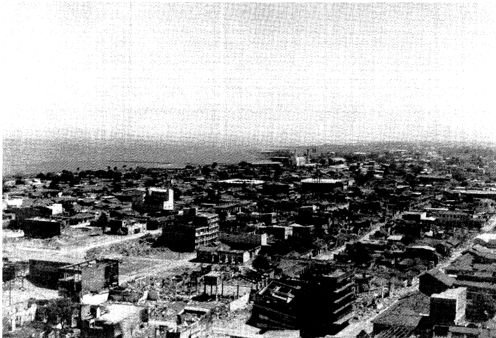
FIGURE II-27 View After Earthquake, Looking N-N-E from Banco de America Building.
