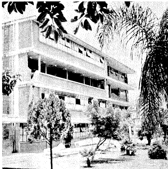
Figure 21 Damage to classroom block (Building B), Technologico of Orizaba.
