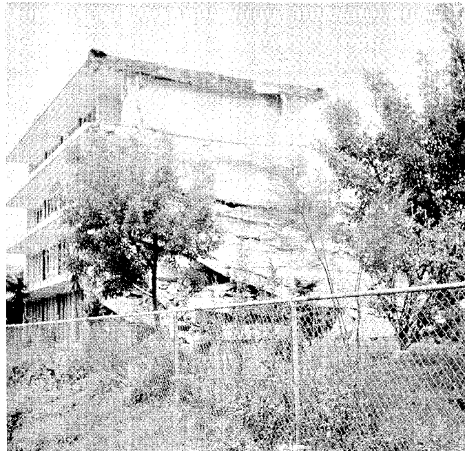
Figure 16 Collapse of classroom block (Building A), Technologico of Orizaba.
