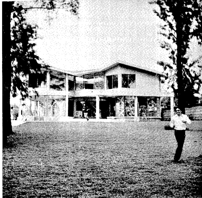
Figure 44 View of a modern house under construction in Córdoba.
