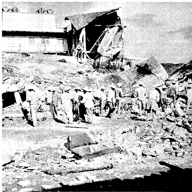
Figure 13 Collapse of "Packard" apartment building, Orizaba
