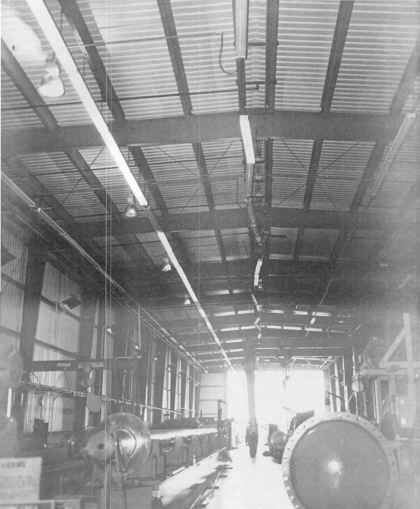
Fig. 3.6 Dislodged and missing fluorescent lighting fixtures from overhead electrical raceways, in Flight Physics Building, Delco Electronics.
