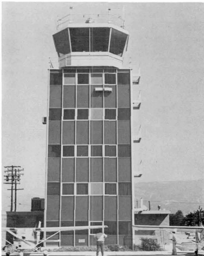
Fig. 7.60 Air traffic control tower, Santa Barbara Municipal Airport (view from south).
