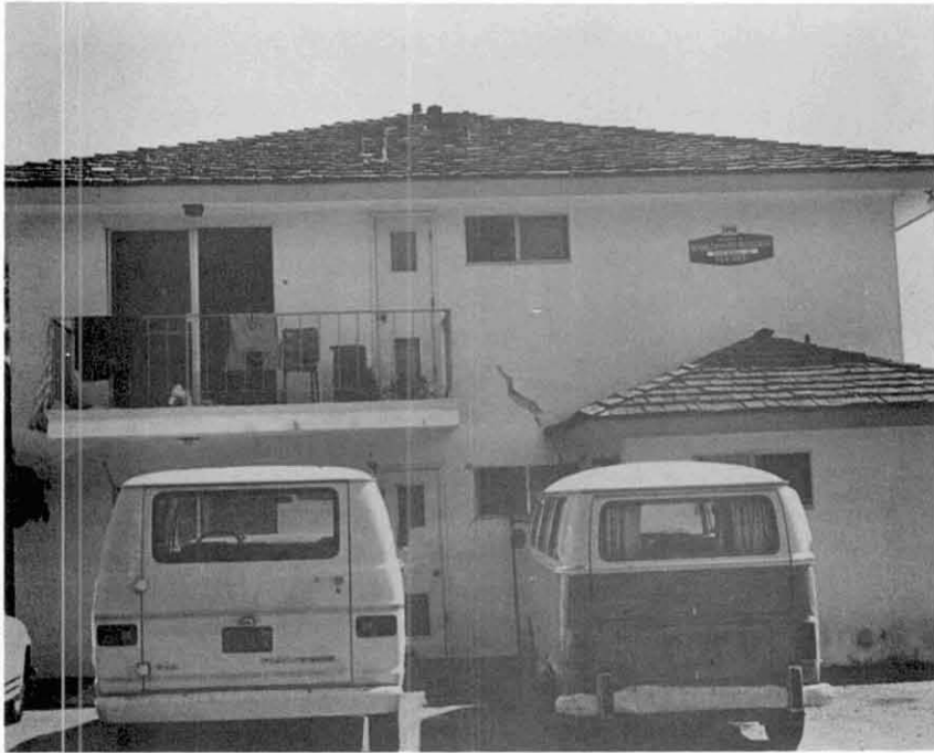
Fig. 7.50 Cracks in exterior plaster walls of two story residential building in Isla Vista.
