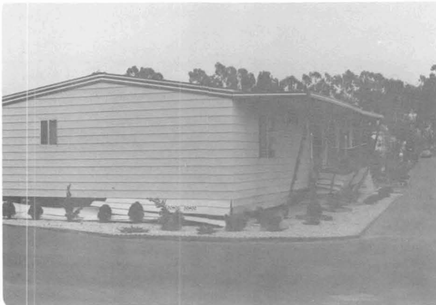
Fig. 7.55 View of damaged porch, awning, and skirt of mobile home which fell from its foundation at Santa Barbara West Mobile Home Park.
