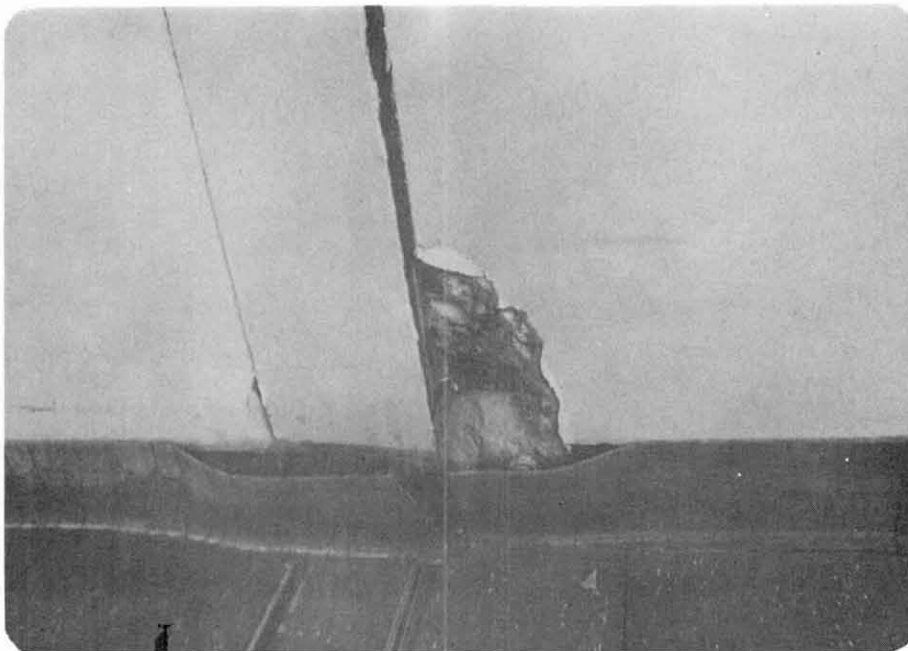
Fig. 11.4 Close up of the damage in the corner at the right in Fig. 11.3.
