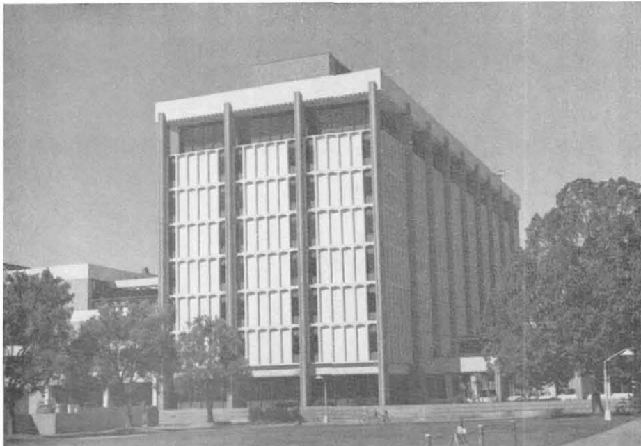
Fig. 7.38 Eight story Library III Building, UCSB. This building also sustained cracks in shear walls in lower stories.
