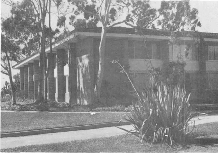
Fig. 7.18 Anacapa Residence Hall, UCSB.
