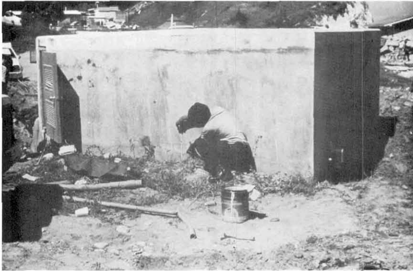
Fig. 9.5 Settlement of soil near pumping facility at sand spit, UCSB. Note previous soil line on concrete.
