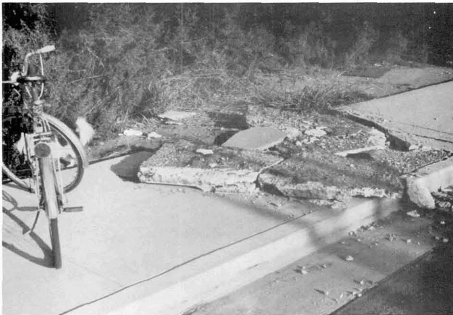
Fig. 9.8 View of sidewalk in Fig. 9.7 from opposite direction.
