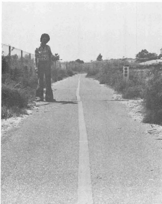
Fig. 9.1 Extension fracture in the bicycle path north-east of UCSB. Note misalignment of centerline. Building at upper right is Biological Sciences II, UCSB. Cracks runs in a northwesterly direction.
