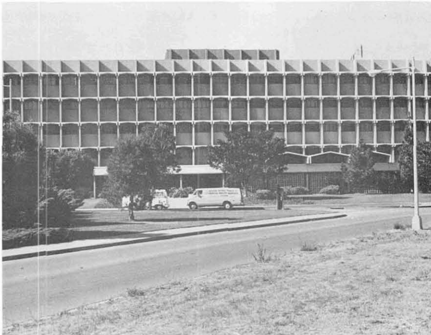
Fig. 7.26 Engineering Building UCSB. (View from south).
