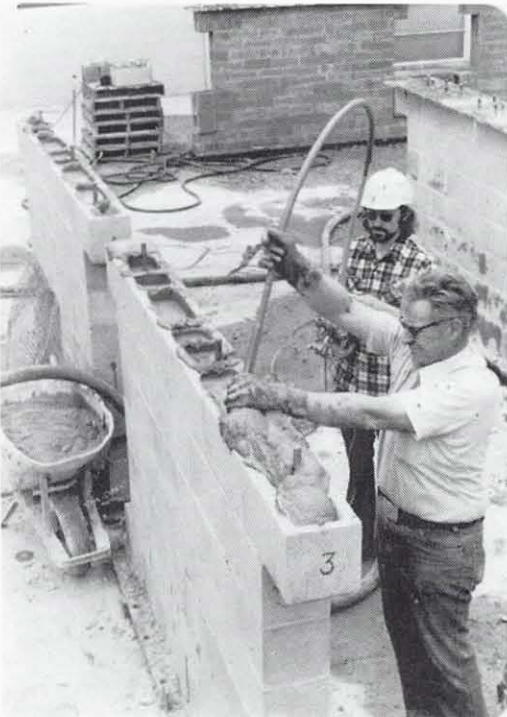
FIG. 2.2 CONSTRUCTION OF TEST SPECIMENS
