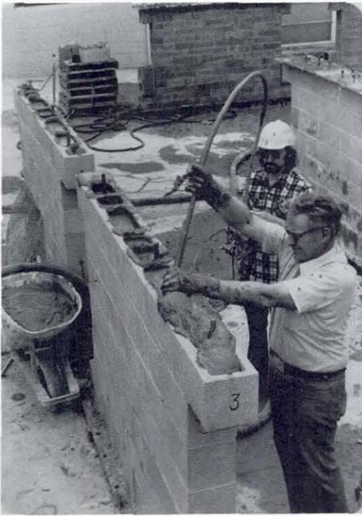
FIG. 2.2 CONSTRUCTION OF TEST SPECIMENS
