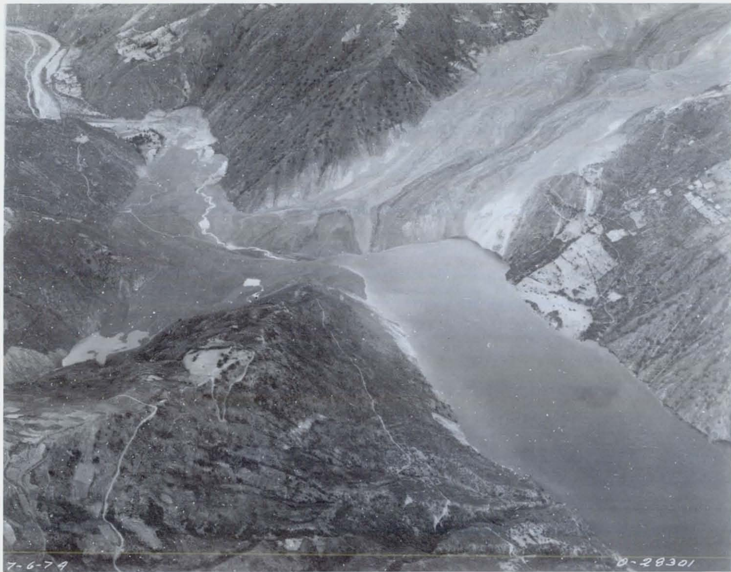
FIGURE 32. Oblique air photo taken June 6, 1974, showing water as it begins slowly to flow over the debris dam. (Defensa Civil Photograph)
