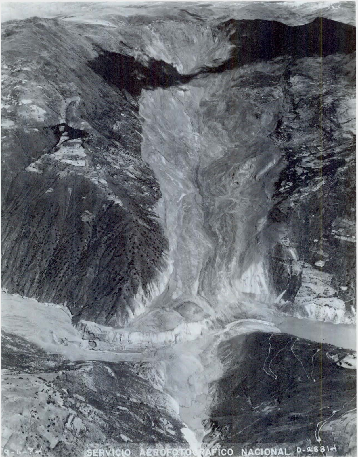
FIGURE 15. Oblique air photo taken June 9, 1974, the day following the major flooding from overtopping. (Servicio Aerofotografico Nacional, Peru)
