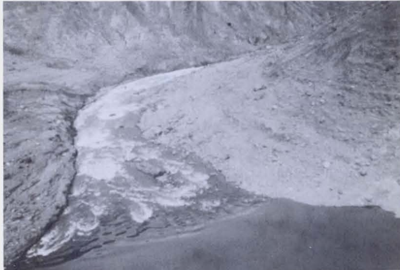
(b) After overtopping, showing nature of material exposed in the erosion slopes.
