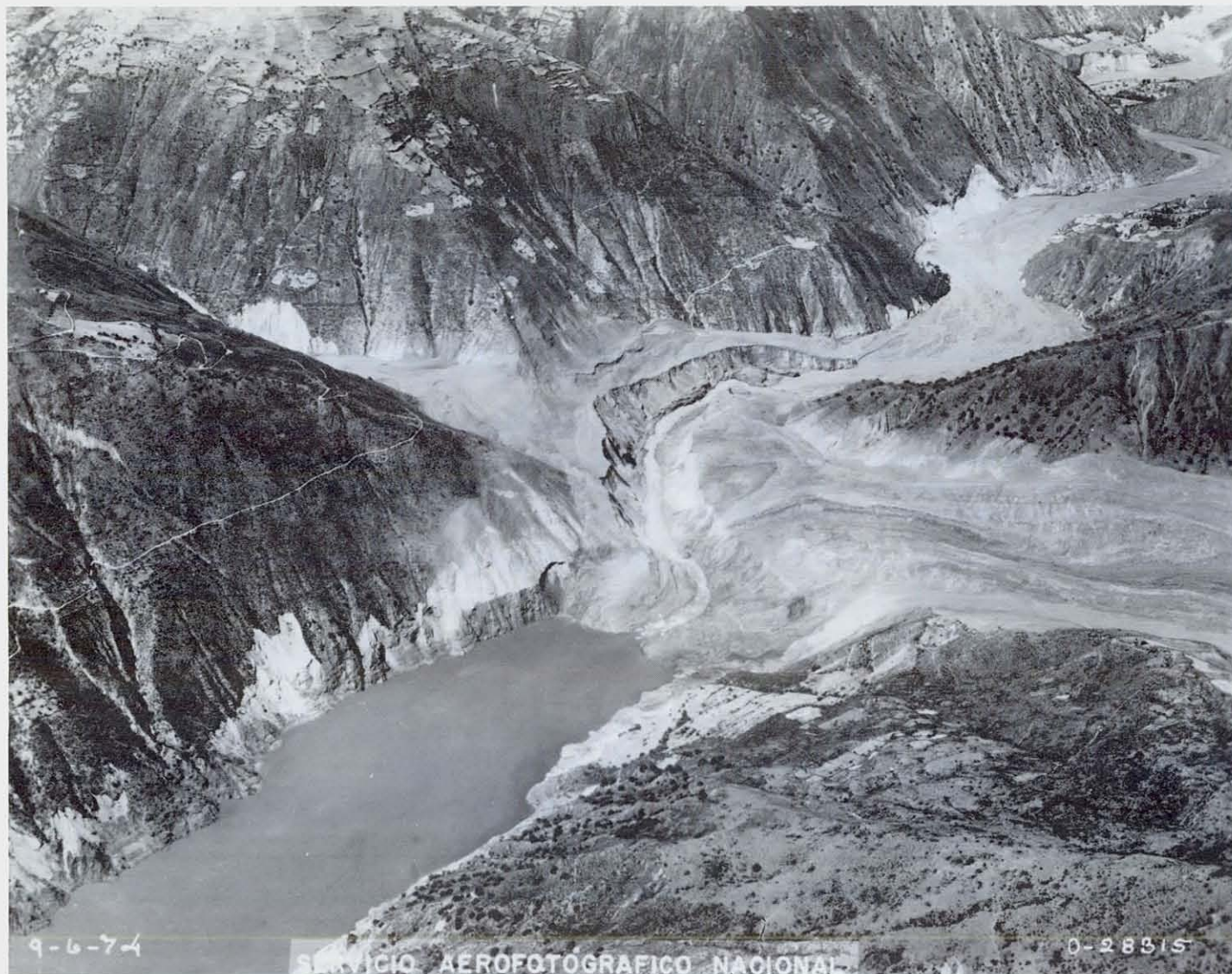
FIGURE 34. Oblique air photo looking downstream across the debris dam, taken June 9, 1974, the day after the flood. (Defensa Civil Photograph)
