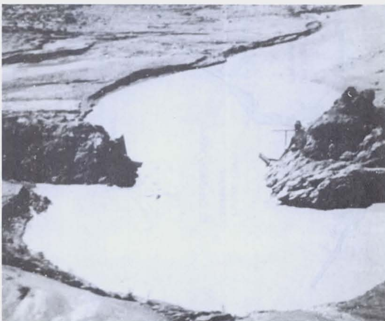
FIGURE 39. Mayoc bridge across the Mantaro River after destruction by the high flood water. (Photograph courtesy of Gen. Rodolfo Acevedo del Campo)
