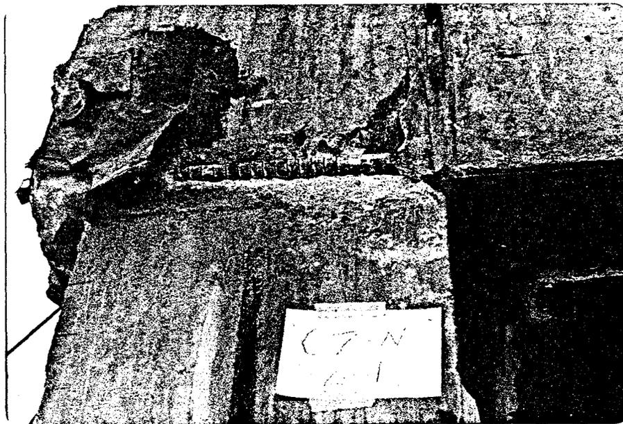
Fig. 74 Exposed Reinforcing Bar,
