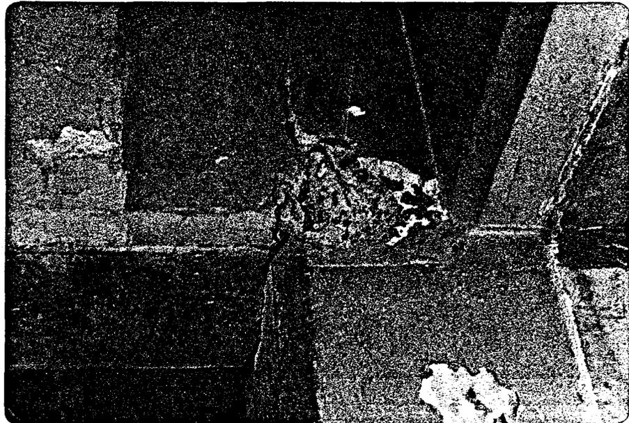
Fig. 71 Beam-Column Joint Damage,
