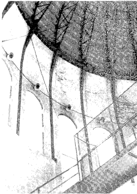
FIGURE 17 EXISTING TRUSSES AT UPPER DOME
