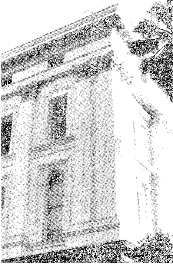
FIGURE 3 CAST IRON WINDOW FRAMES AND ROOF CORNICES
