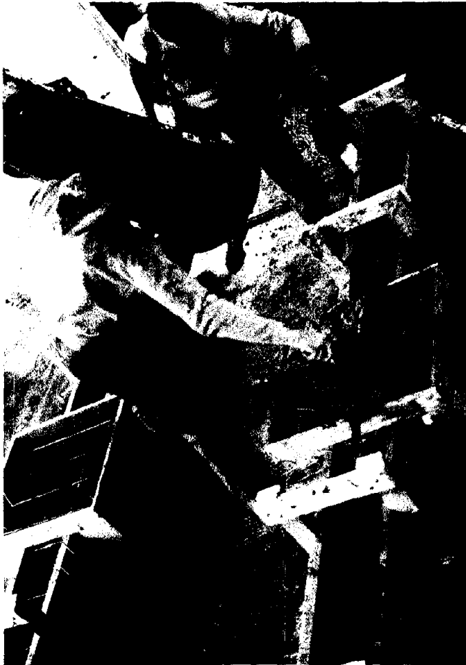
Figure 2.6 Casting column specimens.
