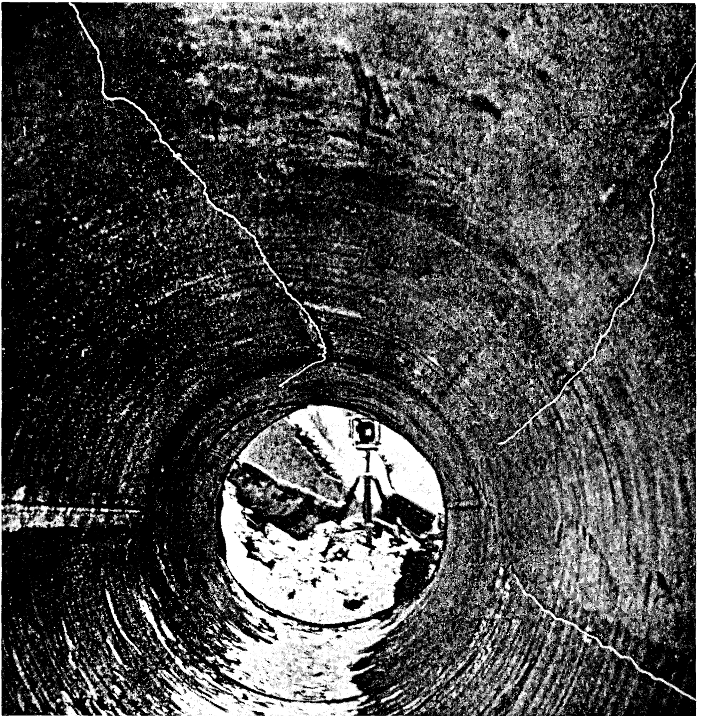
Figure 2 Brittle Crack Propagation in a Concrete Pipe.
