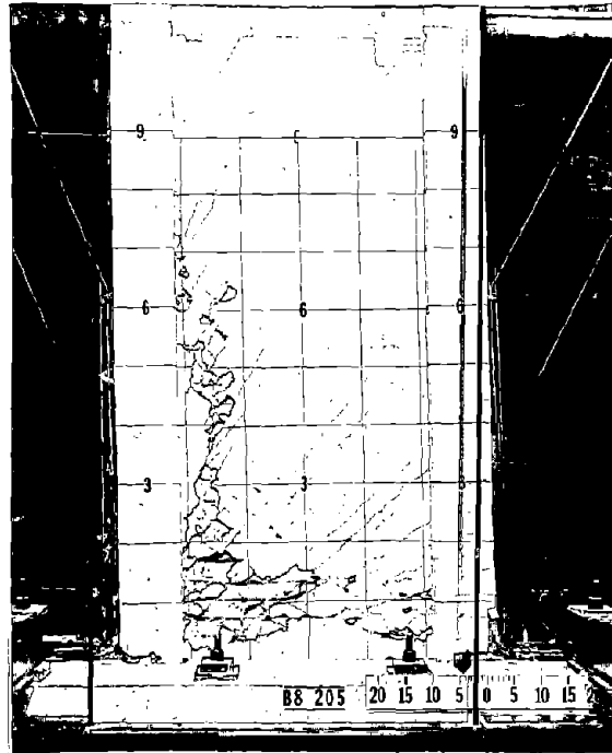
Fig. B-67 - Specimen B8 After Web Crushing
