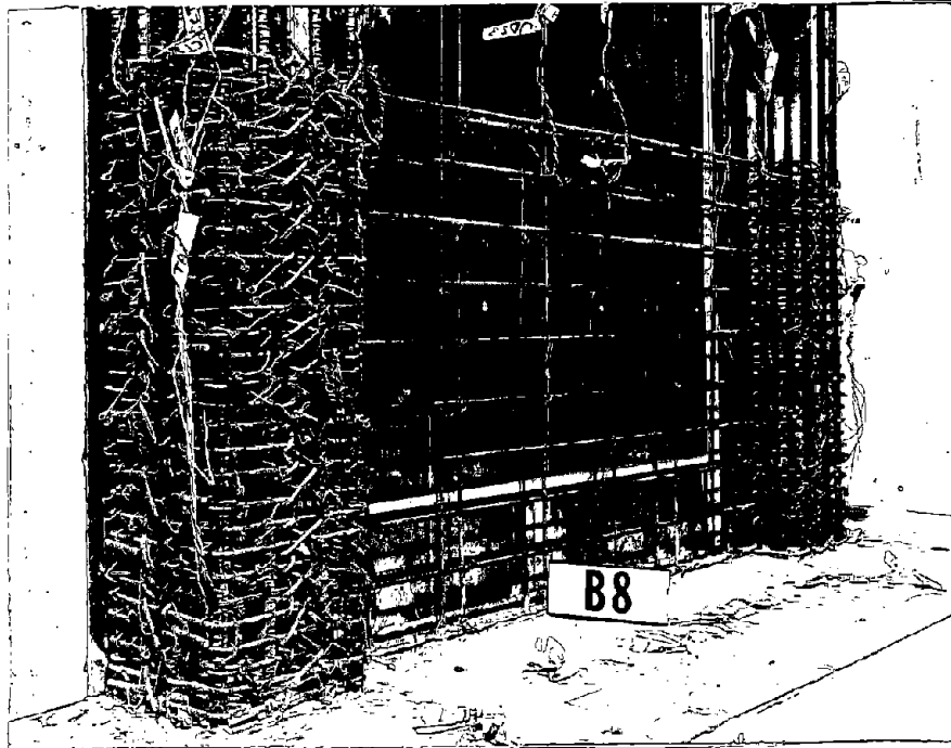
Fig. A-12 Reinforcing for Specimen B8
