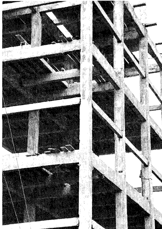
FIGURE 3.47 Occupied brick apartment house in Chengtu. Note the brick columns.
