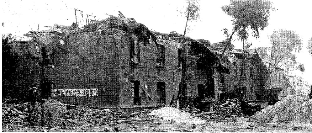
FIGURE 4.25 Collapsed top story of the three-story Kailuan coal mine dormitory, Tangshan.
