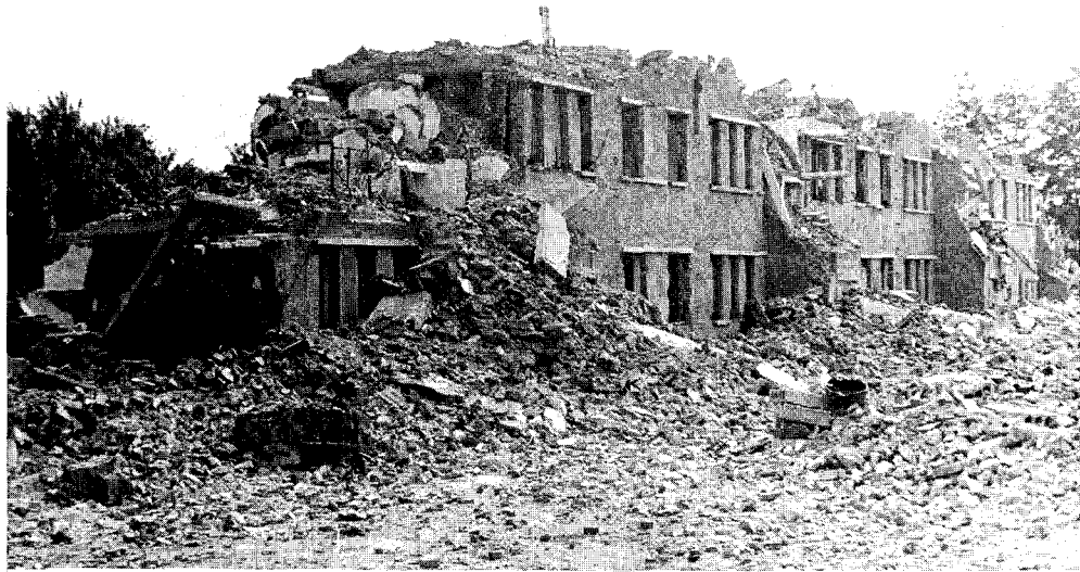
FIGURE 4.26 Collapsed four-story Tangshan Mine-Metal Institute residence building.
