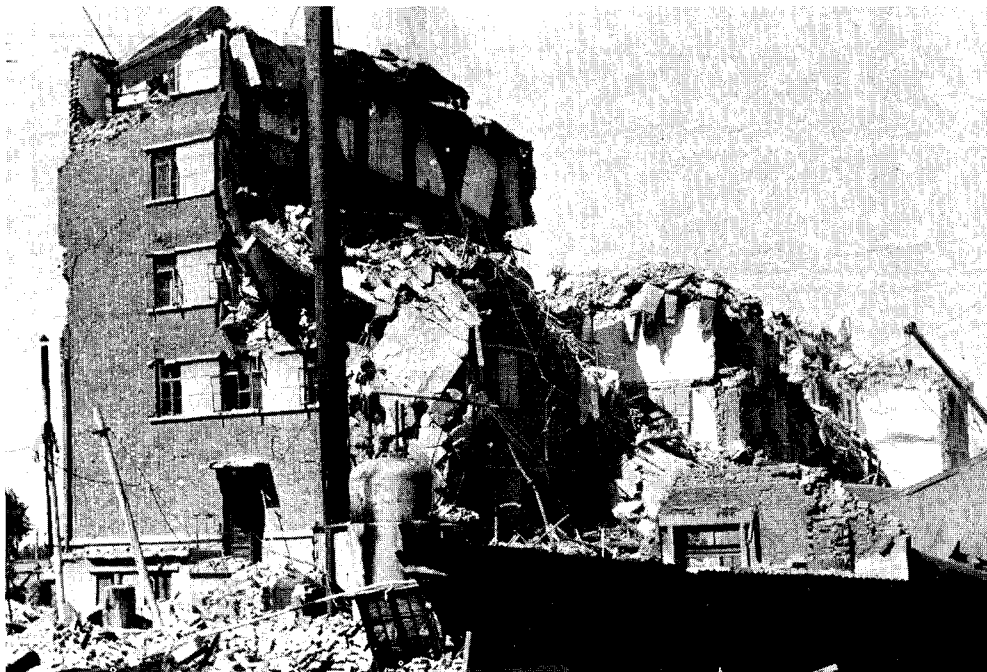
FIGURE 4.28 Collapse of Kailuan coal mine reception building, Tangshan.
