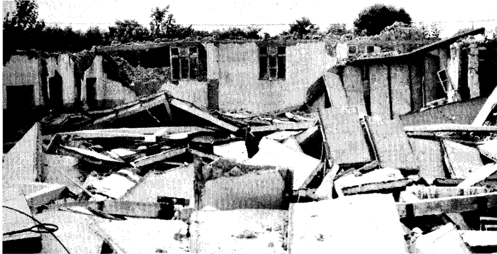
FIGURE 4.33 Collapsed workers' cafeteria building of the Chinkechuang coal mine.
