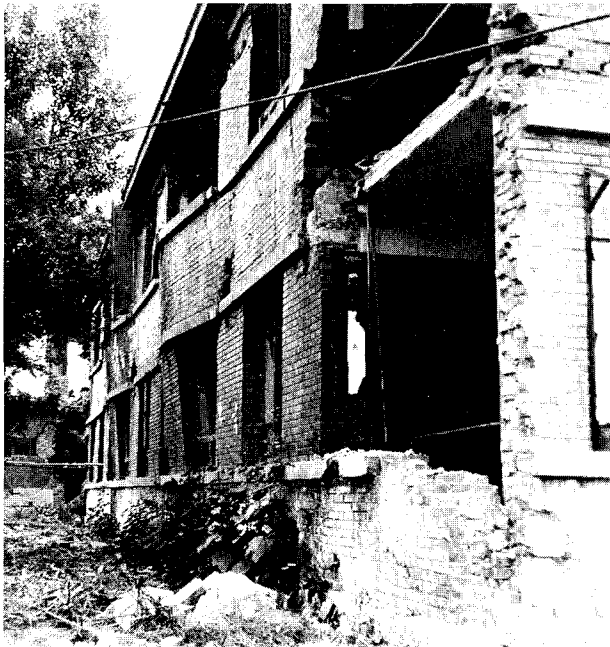
FIGURE 4.36 Badly distorted brick building on the verge of collapse. The second floor appears to be of precast concrete slabs supported on precast concrete beams, which, in turn, are supported on unreinforced brick piers.
