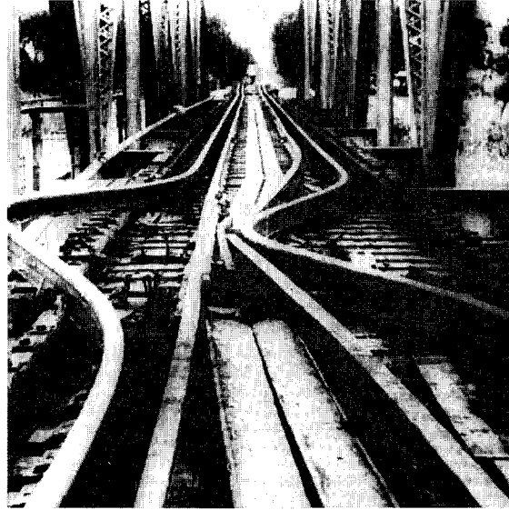
FIGURE 4.58 Buckled steel rails on railway bridge on Peking-Shanhaikuan line.
