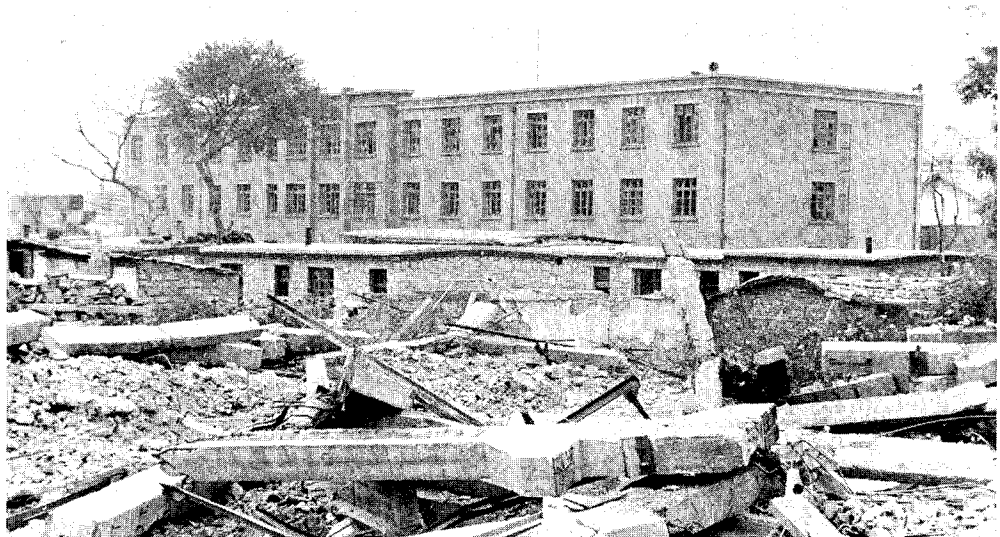
FIGURE 4.52 Tangshan light-machine plant official building. This structure, which was located in district 13 of Figure 4.21, was only slightly damaged. The remains of a collapsed building can be seen in the foreground.
