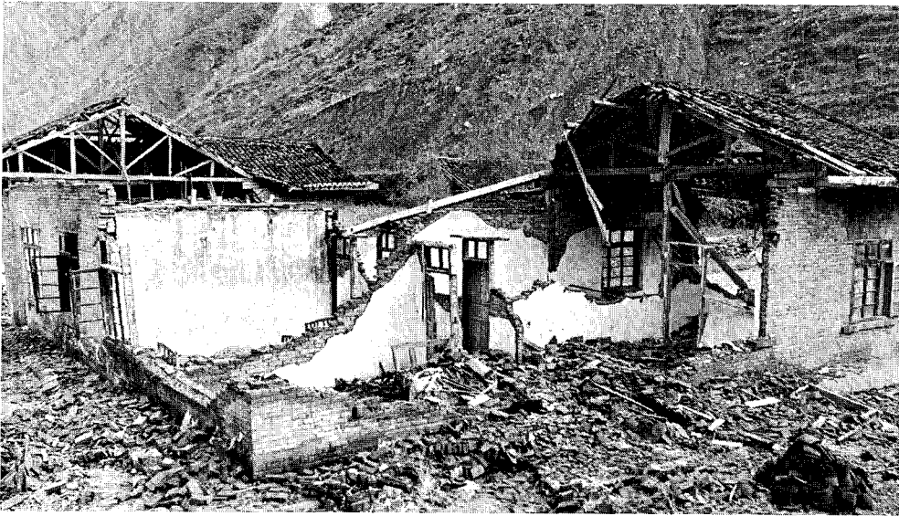
FIGURE 5.12 A second less common and less resistant type of construction consists of brick columns and walls, with wooden roof trusses.
