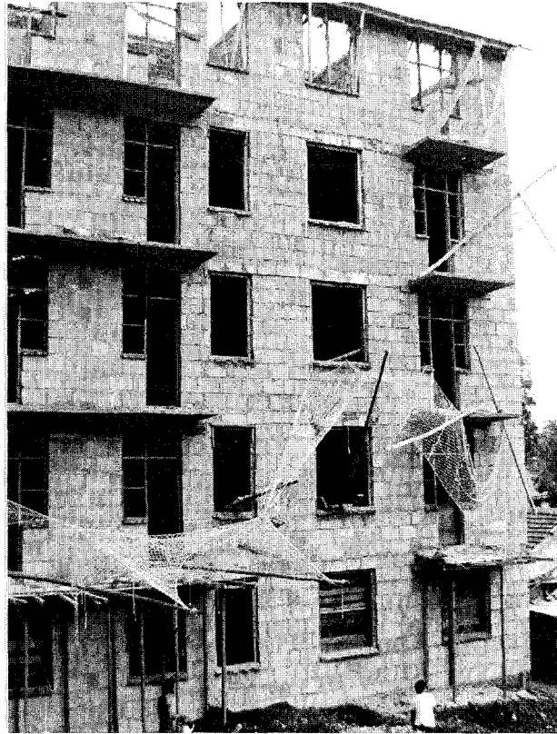
FIGURE 3.28 Exterior view of six-story apartment building in Harbin. Masonry blocks are cast of fly ash concrete.
