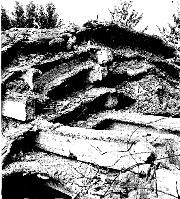
FIGURE 4.27 Collapsed five-story physics-chemistry building of the Tangshan Mine-Metal Institute.
