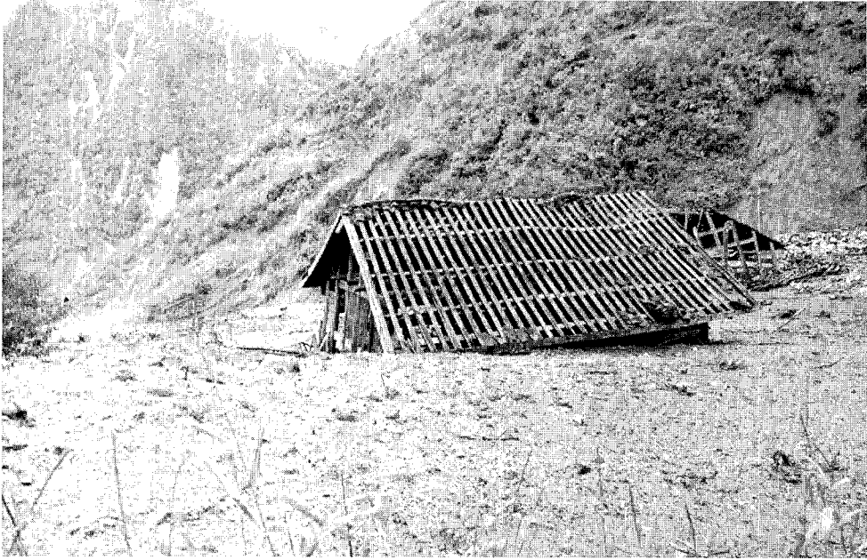
FIGURE 5.18 Mud flow damage from the SP earthquakes.
