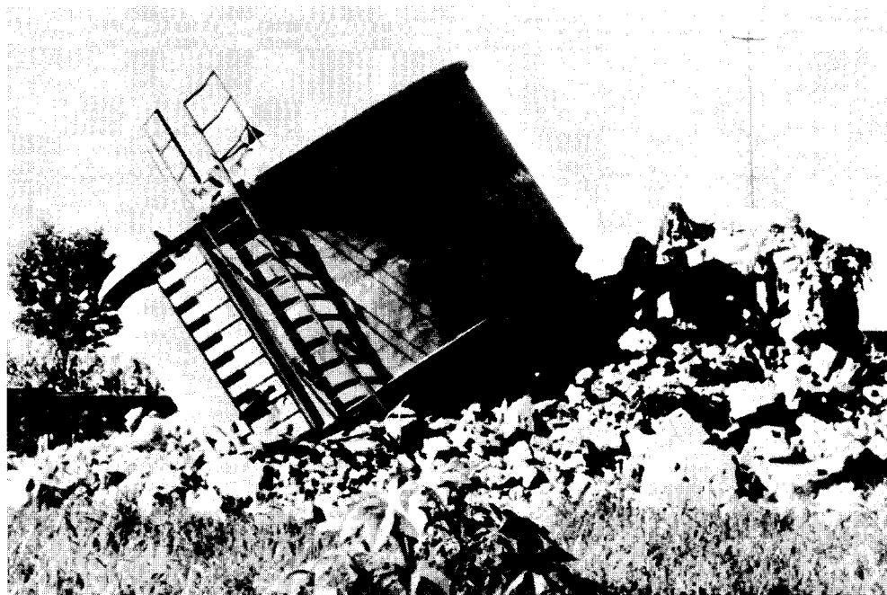
FIGURE 4.38 Collapsed elevated storage tank that had been supported on a brick cylindrical tower, Tangshan scale factory.
