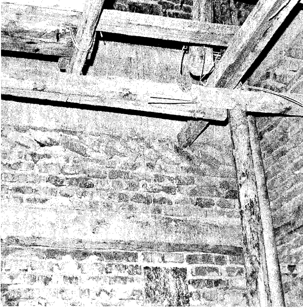
FIGURE 3.22 Interior of elevator shaft of Peking Duck Restaurant showing brick filler walls. Note "leaning soldier" bricks at top, a method of filling space, not a module of brick dimensions.
