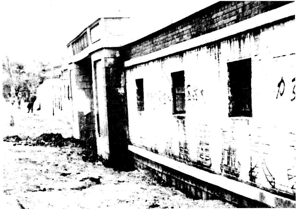
FIGURE 4.47 Uneven settlement of office building, Fanken Chuang Commune, Luan-nan Hsien.
