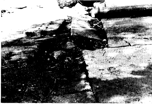
FIGURE 4.18 Surface breaks and compressed pavement over drainage trench in Tangshan.
