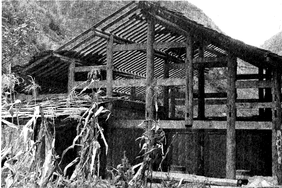
FIGURE 5.11 Wood framing is the most common residential construction in the mountainous epicentral area of the Sungpan-Pingwu (SP) earthquakes.
