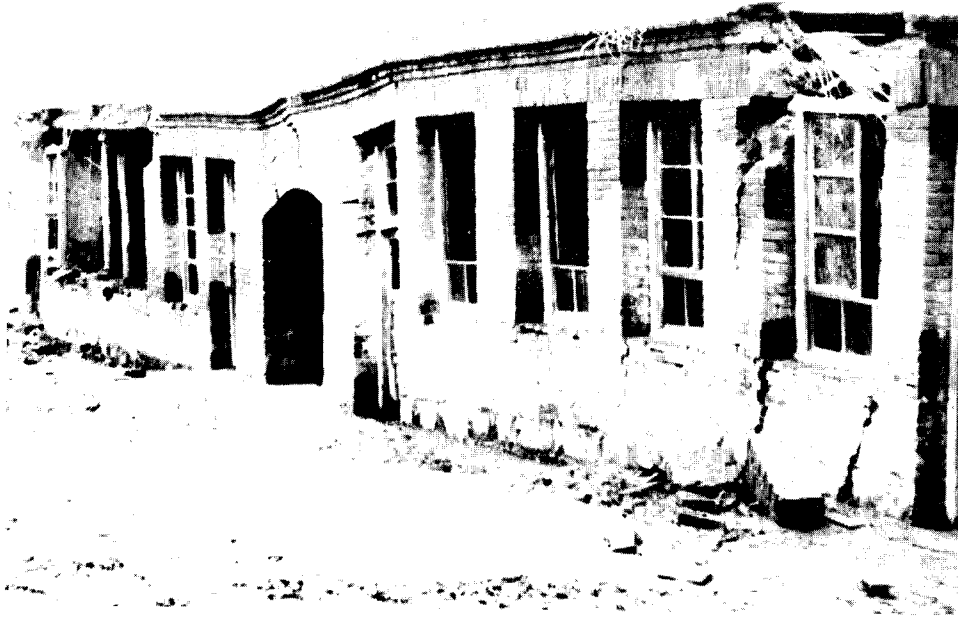
FIGURE 4.61 Structure damaged by unequal ground settlement.
