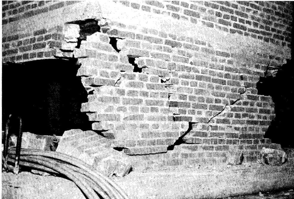
FIGURE 3.13 Close-up view of the lower floor of the end wall of the model shown in the previous figure. The end wall has failed in shear, with fracture occurring mainly through the bricks, rather than the grout.
