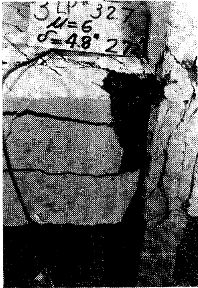
Fig. 4.30 Rupture of Tension Reinforcement at Top of First-Floor Columns, Specimen 4R
