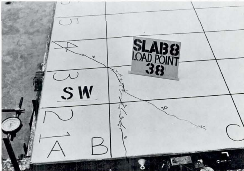
(b) DIAGONAL CRACKING TYPICAL AT CORNERS.
