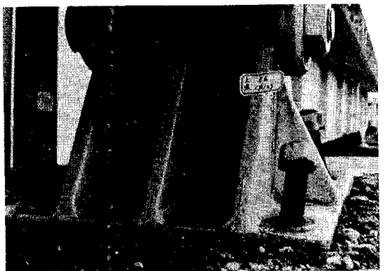
Fig. 25 Pull-out of Anchor Bolts and Settlement of the Shoe at the Upstream Fixed Bearing on Pier 6, Kin-noh Bridge. (After June 12, 1978)
