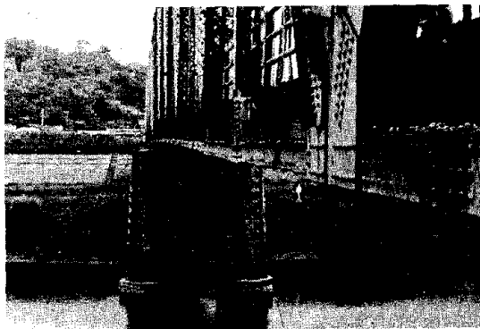
Fig.30 Drooping of the Lower Truss Chord, Maiya Bridge
