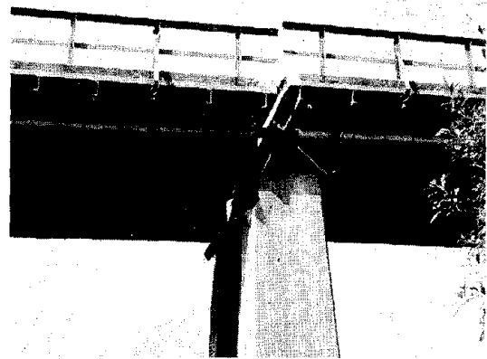
Fig.33 A Girder almost Dislodging from a Pier Cap, Kimazuka Bridge
