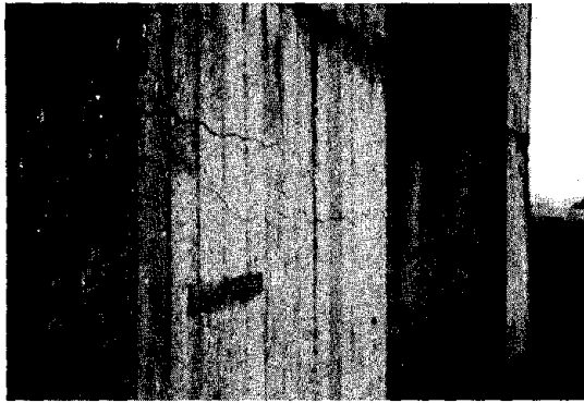
Fig.28 Cracks of Sides of Columns of Pier 8, Kin-noh Bridge (After June 12, 1978)
