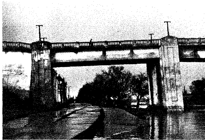
DISTORTION DUE TO SOIL PRESSURE ON ABUTMENT
