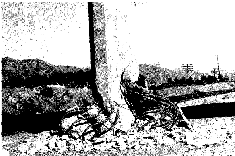
Figure 1 - San Fernando Column Damage - Br. No. 53-1990R
