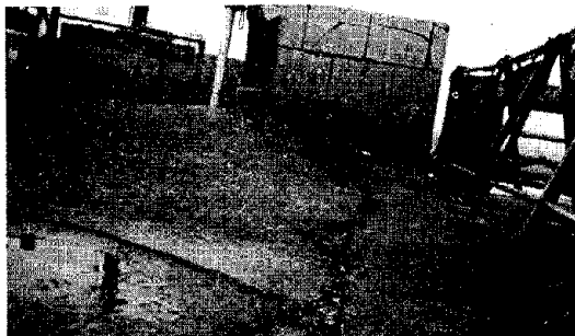
Fig. 24 Heaving of Asphalt Pavement at the Backfill of the Right Abutment, Kin-noh Bridge (After June 12, 1978)
