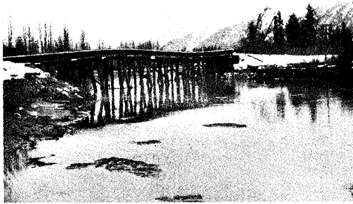
FIG. 3 BUCKLING OF BRIDGE DECK DUE TO INWARD MOVEMENT OF ABUTMENTS. (ALASKA EARTHQUAKE, 1964).
