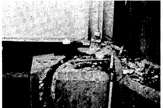
Fig. 23 Failure of the Right-Bank Abutment Girder Moved Toward Abutment Kin-noh Bridge by 10 cm, Temporary Support is seen. (After June 12, 1978)
