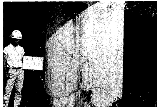
Fig.35 Cracks at Pier 1, Yuriage Bridge
