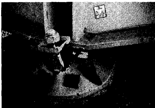
Fig. 18 Failure of Side Block of Oval Line Bearing on Pier 11, Kin-noh Bridge (Just after February 20, 1978)
