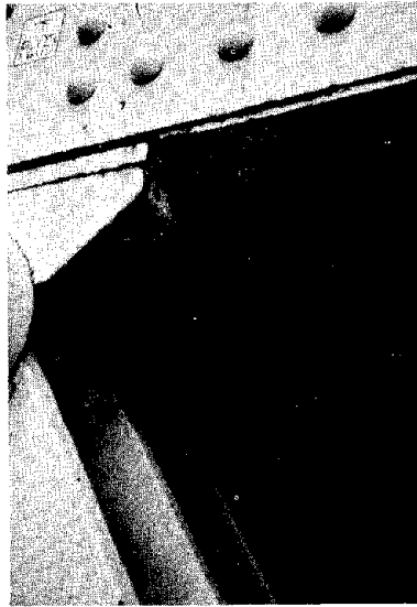
Fig. 20 Failure of Set Bolts at downstream Fixed Pin-type Bearing on Pier 6, Kin-noh Bridge (June After February 20, 1978)
