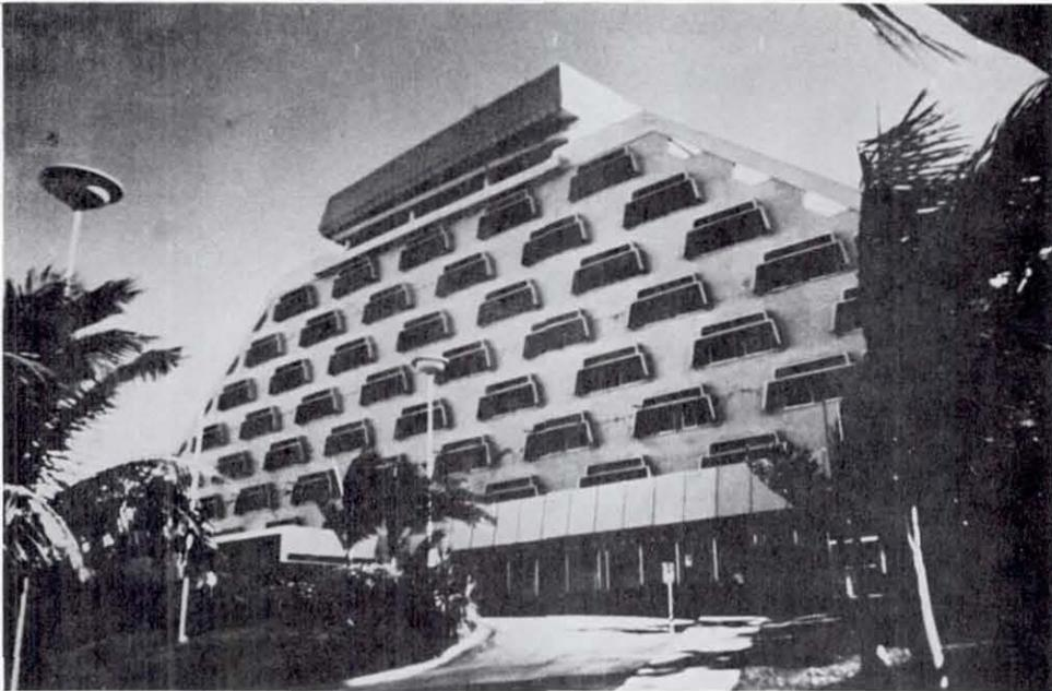
Figure 8 The penthouse of this hotel rotated during the Managua, Nicaragua earthquake, December 23, 1972.<sup>5</sup>
