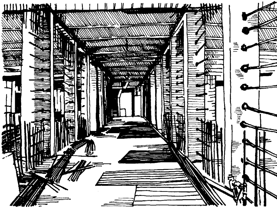
COLUMN TIES FOR NEW SHEAR WALL Figure 17.8
