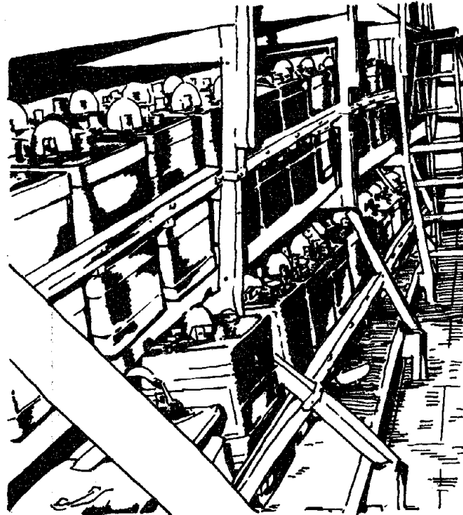
DISRUPTION OF POWER SOURCE COMMUNICATIONS BUILDING - 1964 ALASKA EARTHQUAKE Figure 13.9
