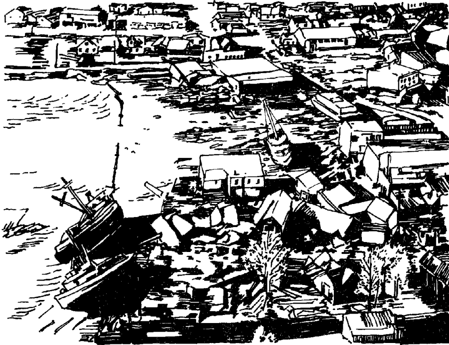
TSUNAMI DAMAGE KODIAK, ALASKA - 1964 ALASKAN EARTHQUAKE Figure 4.3
