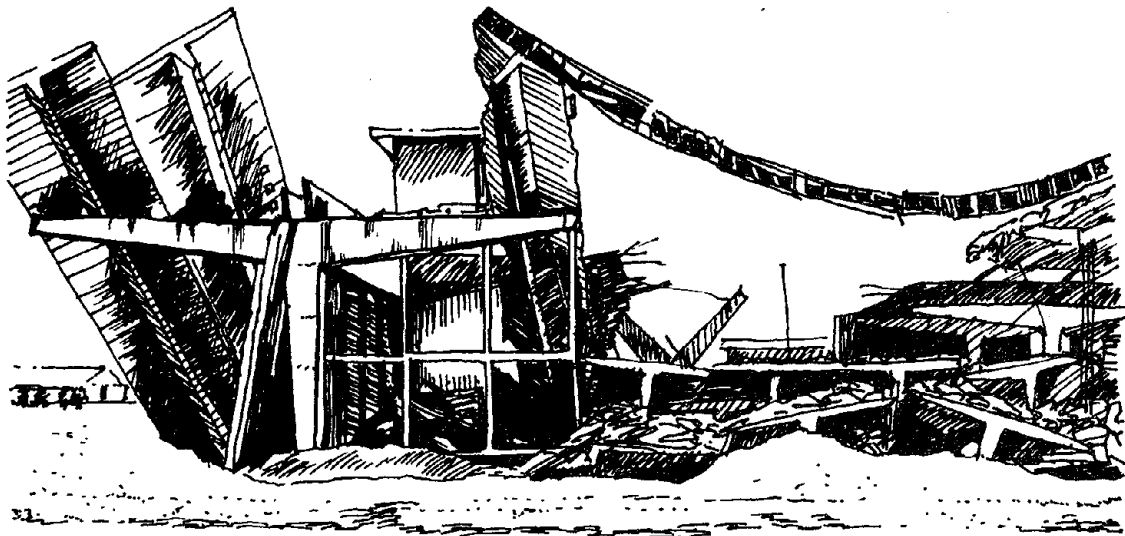
PRECAST CONCRETE FAILURE ALASKA SALES & SERVICE BUILDING - 1964 ALASKA EARTHQUAKE Figure 11.4
