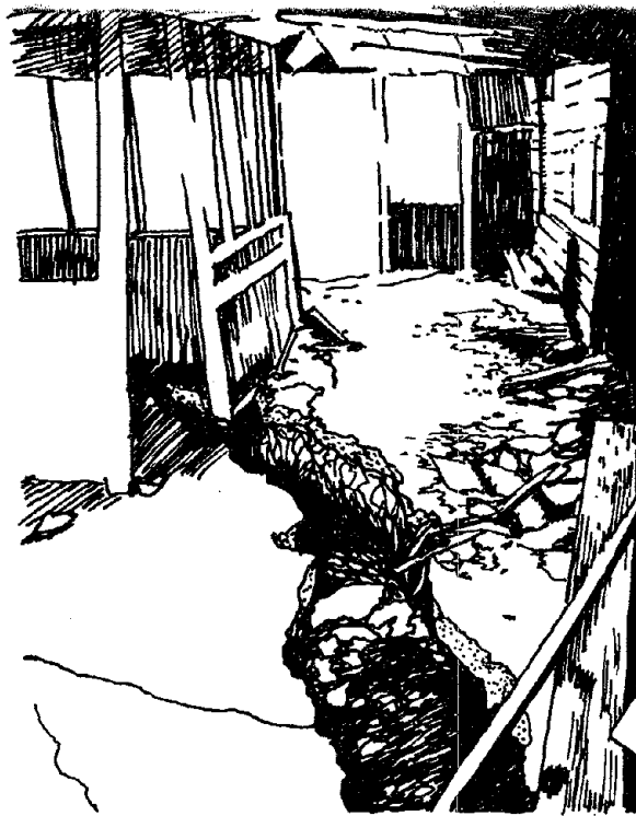
FAULTING THROUGH BUILDING JUVENILE FACILITY - 1971 SAN FERNANDO EARTHQUAKE Figure 4.1
