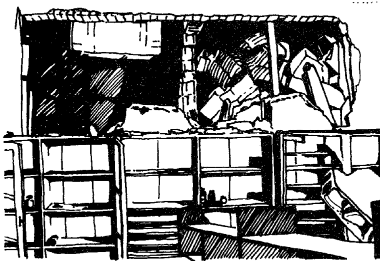
WALL DAMAGE BY ELEVATOR COUNTERWEIGHT BAUTISTA HOSPITAL - 1972 MANAGUA EARTHQUAKE Figure 14.17
