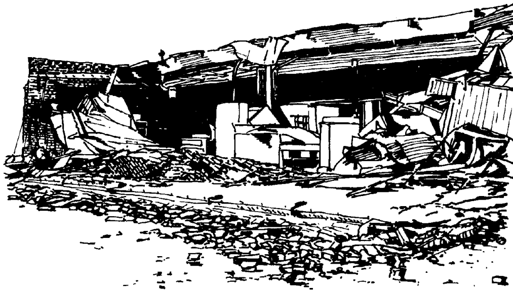
FAILURE OF PLYWOOD DIAPHRAGM Figure 17.12
