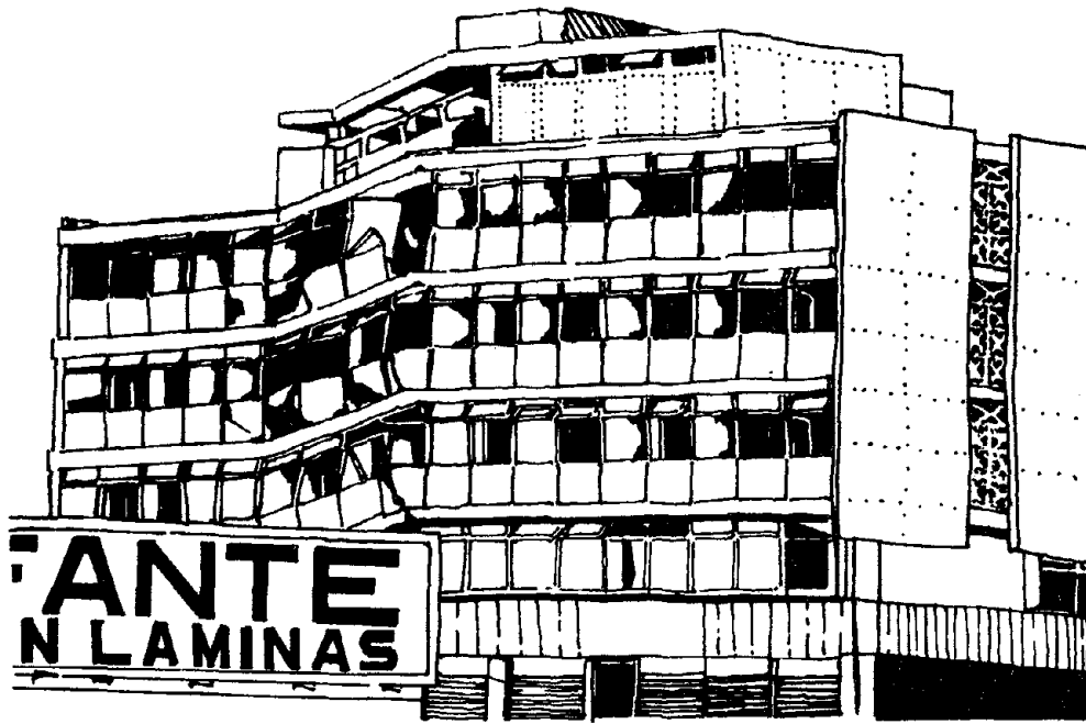
COLLAPSE OF OPEN PORTION OF BUILDING TERMINAL HOTEL - 1976 GUATAMALA EARTHQUAKE Figure 11.9
