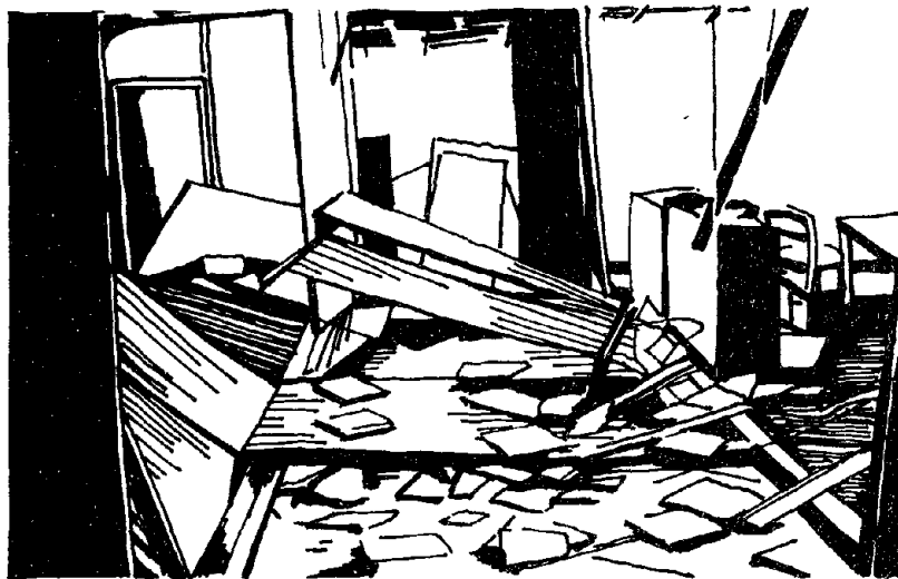
CEILING FAILURE 1972 MANAGUA, NICARAGUA EARTHQUAKE Figure 13.1
