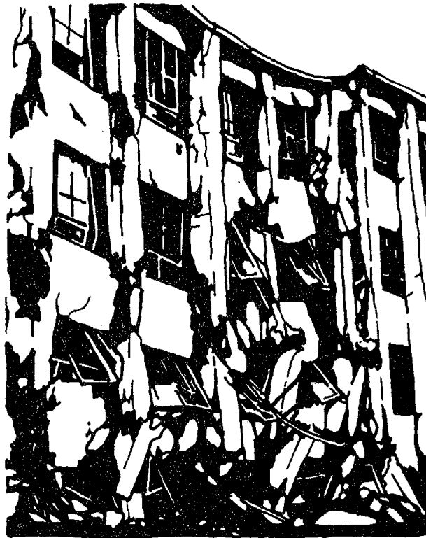
FAILURE OF SMALL COLUMNS SCHOOL BUILDING - 1968 JAPAN EARTHQUAKE Figure 12.10
