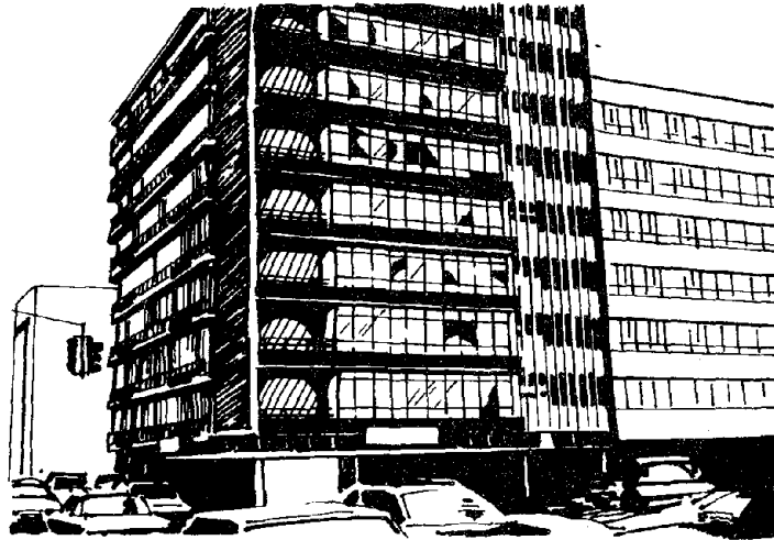
GLASS FAILURE OFFICE BUILDING - 1974 LIMA, PERU EARTHQUAKE Figure 14.11
