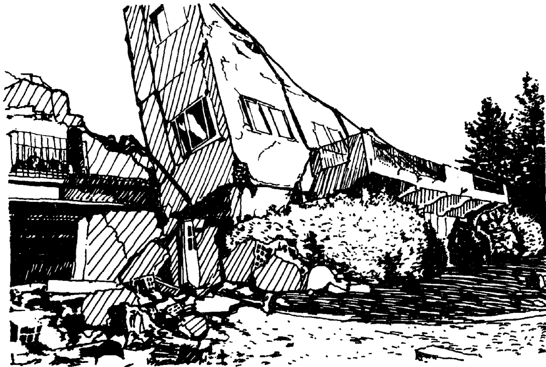
VETERANS HOSPITAL – 1971 SAN FERNANDO EARTHQUAKE Figure 10.8
