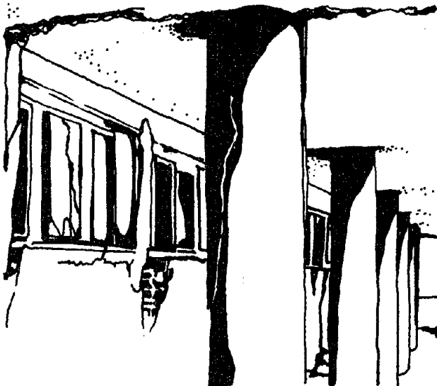
COLUMN FAILURES STUDENT CLUB - 1963 SKOPJE EARTHQUAKE Figure 11.8
