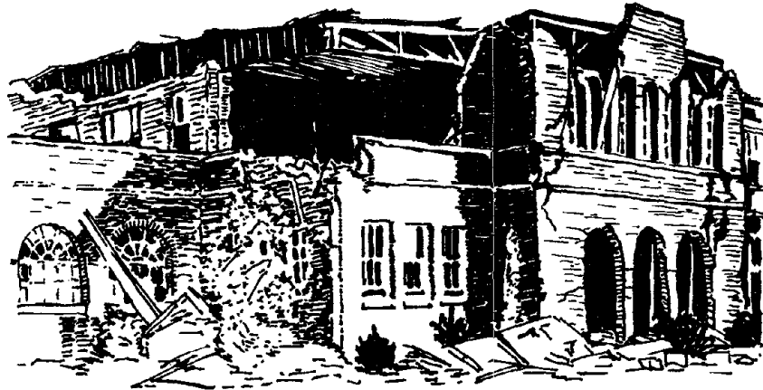
COLLAPSED SCHOOL BUILDING HAMILTON SCHOOL - 1933 LONG BEACH EARTHQUAKE Figure 7.1
