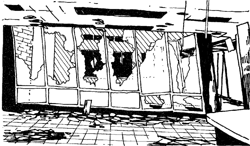
GLASS BREAKAGE OLIVE VIEW HOSPITAL - 1971 SAN FERNANDO EARTHQUAKE Figure 13.2
