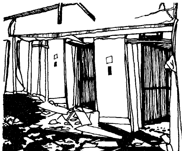
ELEVATOR DAMAGE - 1971 SAN FERNANDO EARTHQUAKE Figure 14.16
