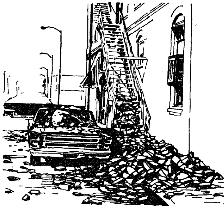
UNREINFORCED PARAPETS - 1969 SANTA ROSA EARTHQUAKE Figure 13.3
