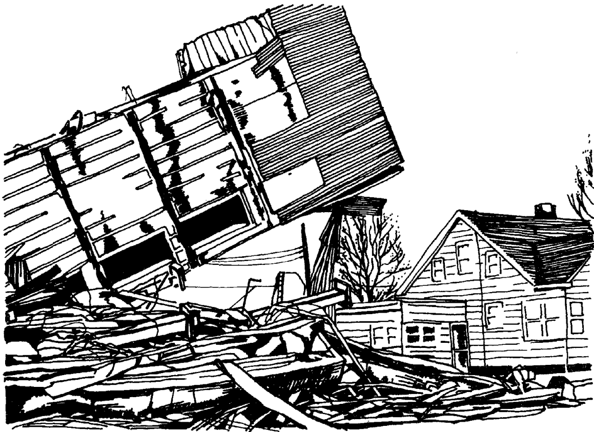
FOUR SEASONS APARTMENTS - 1964 ALASKA EARTHQUAKE Figure 11.6
