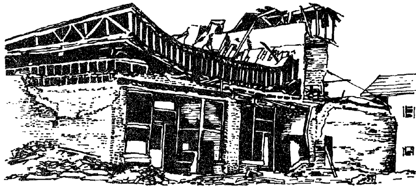
DAMAGED "CLASS C" BUILDING TEHACHAPI LODGE HALL - 1952 KERN COUNTY EARTHQUAKE Figure 10.7
