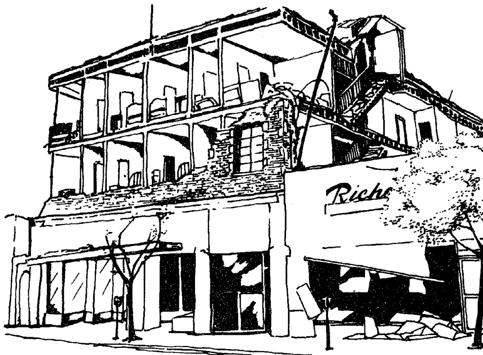
MASONRY WALL FAILURE - 1971 SAN FERNANDO EARTHQUAKE Figure 10.4
