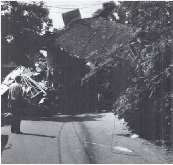
Figure 9. House fallen onto Meadowlark Drive, October 5, 1978
