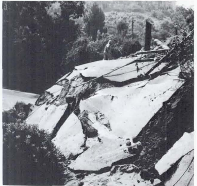
Figure 12. Toe of the landslide at Oriole Drive, October 5, 1978
