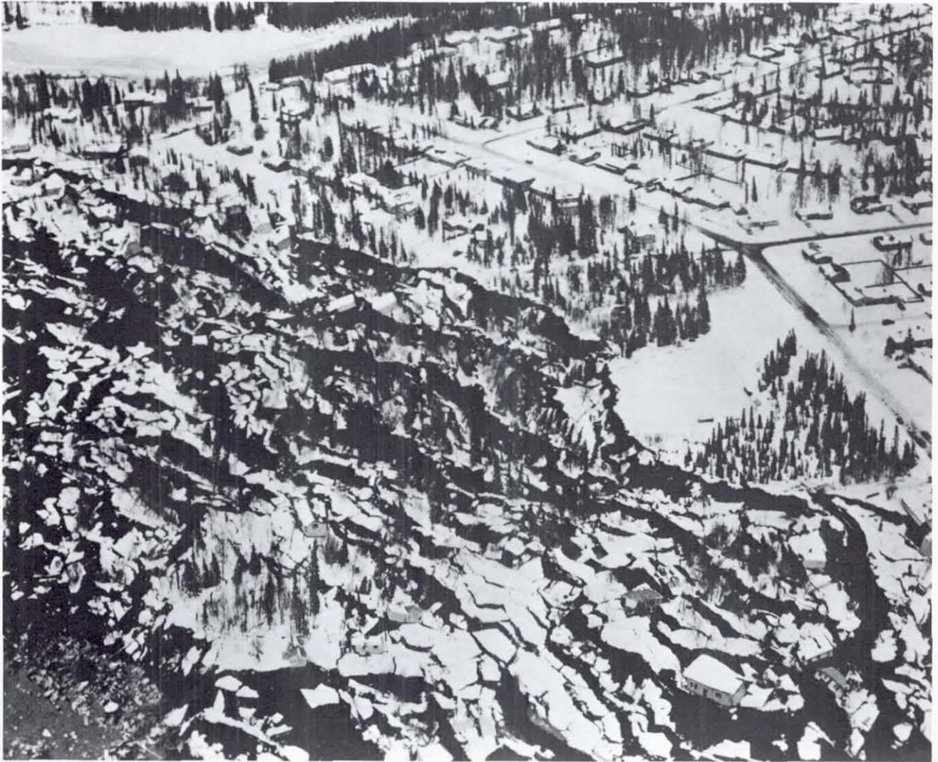
Figure 26. Aerial view of Turnagain Heights slide (Source: Krauskopf, 1970, p. 252)
