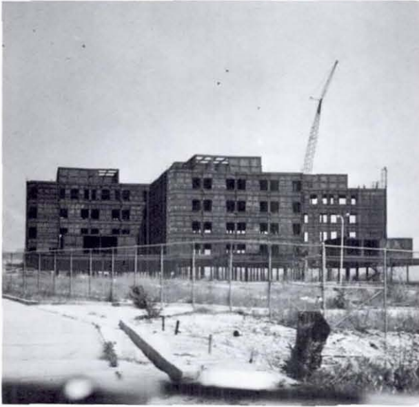
Figure 24. Olive View Hospital building under construction, Spring 1978
