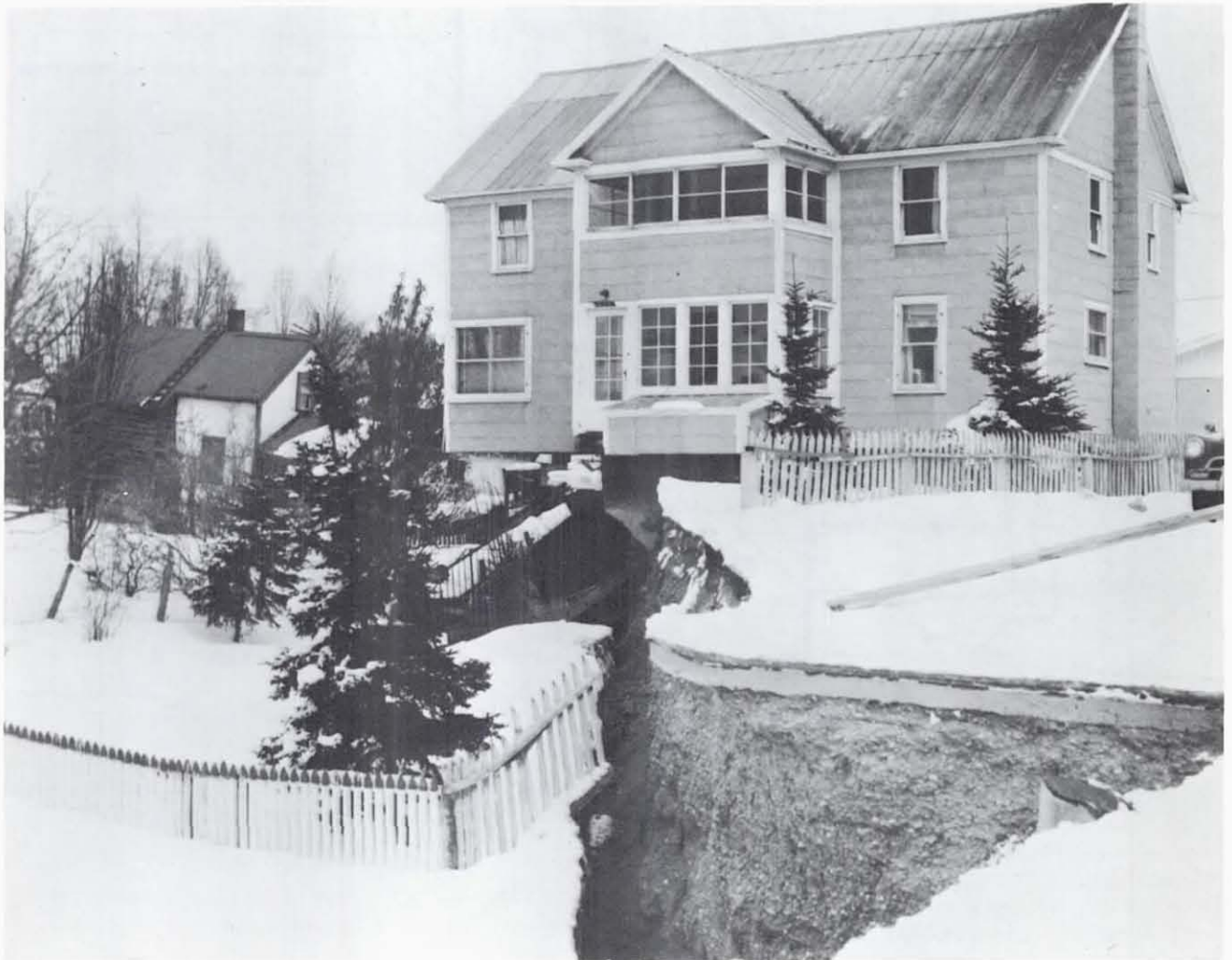
Figure 21. Relatively undamaged house at edge of graben, L Street slide Photo Credit: Stewart's Photo Shop, Anchorage
