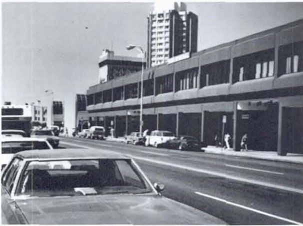
Figure 17. Shopping malls on north side of Fourth Avenue at top of buttress. Anchorage-Westward Hotel in background, Summer 1978.
