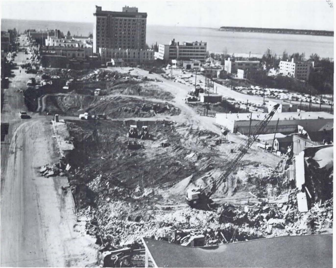
Figure 14. Debris clearance from the Fourth Avenue slide area. Fourth Avenue is on the left; the slide moved toward the right. The high-rise building in the background is the Anchorage-Westward Hotel. (Source: Eckel and Schaeni, 1970, p. 173) Photo Credit: U.S. Army Corps of Engineers
