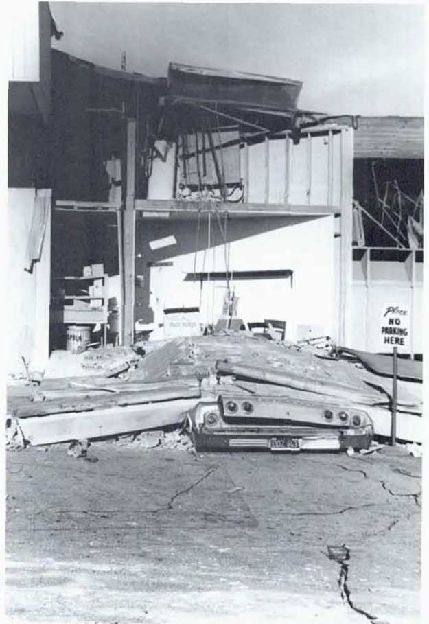
Figure 22. Collapsed Boys Market, corner of Glenoaks Boulevard and Hubbard Avenue (Source: Jennings, P.C., ed., 1971, p. 475)
