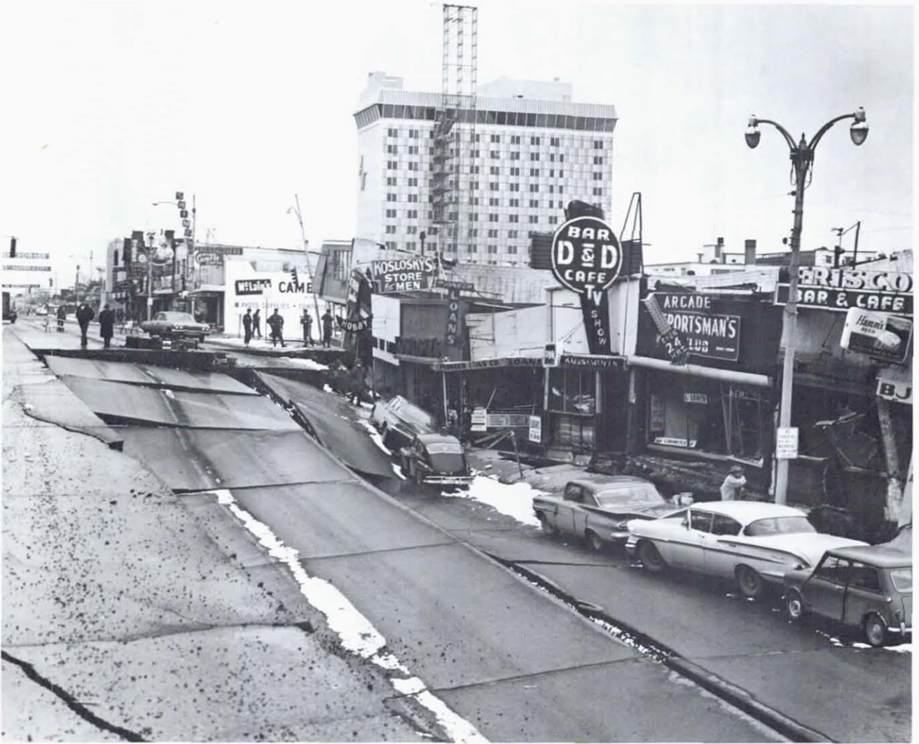
Figure 11. Building damage along Fourth Avenue caused by the slide. The 14-story Anchorage-Westward Hotel, still under construction, is a few feet from the slide area in the right background. (Source: Norton and Haas, 1970, p. 258) Photo Credit: U.S. Army
