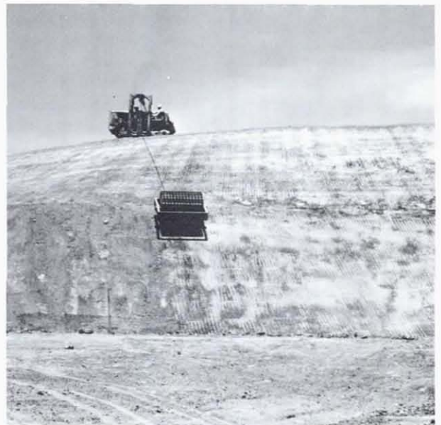
Figure 20. Compaction of lower gravity buttress, July 1979
