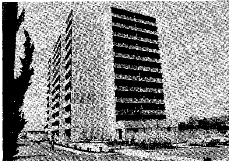
FIG. 1 WESLEY MANOR BUILDING, CAMPBELL, CA
