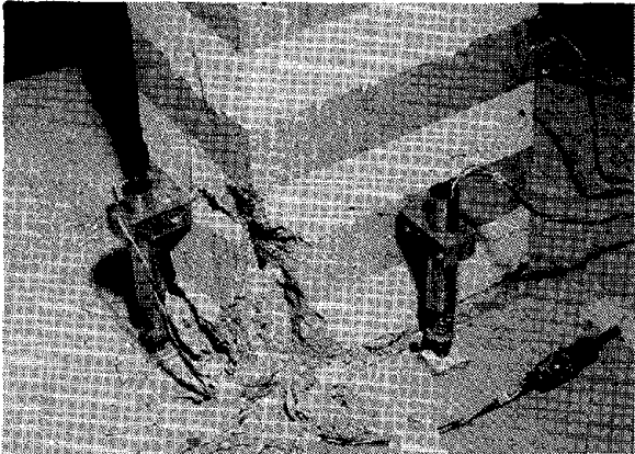
Fig. 8 Damage at Column Base
