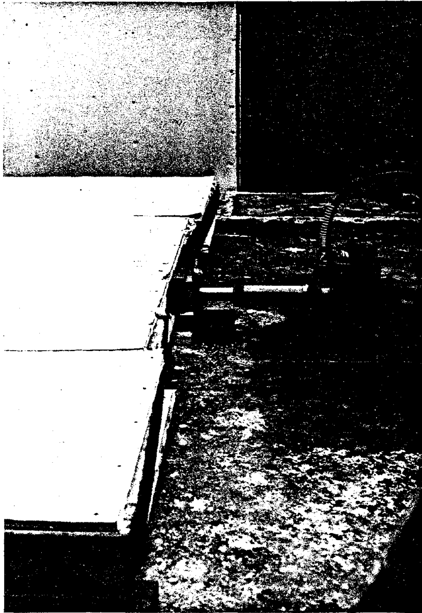
FIGURE 3-8. TRANSFER OF LOAD AT JACK TO WOOD FRAMING MEMBERS
