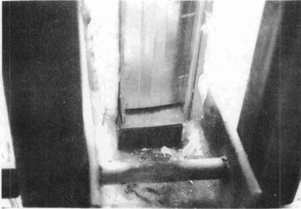
Fig. 46: Partition Test Specimen P2: Failure @ Loading End Stud @ Bottom Runner
