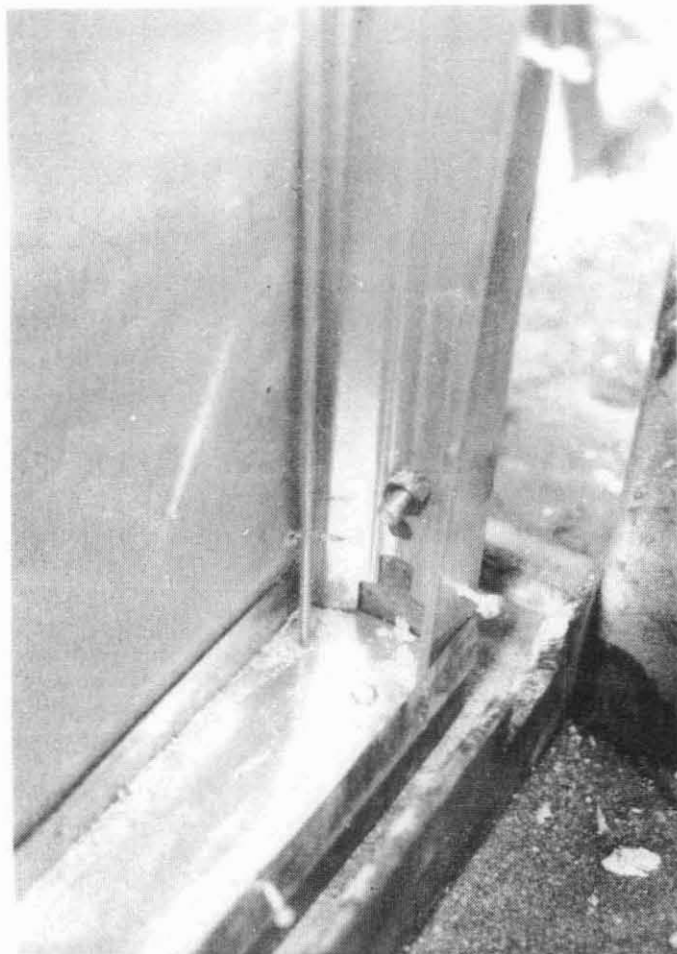
Fig. 75: Partition Test Specimen P7: Detail at Uplift Restraint Strap
