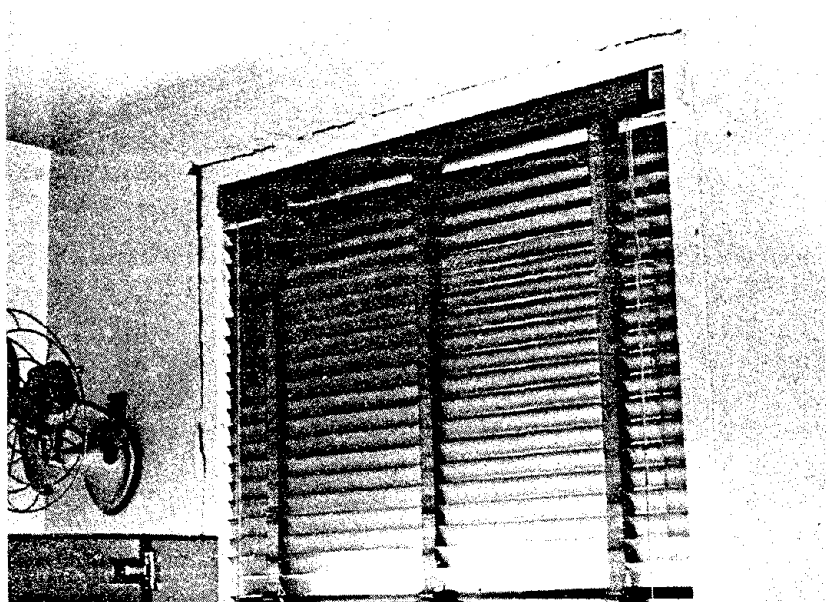
FIGURE 3-16. WINDOW JAMB IN SIXTH FLOOR JOLTED OUT OF PLACE BY STRONG SHAKING OF BUILDING 3
