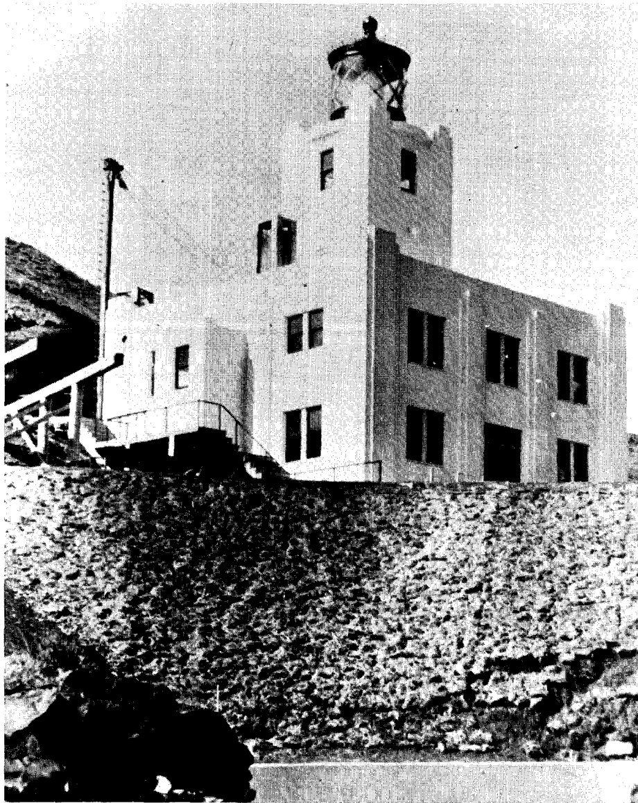
Scotch Cap Light Station, destroyed by Tsunami of 1946, killing all five occupants. Built in 1940 of concrete to replace a wooden structure built in 1903, it stood 60 feet high and 92 feet above water level. (Credit: U.S. Coast Guard.)
