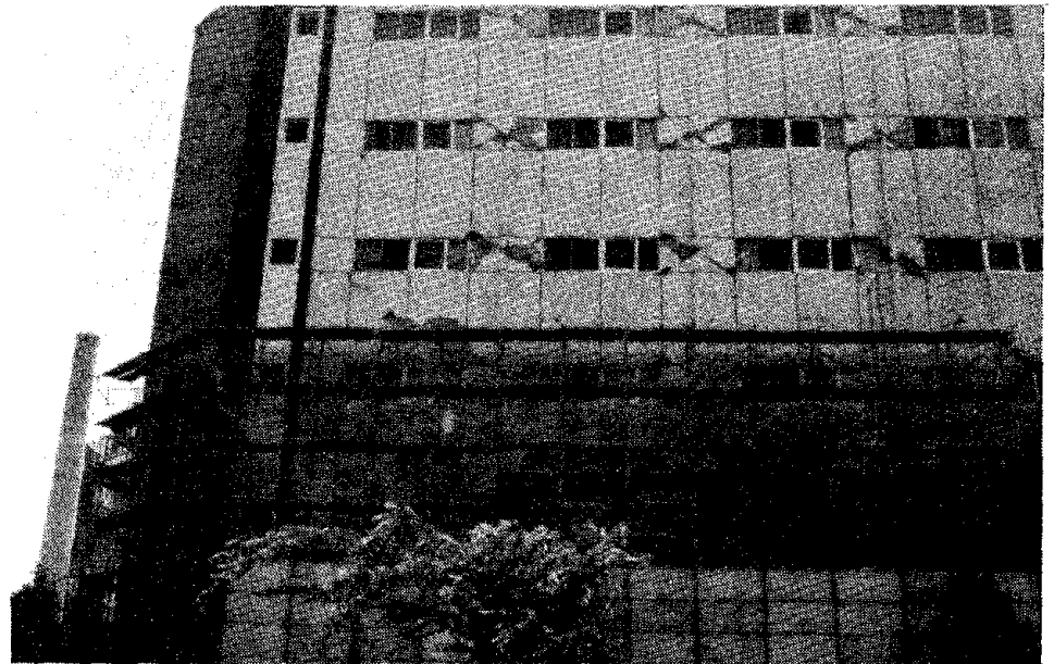
Figure VIII-22. Weak columns and strong beams commonly lead to damage during earthquakes, Maruhon building, 1978 Sendai Japan earthquake.
