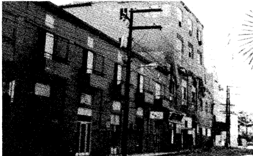
Figure IX-1. Gran Hotel damaged in the 1972 Managua Nicaragua earthquake.
