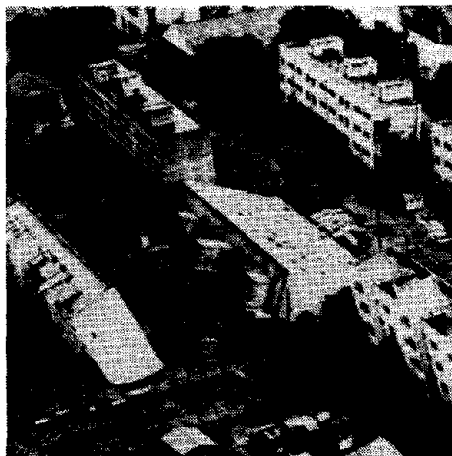
Figure II-6. Liquefaction, 1964 Niigata Japan earthquake.
