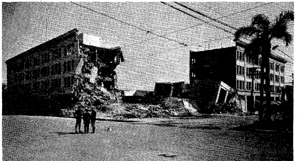
Figure VI-10. Collapse of re-entrant corner of the L-shaped San Marcos Building, 1925 Santa Barbara California earthquake.
