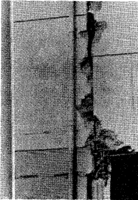
Figure IX-3. Damage due to pounding, Anchorage Westward Hotel, 1964 Alaska earthquake.
