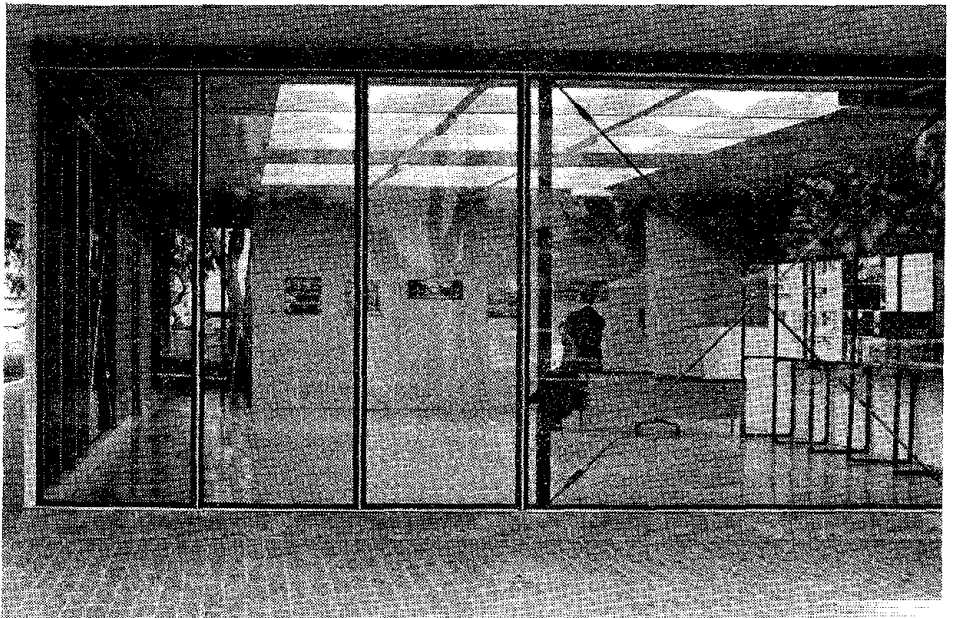
Figure XIV-19. Braced light steel frame. SCSD prototype building. Stanford University, California. BSD, Inc., architects.
