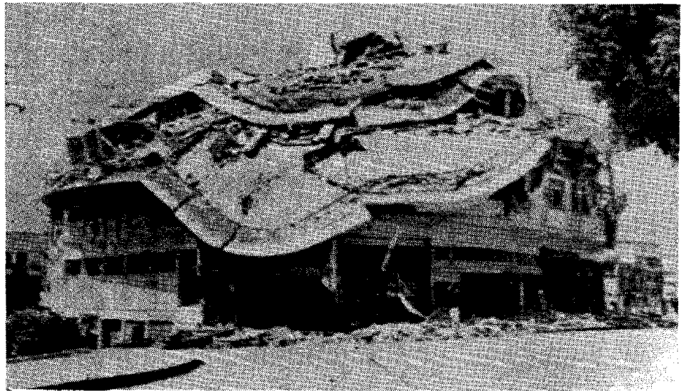
Figure VII-11. Collapse of upper story of inverted setback, Sud Building, 1960 Agadir Morocco earthquake.
