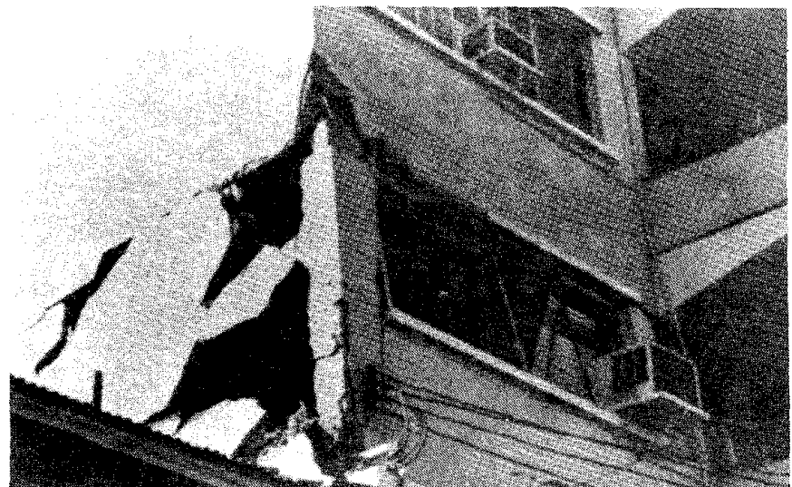
Figure IX-2. Pounding damage suffered by the Lang Building, in the same earthquake. For another view of the Lang Building, see Figure VII-8.
