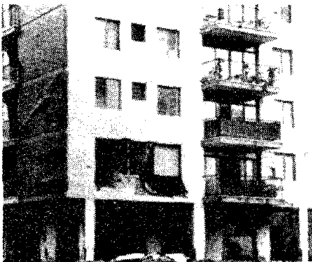
Figure VIII-5. Damage to a soft first story building, the San Bosco building, in the 1967 Caracas Venezuela earthquake.
