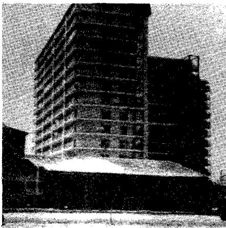
Figure VI-15. General view of the L-shaped Sunnyheights apartment building.
