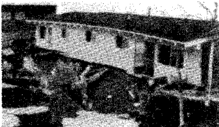
Figure IV-8. Small size allows askew house to remain more or less intact following 1964 Anchorage Alaska earthquake.
