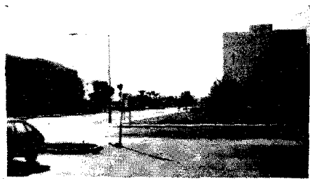
Figure IV-27. 1979 Imperial Valley California earthquake caused no structural damage to the old (1924) Imperial Valley Court House, left, but near collapse of the new (1969) Imperial County Services Building, right.
