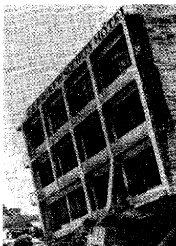
Figure V-10. An example from the 1976 Mindanao Philippines earthquake of a building located on a corner lot. The New Society Hotel had two sides of rigid shear walls and two framed sides of greater flexibility. The amount of torsional movement accompanying ground story collapse is readily apparent.
