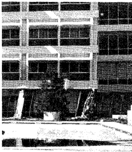
Figure I-2. Olive View Hospital following the 1971 San Fernando California earthquake.
