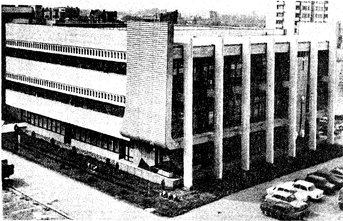
Figure 23 Computing center before the earthquake.
