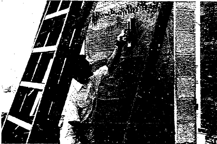
FIGURE 3-12. APPLICATION OF SECOND COAT OF PLASTER TO REINFORCE WALL SPECIMEN
