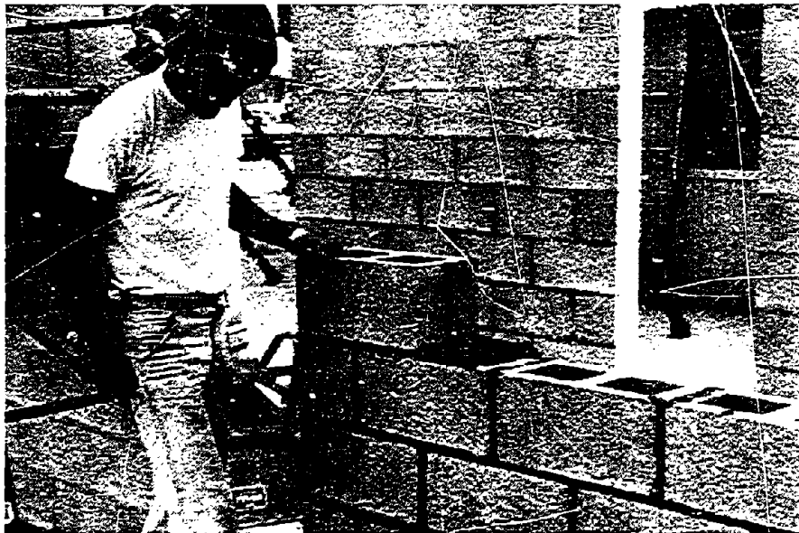
FIGURE 3-7. PLACEMENT OF THROUGH-WALL UNITS ON MORTAR AT FACE SHELL
