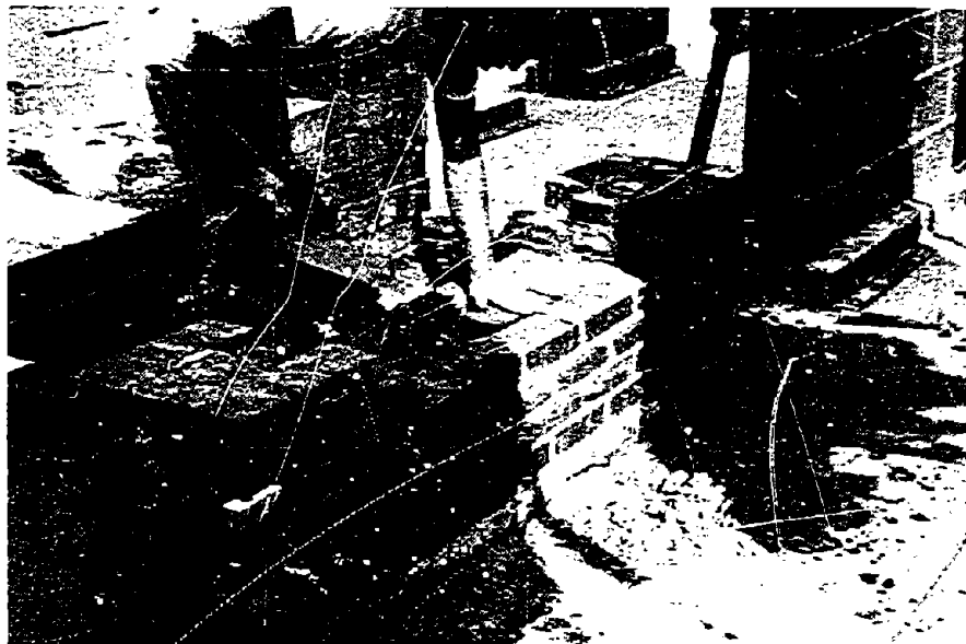
FIGURE 3-6. PLACEMENT OF INTERIOR WYTHE IN THREE-WYTHE MASONRY
