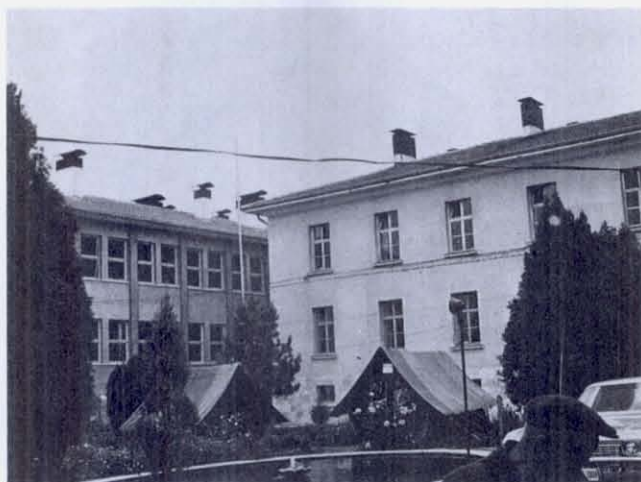
FIGURE 51 The government building in Burdur, made of hard stone set in lime mortar, had some plaster cracking inside and perhaps some mortar joint cracking, but not extensive. The building continued in use after the earthquake. The chimneys on this building, some of which had guy wires, and those on the building next door did not fall or appear to be damaged. Tents in the garden were used by officials for handling relief work.
