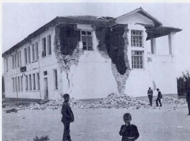
FIGURE 29 This 30-year old primary school in Hacilar, 22 km SW of Burdur, partly brick, partly coarse masonry, was laid in mortar which easily could be powdered in the fingers. Perhaps the nonsymmetry of the second story was responsible for the damage there being greater than in the first story.
