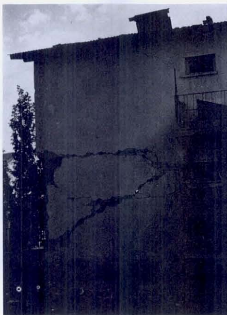
FIGURE 45 Both stories of the south face, southwest corner.
