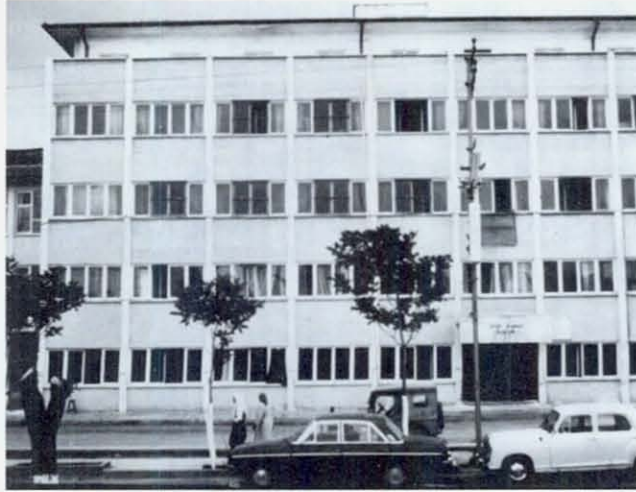
FIGURE 62 A front view of Burdur's hospital, showing permanent displacement to the right in the lowest story. The structure on the left is a second and third floor passageway to an older masonry building, which was severely cracked.
