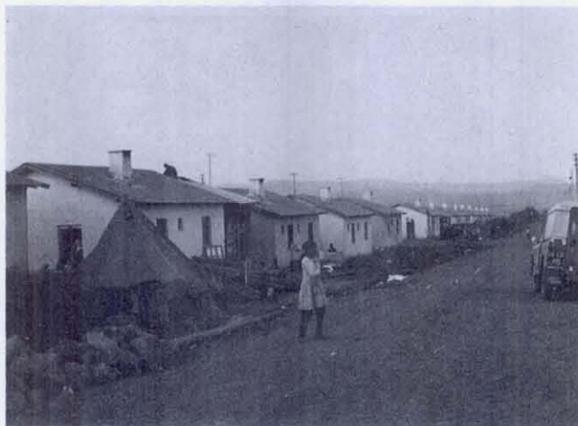
FIGURE 85 A closer view of the undamaged resettlement houses. The houses are of masonry, contain 55 \text{ m}^2 gross area, and are on lots of 450 \text{ m}^2 . They cost $1,300, payable over a 20-year period with no interest charge. Water piped to a house costs $35 extra, and electric service is $40 extra. The chief complaint voiced by the owners of the houses is their small size. One resident is seen on the roof of an addition he is just completing. The complete absence of damage suggests that ground motion here was not as strong as in surrounding areas.
