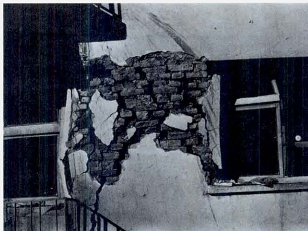
FIGURE 43 A close-up of the pier west of the west balcony, north side. Bricks in the Bingöl region were soft, but mortar was of good quality.
