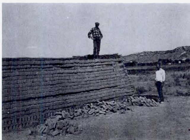
FIGURE 91 A roasting stack being constructed of air-dried bricks. Thin layers of coal can be seen between some of the layers of bricks. These bricks sell for about one cent each in the brickyard.
