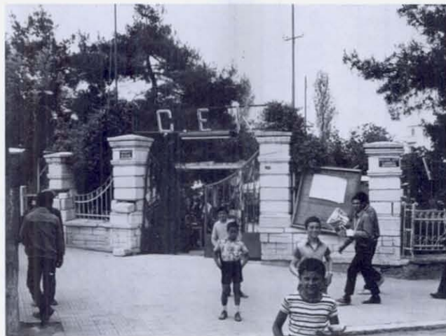
FIGURE 49 Gate posts at the park entrance in Burdur were shattered, whereas across the street, some 200 feet distant, rather tall chimneys in the government building (Figure 51) did not fall.
