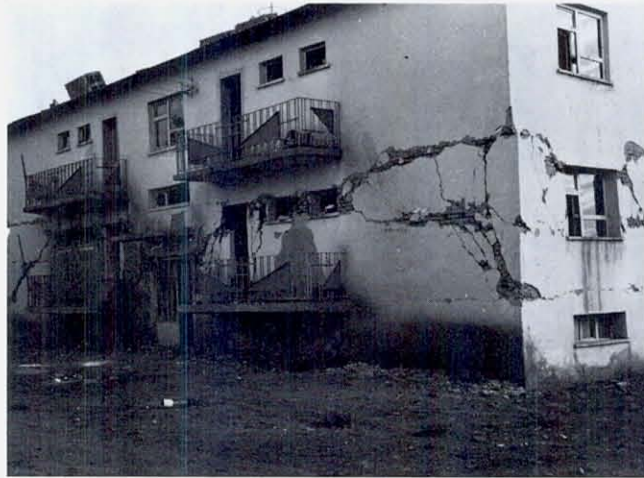
FIGURE 46 The south face, at the southeast corner.
