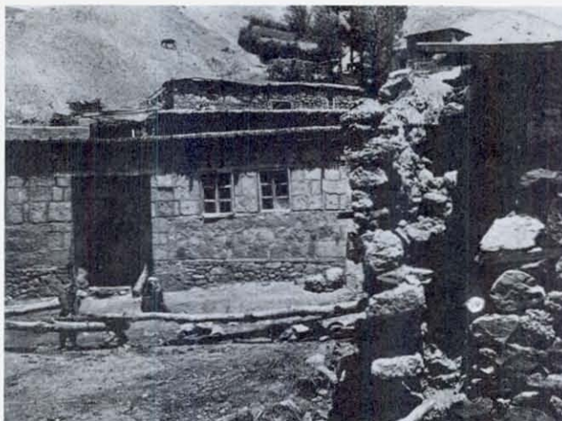
FIGURE 26 Most of the houses in Hacilar are one-story, of uncemented stone, with wood bond members built into the walls. In the foreground the bond members failed to hold the corner together. In the background the building with squared stones appears to be laid in cement mortar, but the mortar is on the surface of the joints only, and no mortar was observed inside the joints. The earthquake displaced some stones perpendicular to the wall and opened cracks between others. The villagers said the squared stones came from "ancient constructions."
