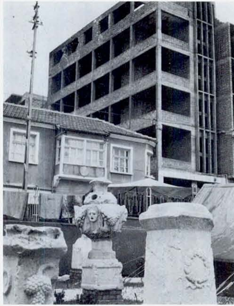
FIGURE 54 A top-heavy stone carving, about 2 m tall, probably originally a fountain, could be easily rocked by hand, but was not toppled by the earthquake. In the background is seen the bus station building, under construction, which suffered fallen brick walls in the penthouse.
