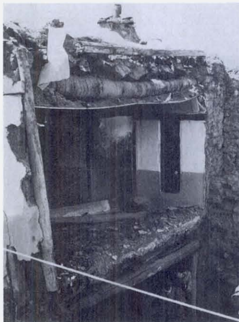
FIGURE 20 A close-up view of the house in Figure 19, showing the heavy roof and the walls of uncemented stone and adobe.
