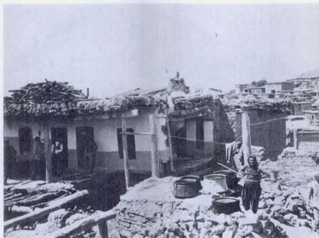
FIGURE 19 This type of construction, in Askeriye, near Burdur, is common in villages on sloping ground. One- and two-story houses are intermingled, the roofs of the one-story houses serving as working platforms. One can easily imagine that when an owner needs more living space, he simply lays up more adobe walls on top of the first story. The tremendous weight and fragility of such structures is frightening.
