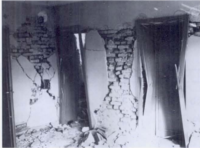
FIGURE 48 Interior walls of the building shown in the preceding figures were just as badly shattered as exterior walls.
