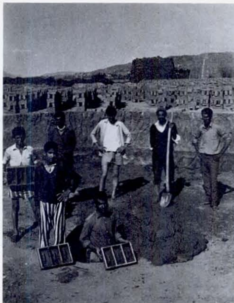
FIGURE 90 A brickyard in Genç, near Bingöl. Mud, soaked for 12 or so hours, is brought to the man in the pit who fills the molds, using fine sand to prevent the mud from sticking to the molds. The bricks are dumped on the ground for air drying and later piled into small stacks. As shown in Figure 91, a large burning stack is constructed of air-dried bricks, with finely crushed coal sprinkled between layers of bricks, and then plastered over with mud, ignited, and left to smolder for 15 or so days. Bricks made in this manner are soft and relatively weak. Sometimes the bricks are roasted a second time to improve the quality.
