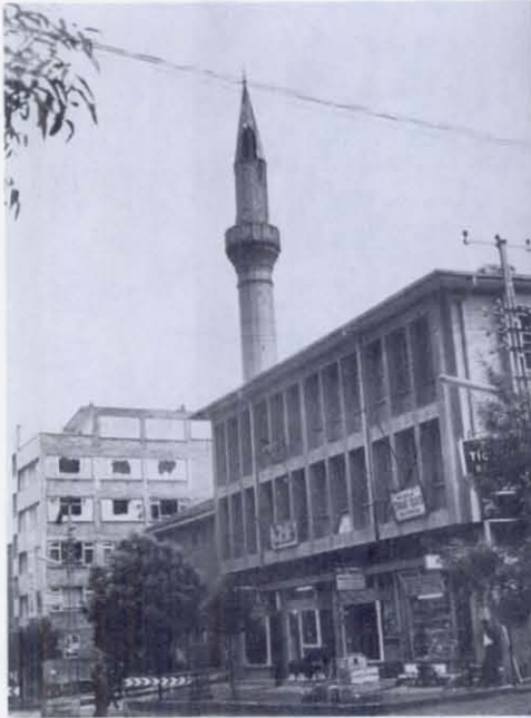
FIGURE 56 Most of the unreinforced masonry minarets in Burdur suffered displaced stones near the top. Lower portions did not show damage. On the other hand, in Yazıköy, 20 km SW, this minaret was broken off at the base. The sheet metal cap covering a wood frame on top of the Tabac Mosque has been torn open by workmen in preparation for dismantling the top portion. Possibly the discontinuance above the balcony of the interior stone steps, built between a central stone column and the outside wall, was responsible for the damage being localized in the top section. The reinforced concrete building with broken windows in the background (shown later) had heavy partition damage as well as structural damage.
