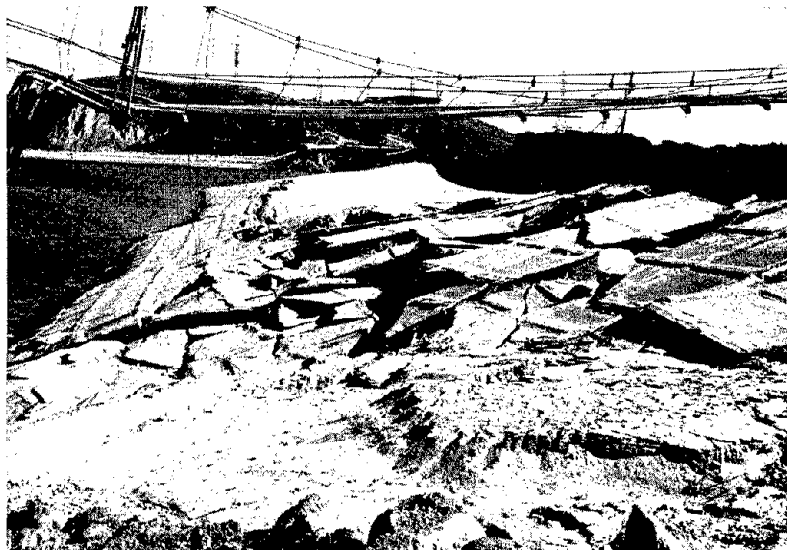
FIGURE 6 The Van Norman Dam, which was so severely damaged by the earthquake that 80,000 people living in the Valley below were evacuated because complete failure appeared imminent. They returned to their homes four days later, after the reservoir had been lowered to a safe level. Photograph courtesy of Earthquake Engineering Research Laboratory, California Institute of Technology.
