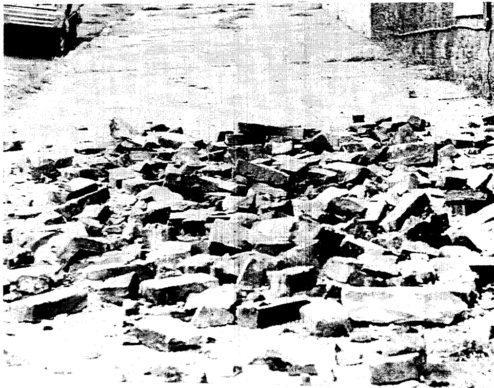
Figure 3. Brick fall from broken parapet in downtown Maysville, KY. Photo by courtesy of J. Parker.
