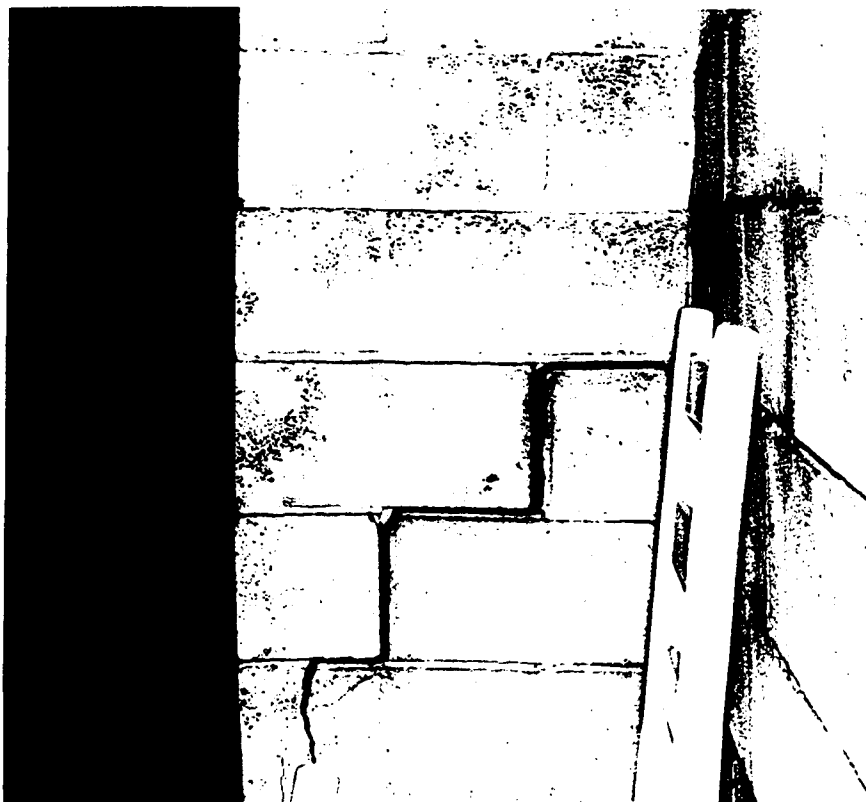
Figure 19. Cracked and bowed concrete block basement wall at Cooper residence in Flemingsburg, KY.
