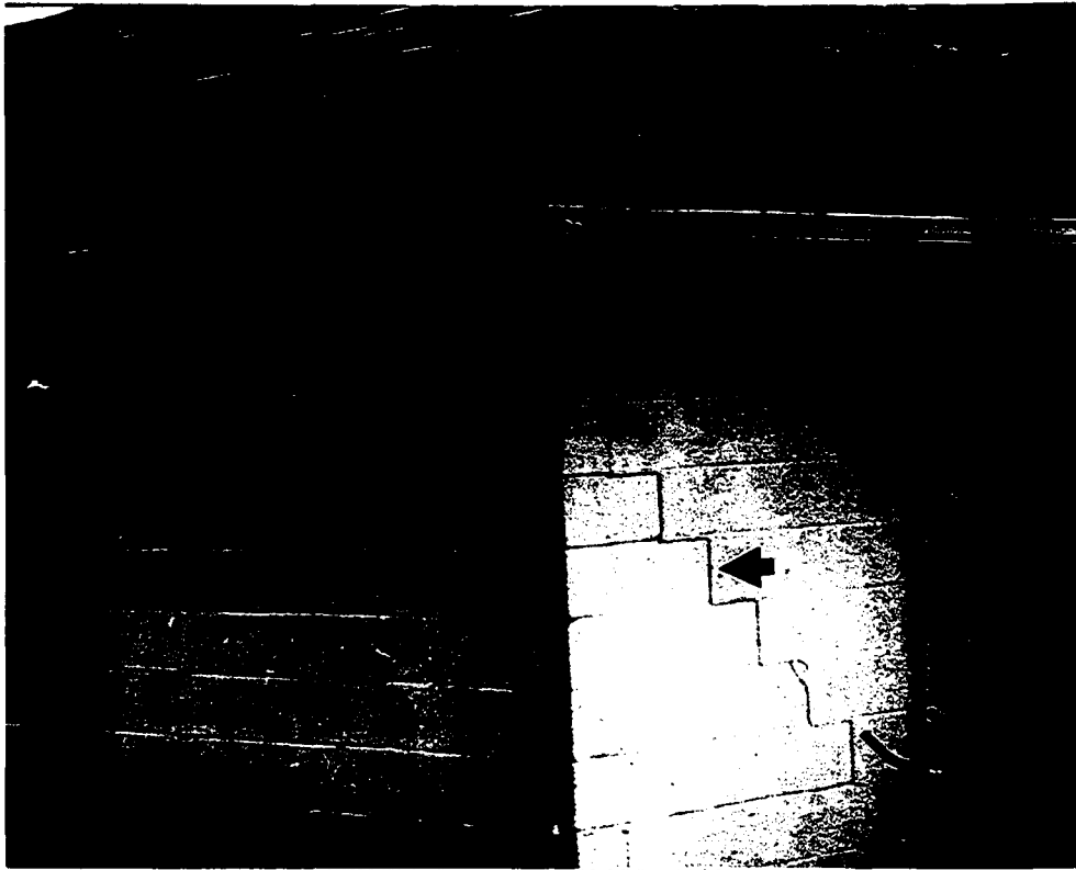
Figure 16. Cracks in concrete block structure at golf course in Mt. Sterling, KY. Photo by courtesy of J. Zollweg.
