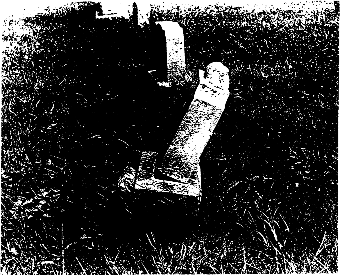
Figure 40. Example of a tombstone in the Sharpsburg cemetery that would have fallen if not for the metal rods connecting the top to the base.
