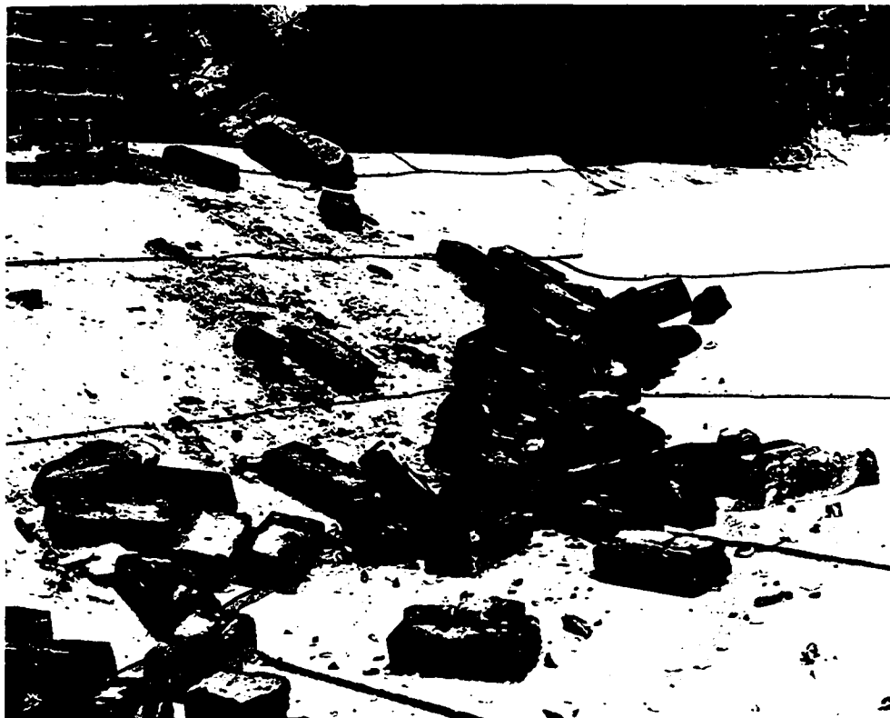
Figure 13. Chimney damage at two story frame Hall residence in Mt. Sterling. Notice poor condition of mortar.
