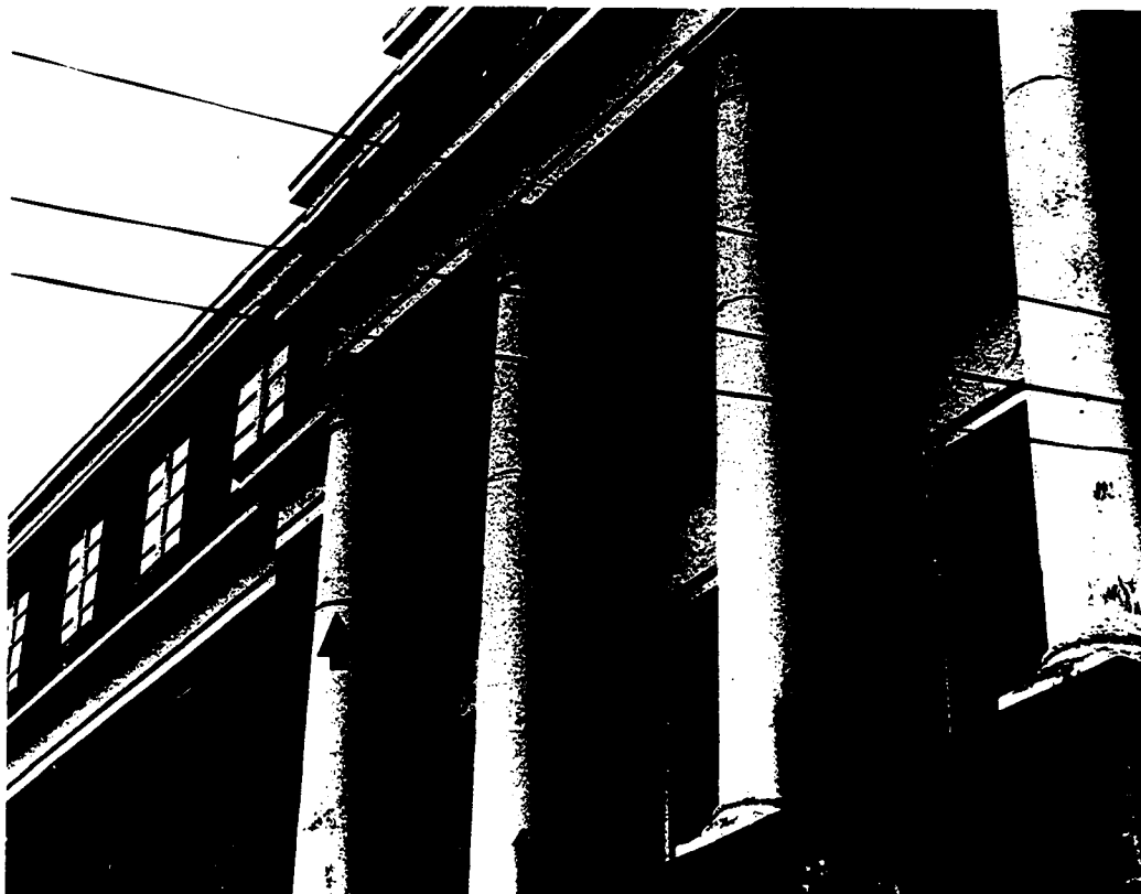
Figure A3. Columns at the front of the Hayswood Hospital in Maysville, KY that were displaced by as much as one inch at the joints.
