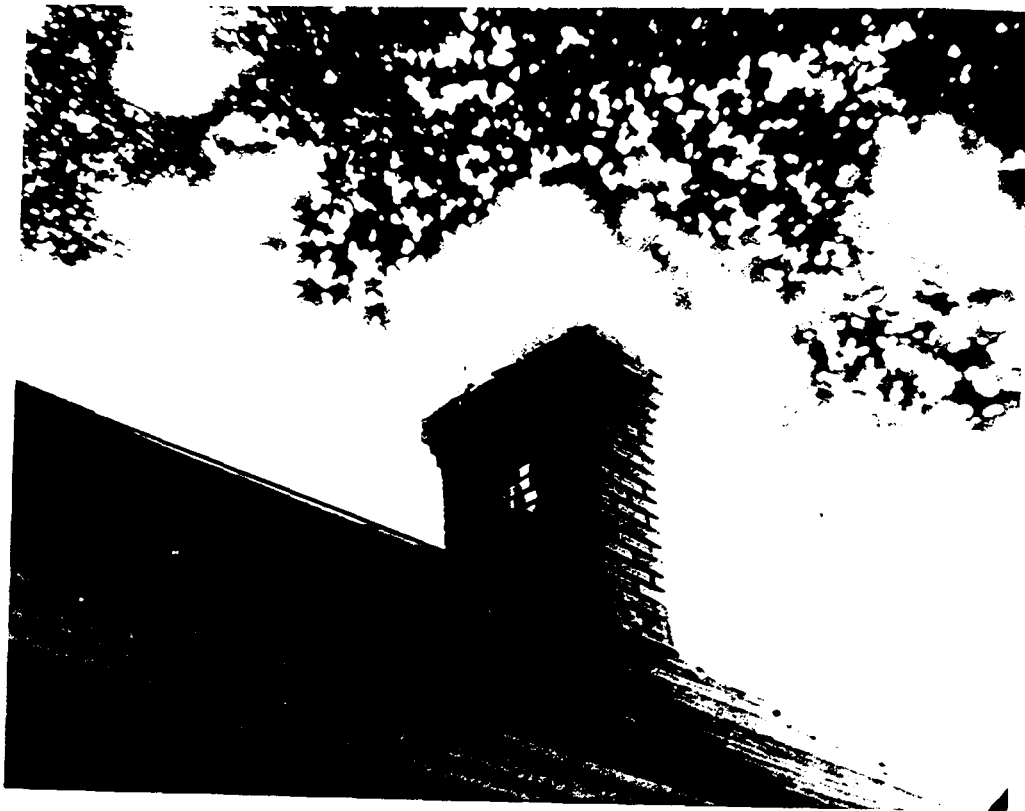
Figure 6. Chimney damage at Robert's residence in Sharpsburg, KY.
