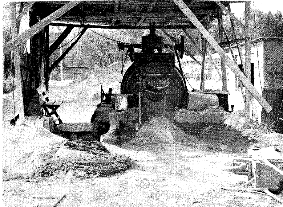
b. Batch plant concrete mixer.
