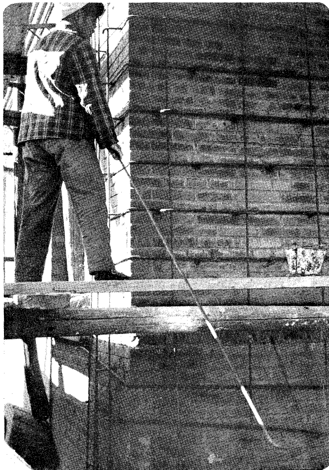
Figure 4.17 Close-up view of reinforcing steel bars.
