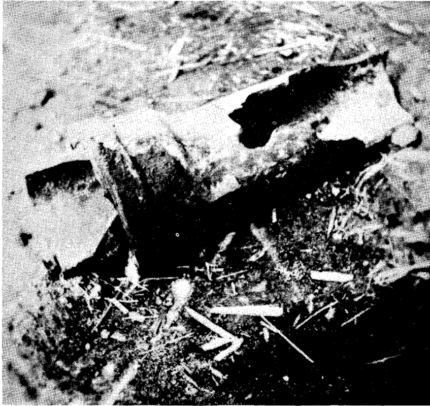
Figure 4.20 A ruptured pipe barrel.
