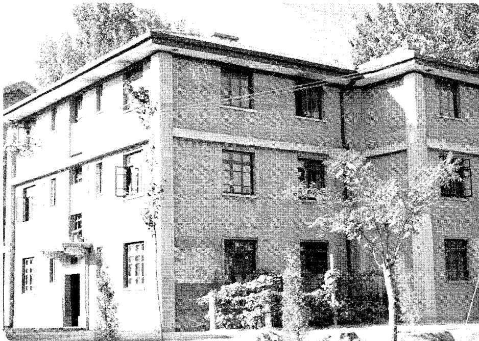
Figure 4.16 An apartment building in Beijing after strengthening.
