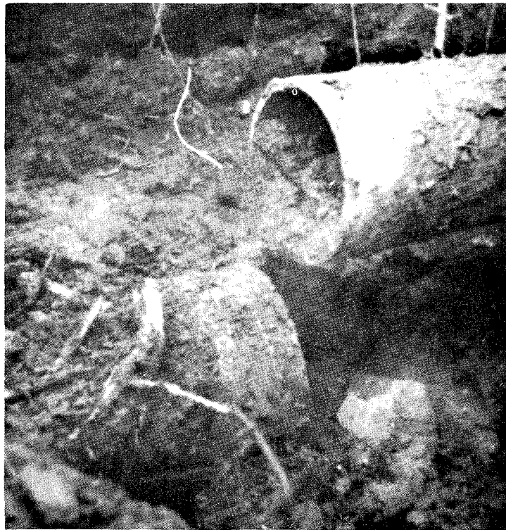
Figure 4.21 Joint separation of a water pipeline.
