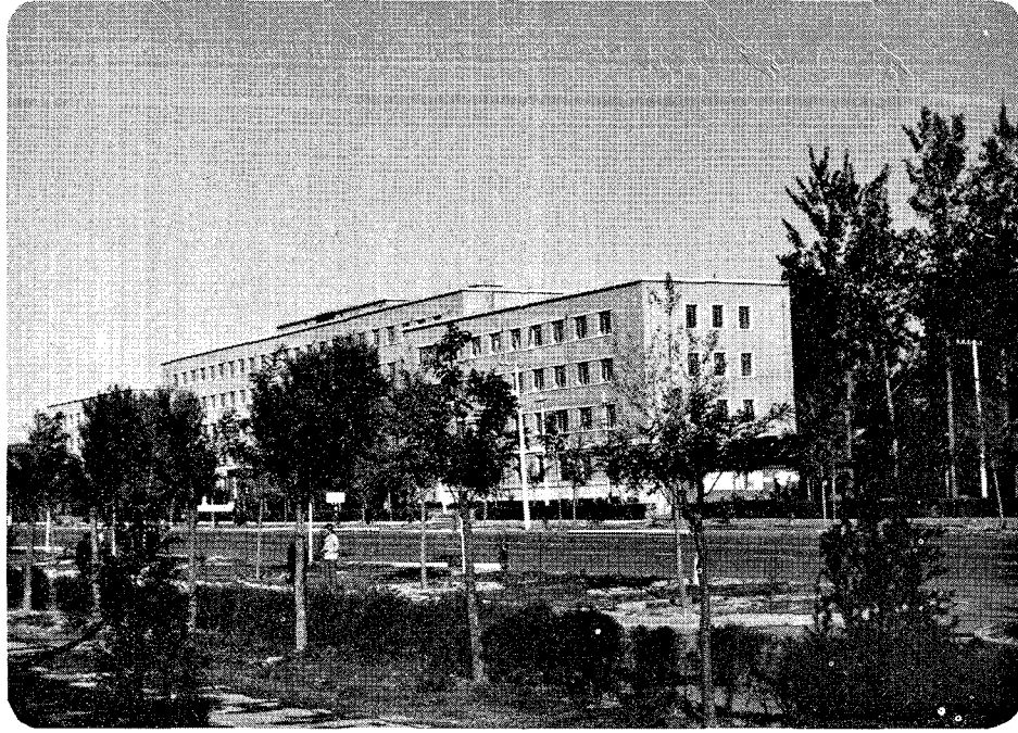
Figure 4.15 The Academy of Building Research after repair and strengthening.
