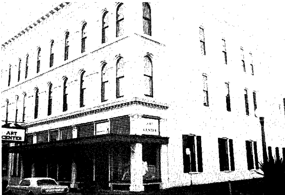
FIGURE 3-81. URM COMMERCIAL BUILDING, EUREKA, CA.
