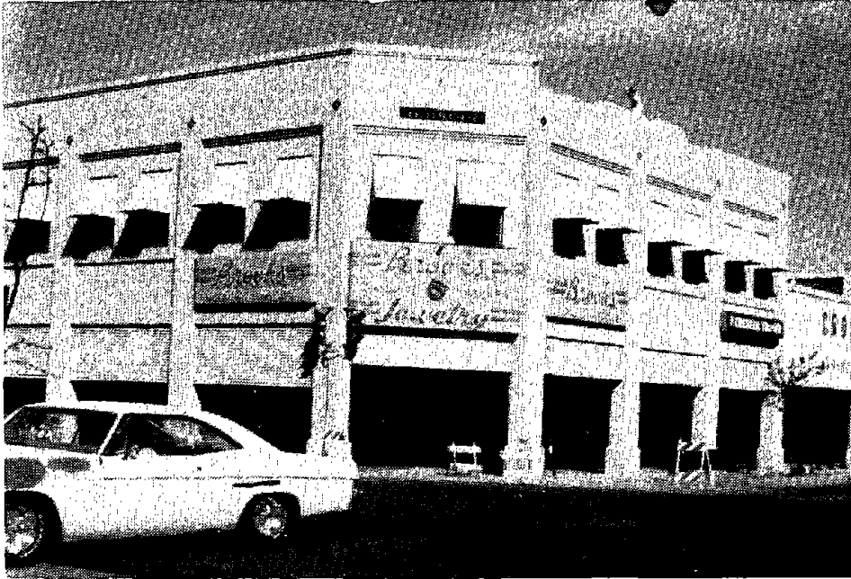
FIGURE 3-70. URM COMMERCIAL BUILDING, EL CENTRO, CA.
