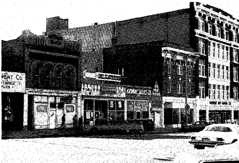
FIGURE 3-40. URM COMMERCIAL BUILDINGS, SALT LAKE CITY, UT.
