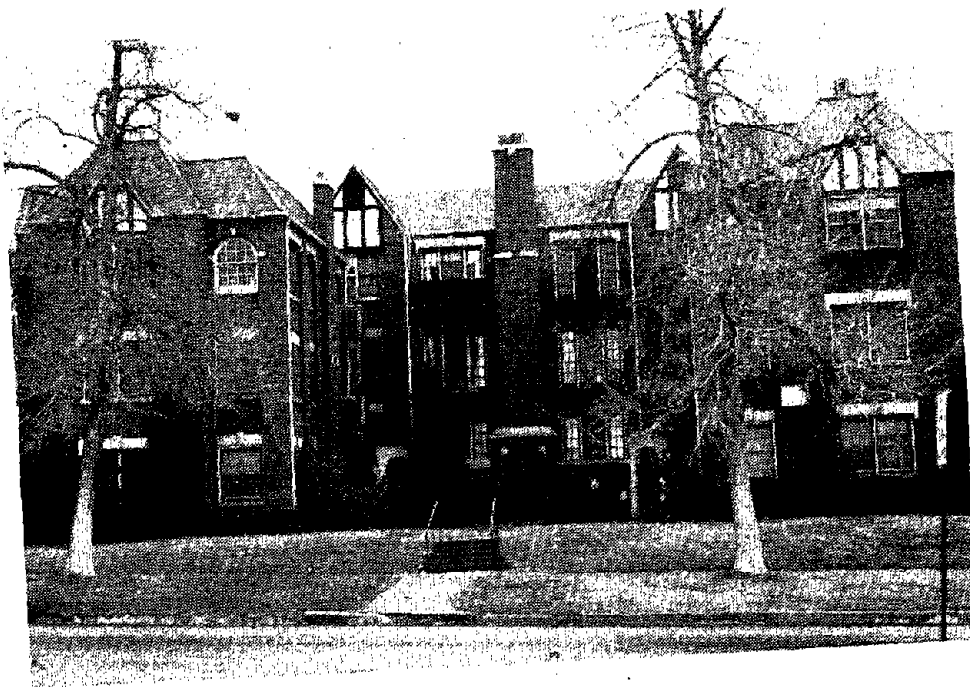
FIGURE 3-52. URM MULTI-FAMILY HOUSING, SALT LAKE CITY, UT.
