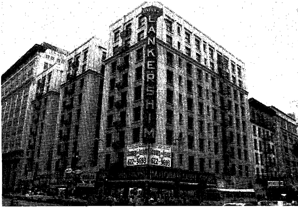
FIGURE 4-7. LARGE URM BUILDING WITH MASONRY WALLED WINGS ABOVE FIRST LEVEL
