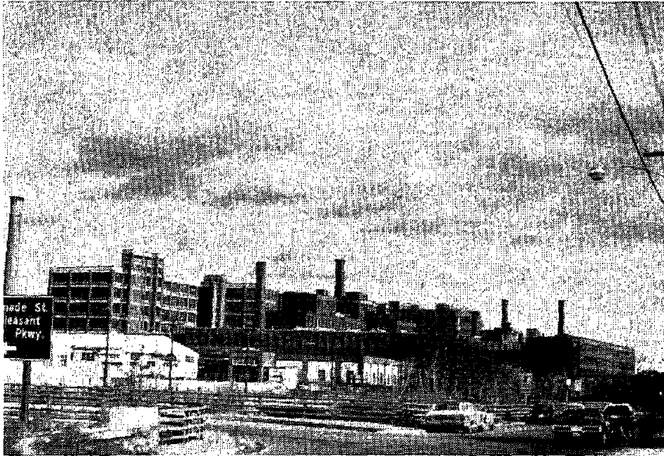
FIGURE 4-5. LARGE INDUSTRIAL URM BUILDINGS, NEW ENGLAND REGION
