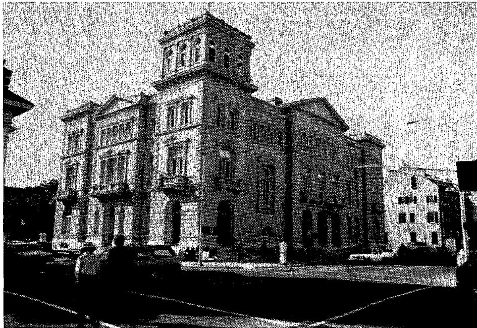
FIGURE 3-14. URM CHURCH PREDATING 1886 EARTHQUAKE IN CHARLESTON, SC.
