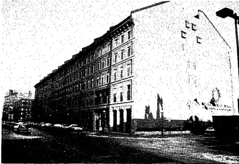
FIGURE 5-1. CONVERTED URM LOFT BUILDING NEW ENGLAND REGION
