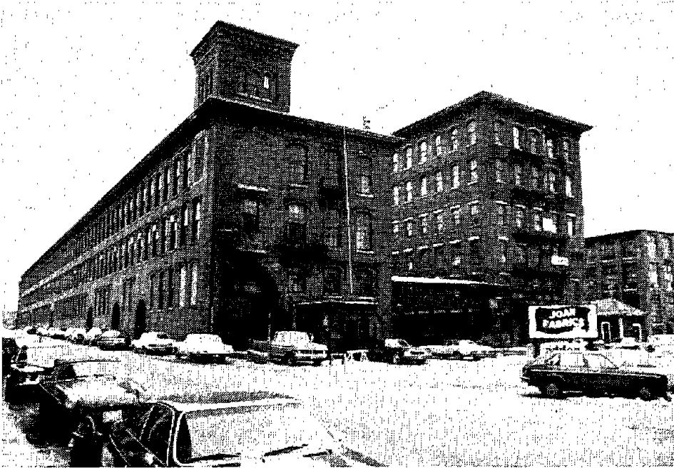
FIGURE 4-15. INDUSTRIAL BUILDING, NEW ENGLAND REGION
