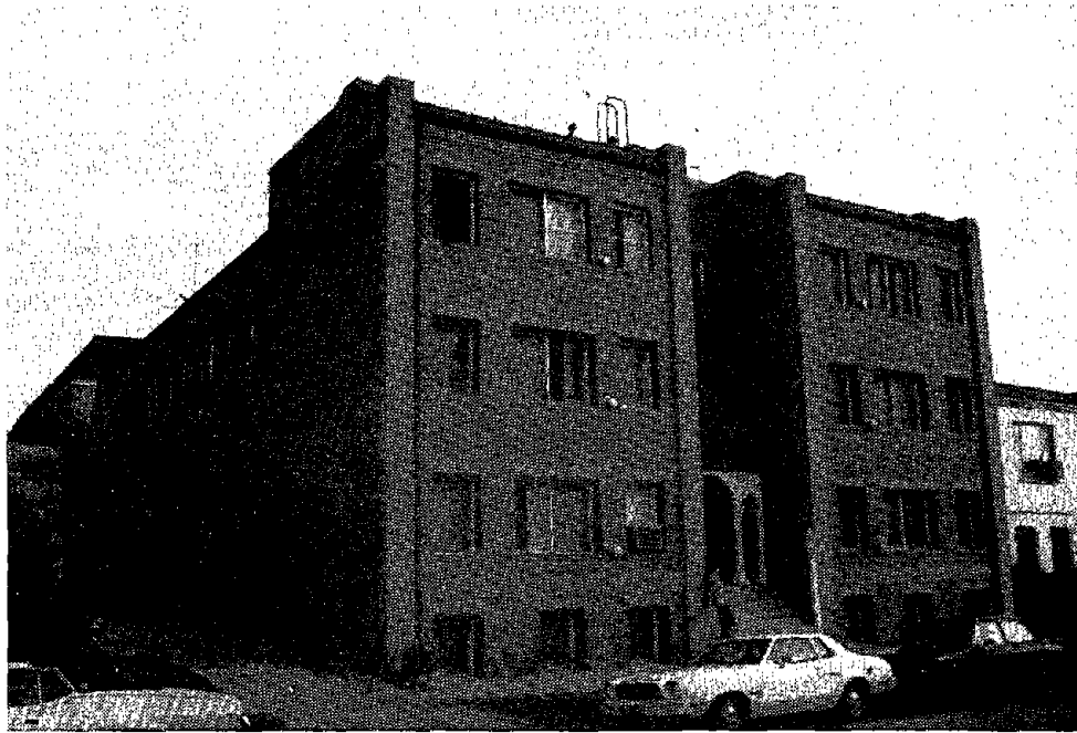
FIGURE 5-5. REPRESENTATIVE URM APARTMENT BUILDING OF MODERATE SIZE
