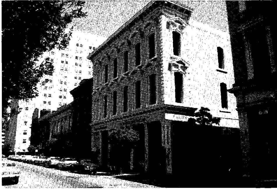
FIGURE 3-80. URM COMMERCIAL BUILDING, SAN FRANCISCO, CA.
