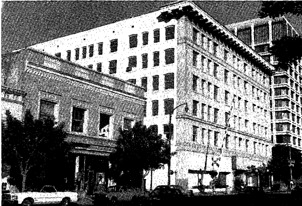
FIGURE 4-2. URM BUILDING WITH CONCEALED STRUCTURAL FRAME
