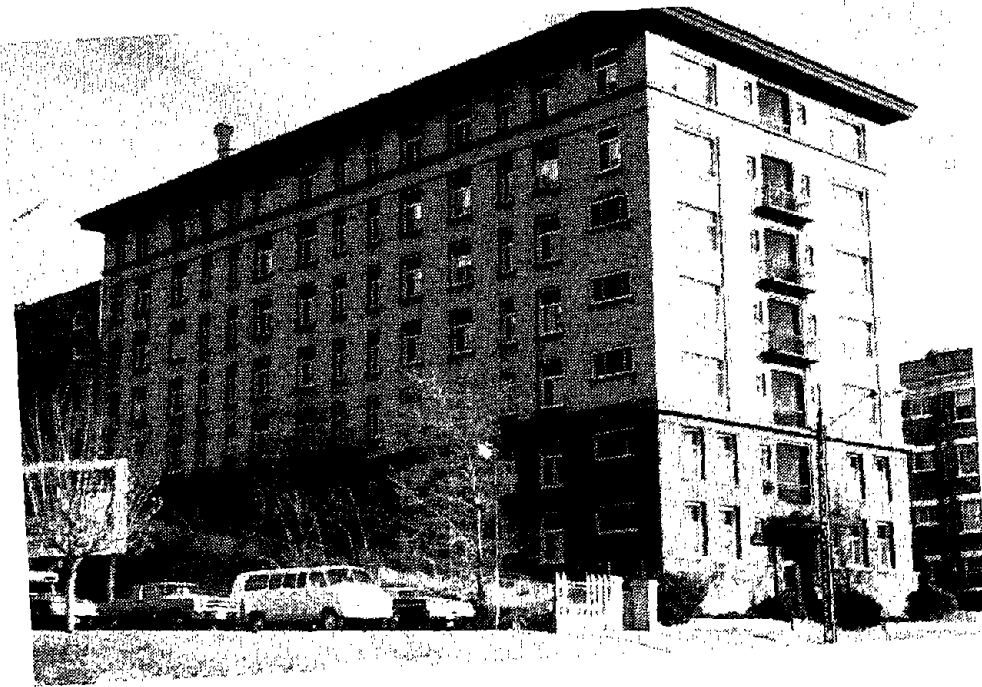
FIGURE 3-51. URM MULTI-FAMILY HOUSING, SALT LAKE CITY, UT.
