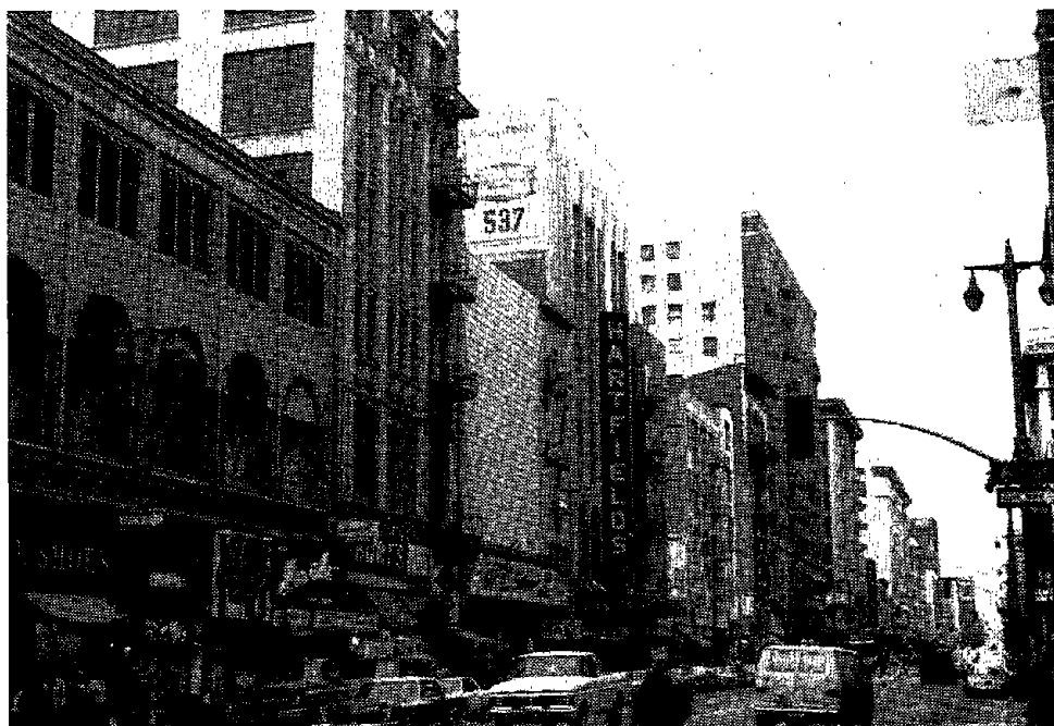
FIGURE 3-79. URM COMMERCIAL BUILDING, LOS ANGELES, CA.
