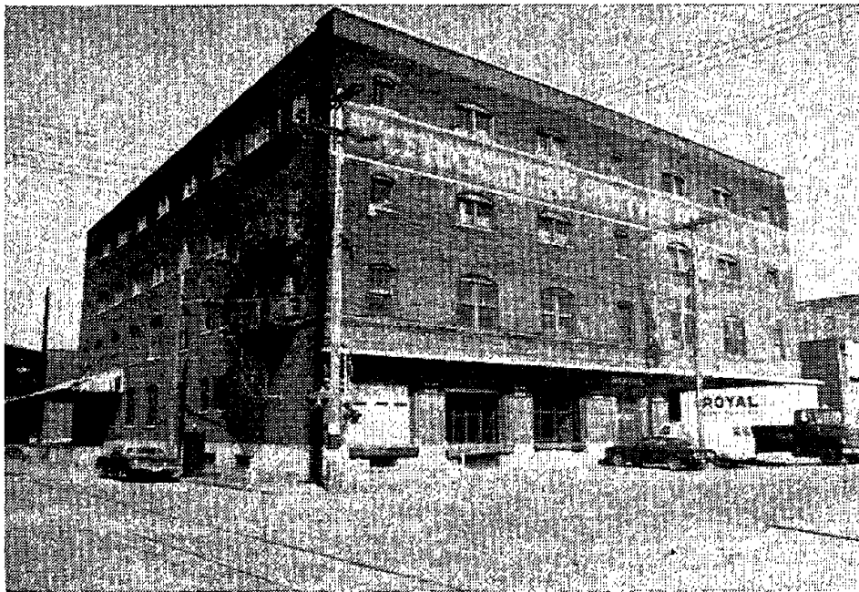
FIGURE 3-27. URM INDUSTRIAL BUILDING WITH INTERNAL CONCRETE FRAME
