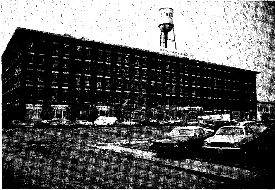
FIGURE 3-39. URM INDUSTRIAL BUILDING, SALT LAKE CITY, UT.
