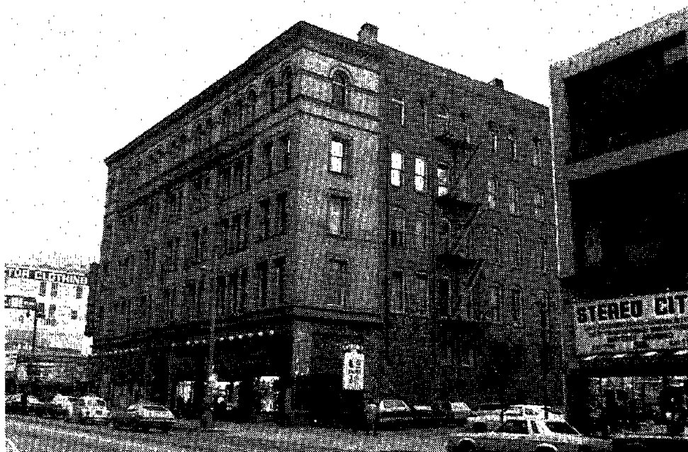
FIGURE 3-77. MEDIUM SIZE OFFICE BUILDING WITH URM WALLS, LOS ANGELES, CA.
