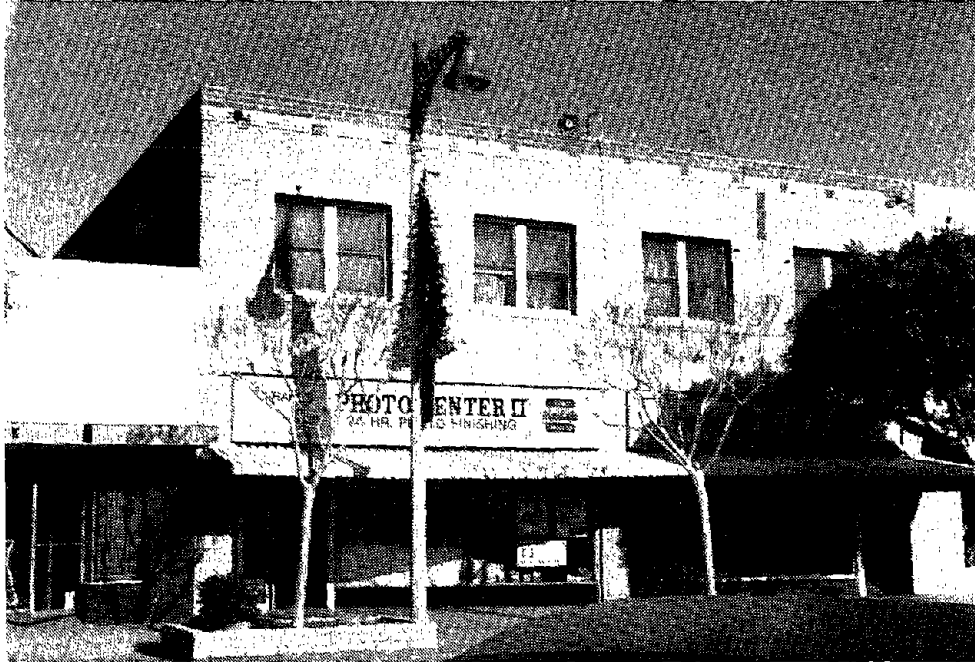
FIGURE 3-72. OPEN FRONT URM BUILDING, SAN FERNANDO, CA.
