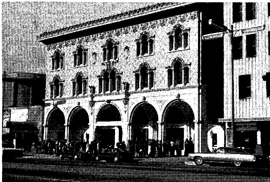
FIGURE 3-47. HISTORIC PRESERVATION OF URM THEATRE SALT LAKE CITY, UT.
