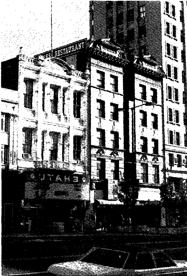
FIGURE 3-41. URM COMMERCIAL BUILDINGS, SALT LAKE CITY, UT.
