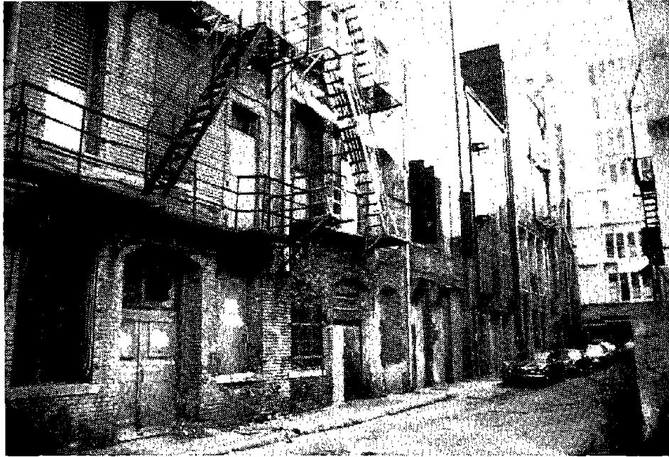
FIGURE 4-13. REAR OF COMMERCIAL BUILDING, MEMPHIS, TN.
