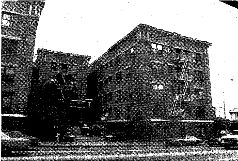
FIGURE 4-8. LARGE URM APARTMENT BUILDING WITH WINGS OF VARIABLE SIZE
