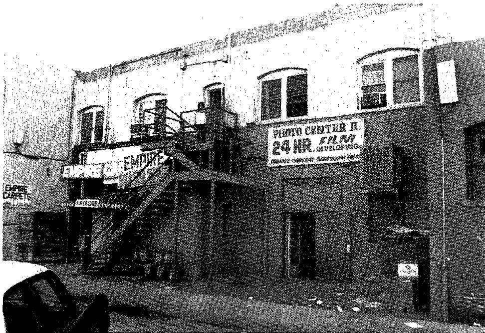
FIGURE 3-73. REAR OF URM BUILDING, SAN FERNANDO, CA.
