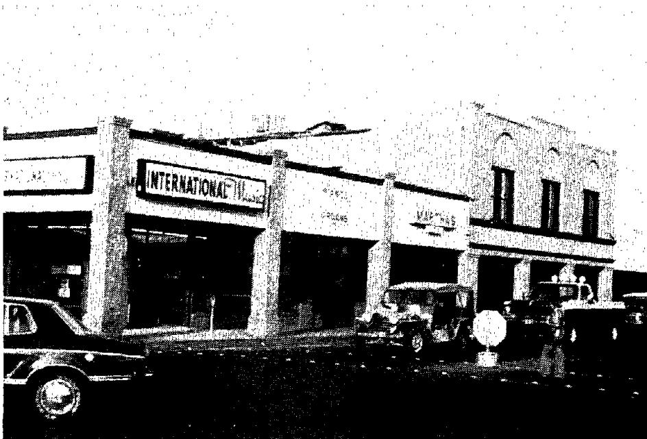
FIGURE 3-71. URM COMMERCIAL BUILDING, EL CENTRO, CA.
