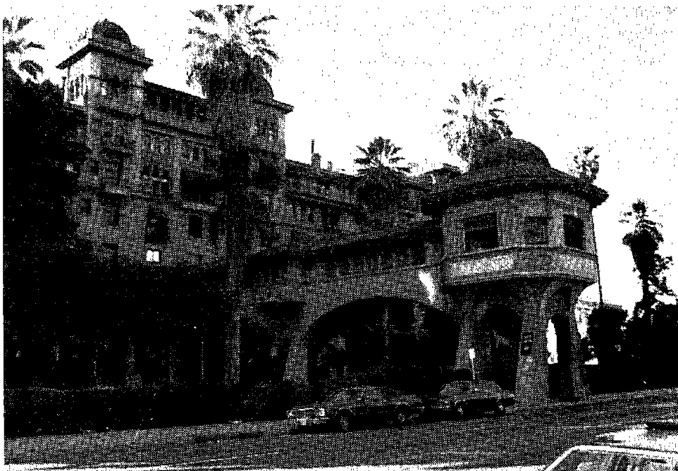
FIGURE 3-82. URM APARTMENT BUILDING, PASADENA, CA.
