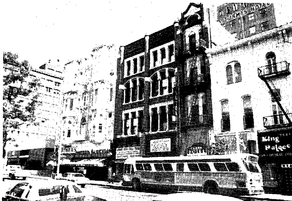
FIGURE 3-78. URM COMMERCIAL BUILDING, SAN DIEGO, CA.
