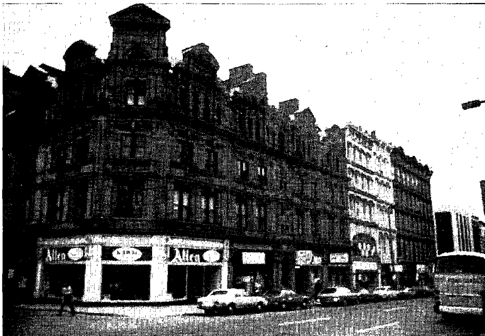
FIGURE 3-7. URM BUILDING, URM PROJECTIONS AT ROOF LEVEL
