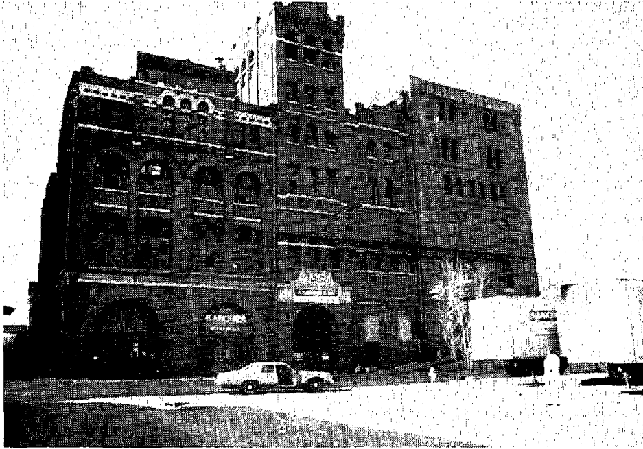
FIGURE 3-23. URM BUILDINGS, INDUSTRIAL DISTRICT, MEMPHIS, TN.
