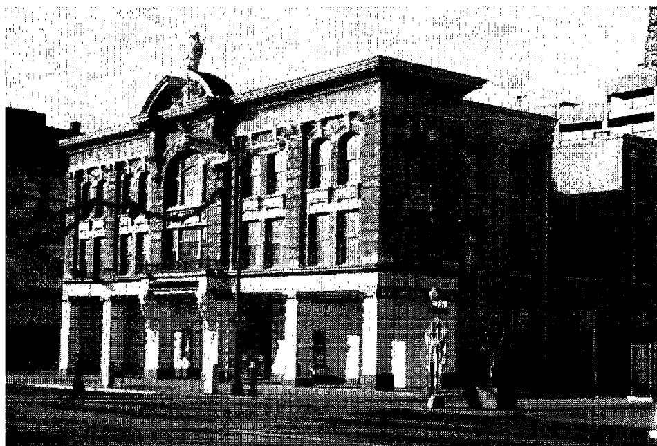
FIGURE 3-48. HISTORIC PRESERVATION OF URM THEATRE SALT LAKE CITY, UT.
