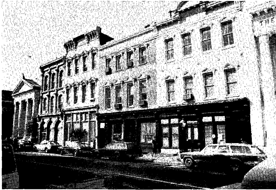
FIGURE 3-13. URM COMMERCIAL BUILDINGS PREDATING 1886 EARTHQUAKE IN CHARLESTON, SC.
