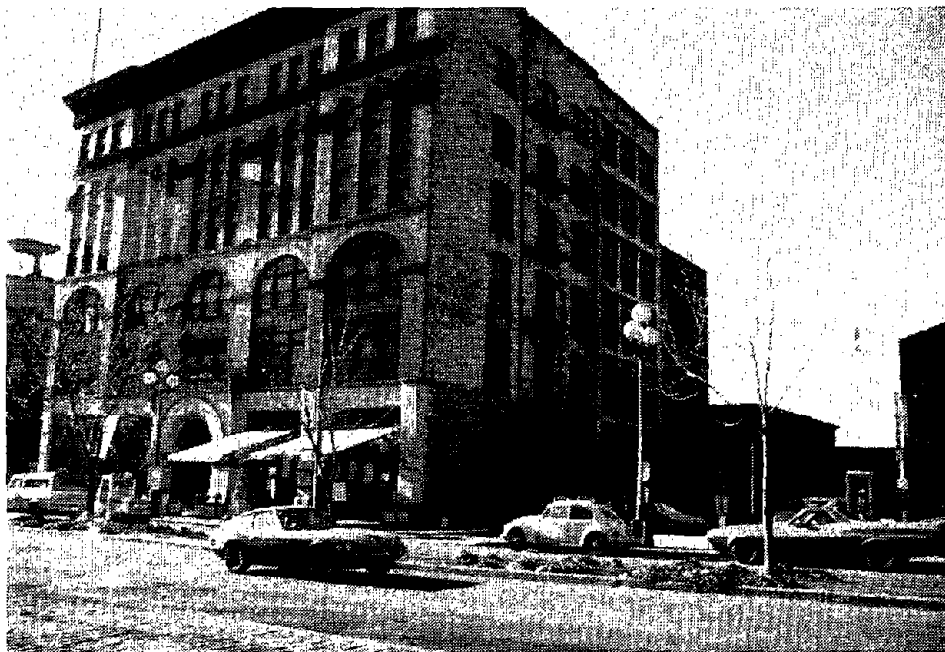
FIGURE 3-61. TYPICAL COMMERCIAL URM BUILDING, SEATTLE, WA.
