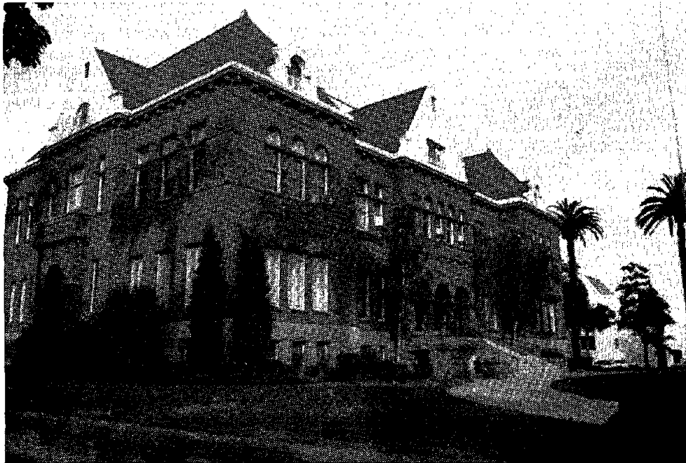
FIGURE 5-4. URM PUBLIC BUILDING CALIFORNIA COAST REGION
