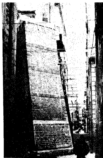
In Naples's Spanish Quarter, buildings were buttressed to protect against failure after the 1980 earthquake
