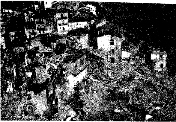
The collapse of older, unreinforced masonry structures often brought down neighboring attached buildings in a characteristic domino effect
