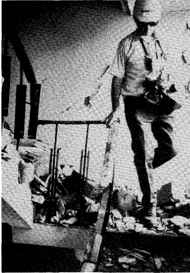
Fig. 2.10 Stairway hazards from debris and broken handrails, Banco Central, 1972 Managua Earthquake. (See also Fig. 2.2) (Photo courtesy of Henry J. Degenkolb.)
