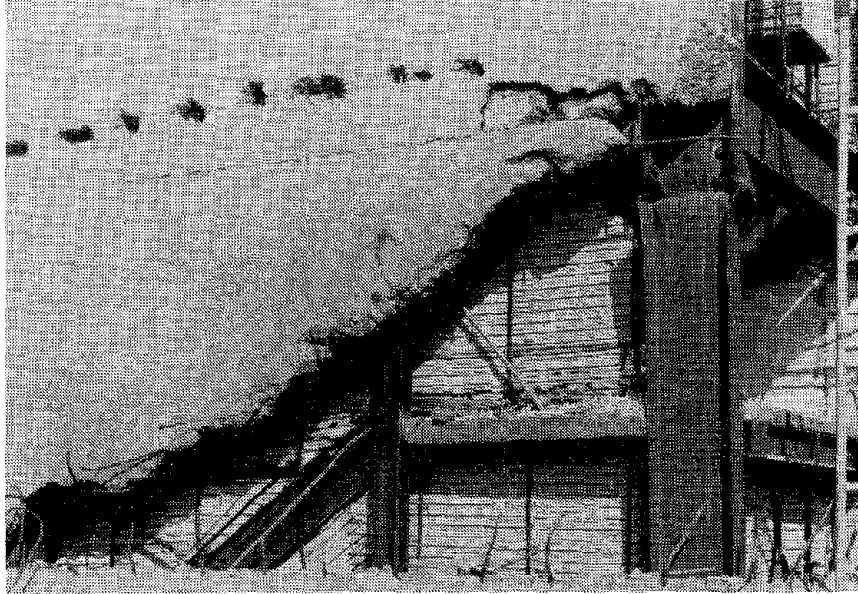
Fig. 2.3 Steel column failure at stair landing, Cordova Building, 1964 Alaska Earthquake. (See also Fig. 2.9) (Photo courtesy of the American Iron and Steel Institute.)
