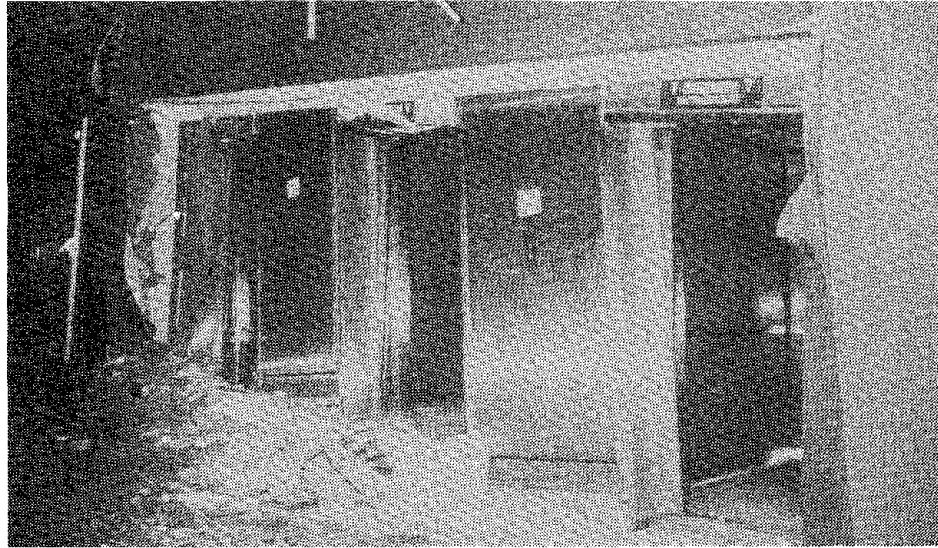
Fig. 4.7 Elevator and service stair lobby, Olive View Hospital, 1971 San Fernando Earthquake. Service stair doorway is visible at the extreme left (see also Fig. 1.1). (Photo reproduced with permission from Engineering Aspects of the 1971 San Fernando Earthquake. )
