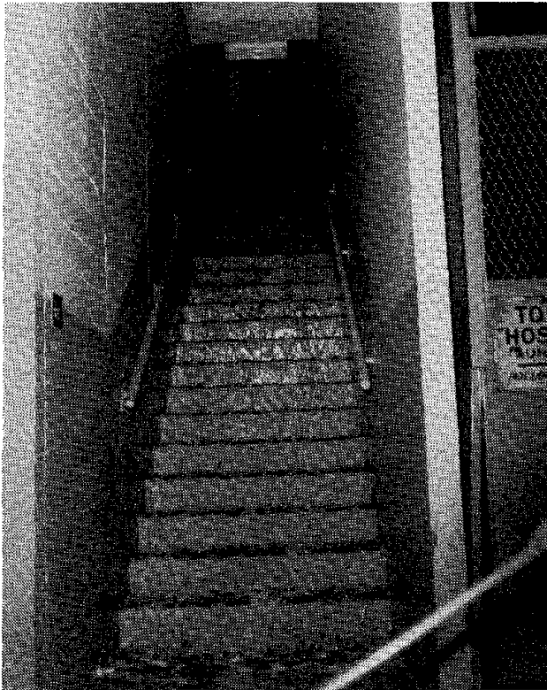
Fig. 2.12 Stairway flooded by broken sprinkler line, Lockheed Building 147, 1971 San Fernando Earthquake. (Photo courtesy of the Lockheed-California Company.)
