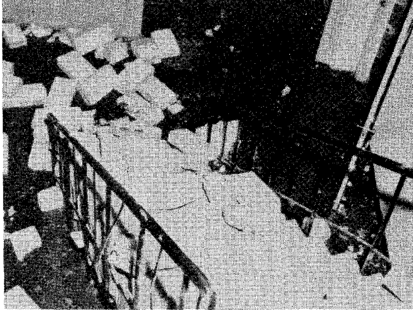
Fig. 2.11 Fatal collapse of masonry walls into stairway, Enlisted Men's Service Club, 1964 Alaska Earthquake. (Reproduced from The Great Alaska Earthquake of 1964--Engineering with permission of the National Academy of Sciences, Washington, D.C.)
