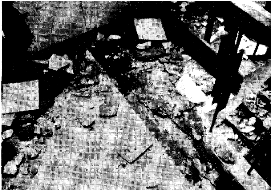
Fig. 2.2 Floor cracking at stair core, Banco Central, 1972 Managua Earthquake. (See also Fig. 2.10) (Photo courtesy of Loring A. Wyllie, Jr.)
