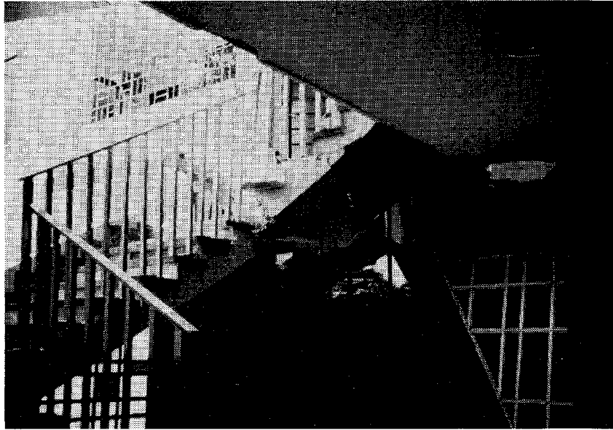
Fig. 4.2 Stair flight damage, San Bosco Building, 1967 Caracas Earthquake. (Photo courtesy of Henry J. Degenkolb.)
