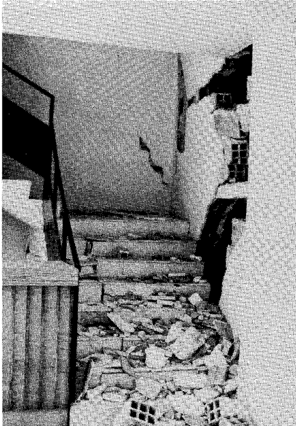
Fig. 2.6 Shattered tile enclosure wall, American School, 1972 Managua Earthquake. (Photo courtesy of Henry J. Degenkolb.)
