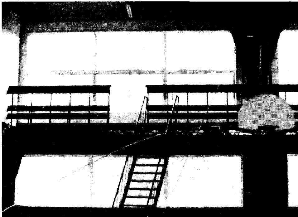
Fig. 5.7 Displaced gallery stair, Shichihyaku Primary School Gymnasium, 1968 Tokachi-Oki Earthquake. (Photo reproduced with permission from General Report on the Tokachi-Oki Earthquake of 1968. )
