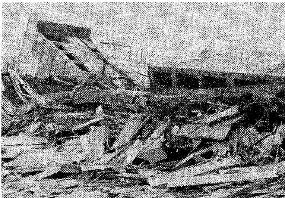
Fig. 5.4 Collapsed structural stair cores, Four Seasons Apartment Building, 1964 Alaska Earthquake. (Ward W. Wells photograph, reproduced with permission from the American Iron and Steel Institute.)
