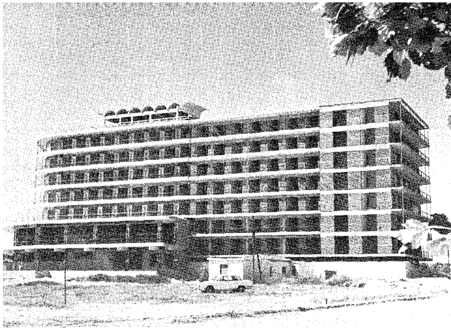
FIGURE 6.17 Galaxy Hotel in Vrahati. North view of the hotel during construction.
