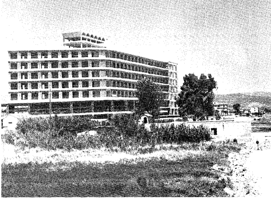
FIGURE 6.16 Galaxy Hotel in Vrahati. Northeast view of the hotel during construction.
