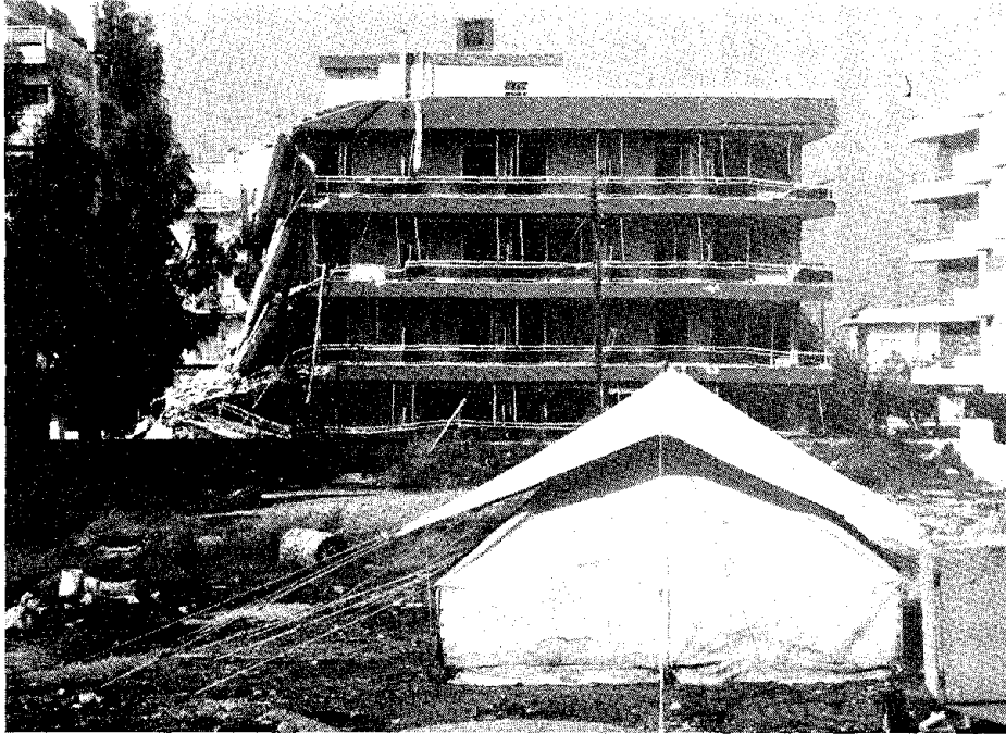
FIGURE 5.2 Partially collapsed five-story block of flats "Segas" in Loutraki. (Note temporary tent shelters in foreground.)
