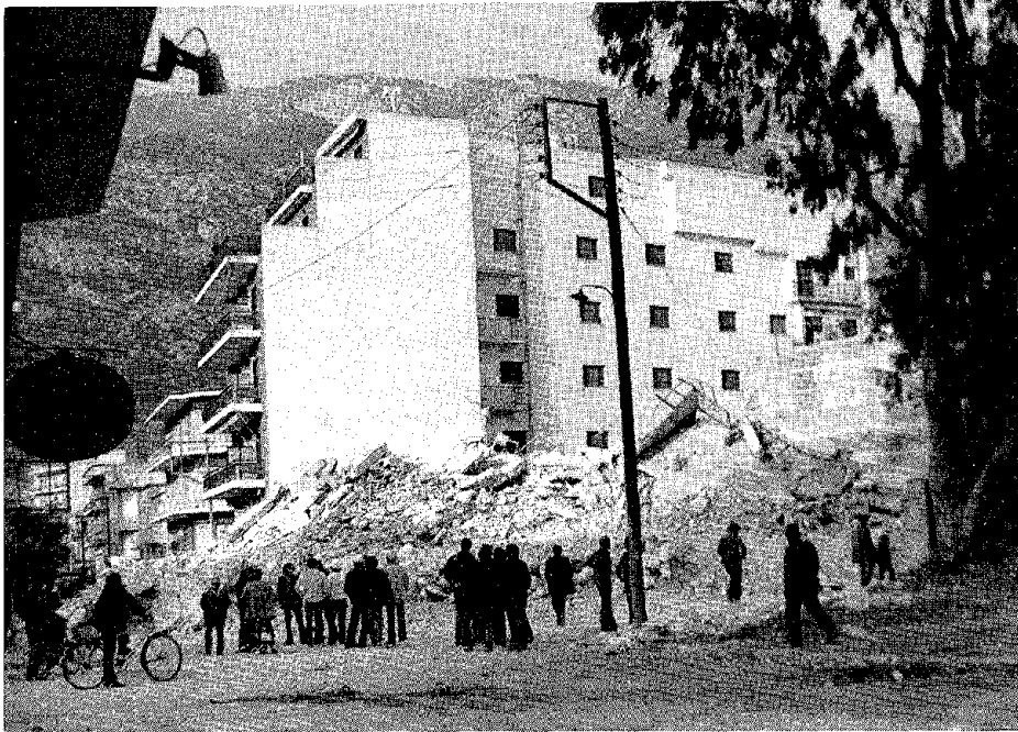
FIGURE 6.8 Contis Hotel in Loutraki. Southwest view one week after collapse. Photograph courtesy A. Manis.
