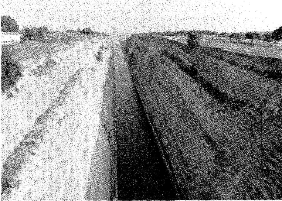
FIGURE 5.14 Corinth canal looking east from the road bridge. Note the descending beddings. At each change of elevation there is a fault.
