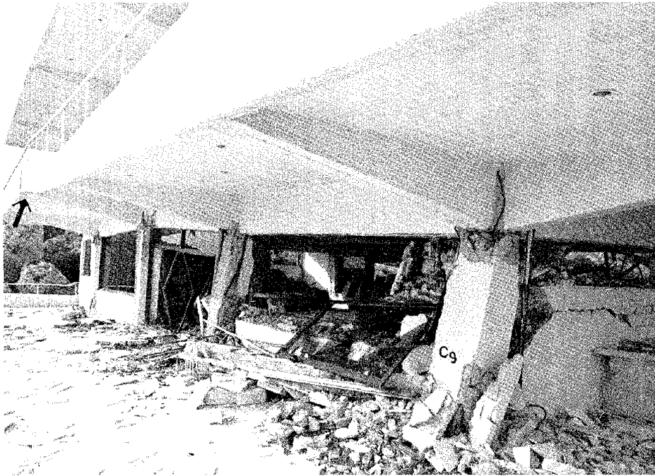
FIGURE 6.4 Vip's Hostel in Perahora. This view from the south shows part of the damaged columns in the second story. The arrow shows the large deformation of the ceiling. There are no ties in the column-to-beam connection ( c_9 ).
