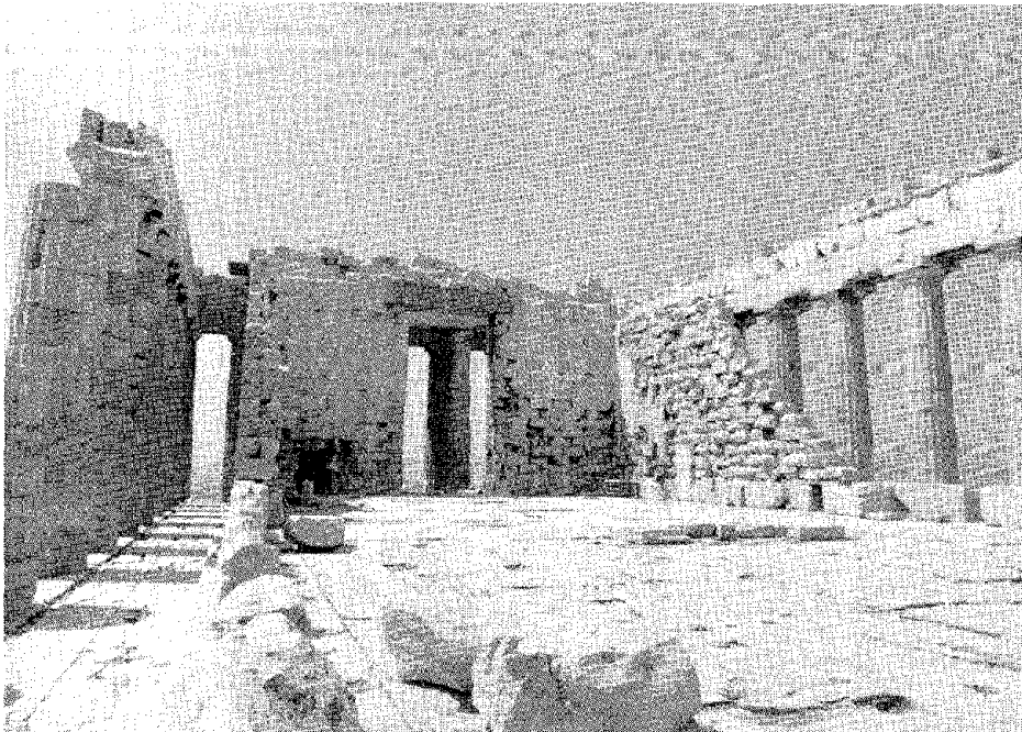
FIGURE 6.46 West side of the Parthenon viewed from the inside. The head beam in the back is connected horizontally by short beams to the inside construction (see Figure 6.42). Source: Dontas (1981).
