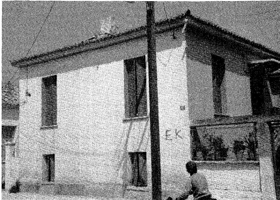
FIGURE 5.28 Some well-maintained earthen buildings in the area, including this one in Kiato, suffered no damage.
