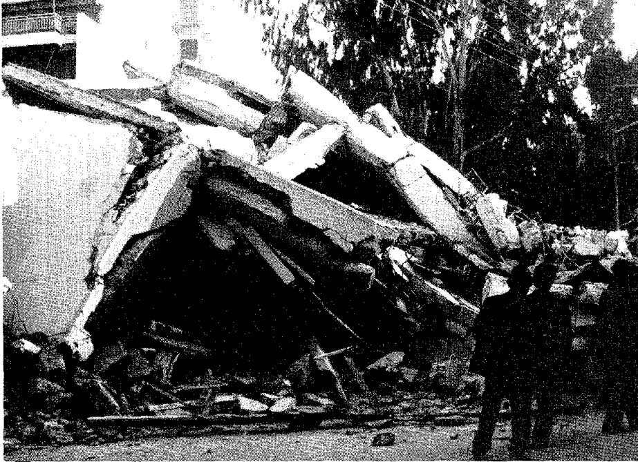
FIGURE 5.6 Collapse of Contis Hotel in Loutraki.
