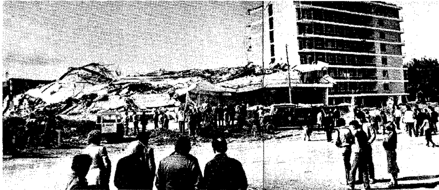
FIGURE 6.20 Galaxy Hotel in Vrahati. View from the east one day after the earthquake and collapse. Photograph courtesy N. Floros.
