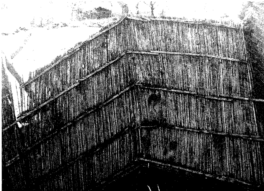
FIGURE 4.2 Timber roof supporting tiles in Perahora.
