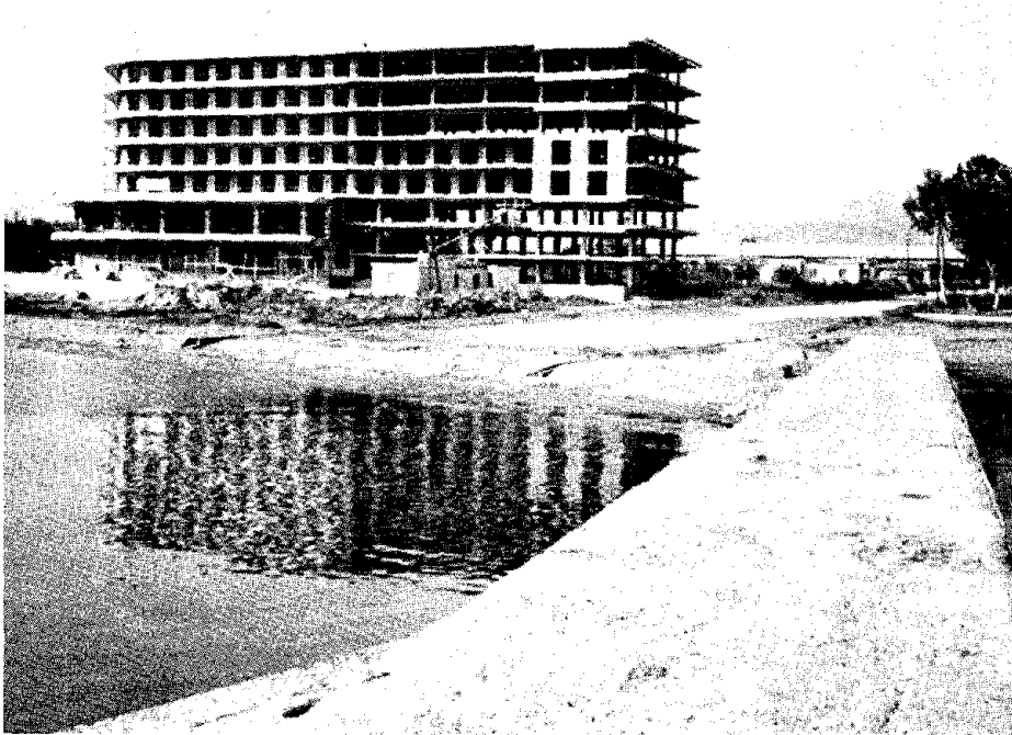
FIGURE 6.18 Galaxy Hotel in Vrahati. North view of the hotel after the earthquake. The remaining part of section III is shown in Figure 6.14a and 6.14b.
