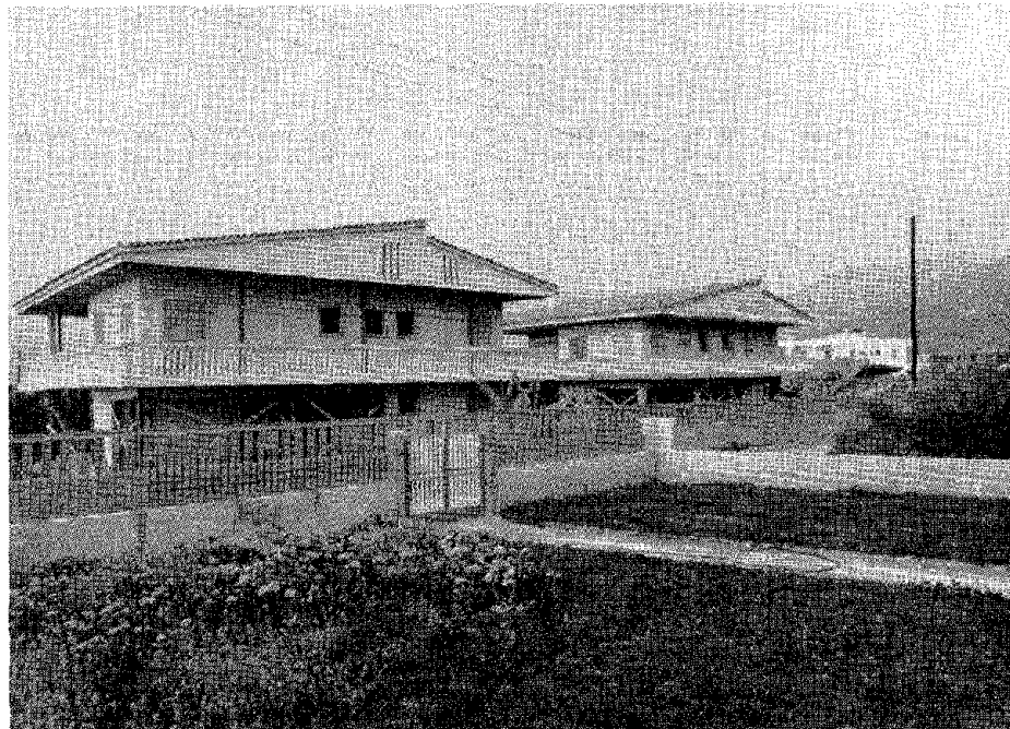
FIGURE 5.12 Three identical two-story buildings in Alepohori showed quite different behavior. The degree of damage increases from left to right. The left building is closer to the sea--no more than 60 m away--and suffered little damage to its first story. The third building collapsed totally (see Figure 5.13).
