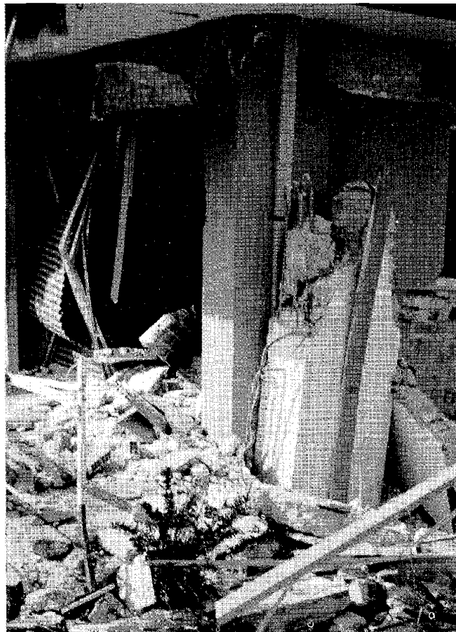
FIGURE 6.40 Block of Flats Segas in Loutraki. As shown by column c_{21} , there is no tie within the height of the column-to-beam connection.
