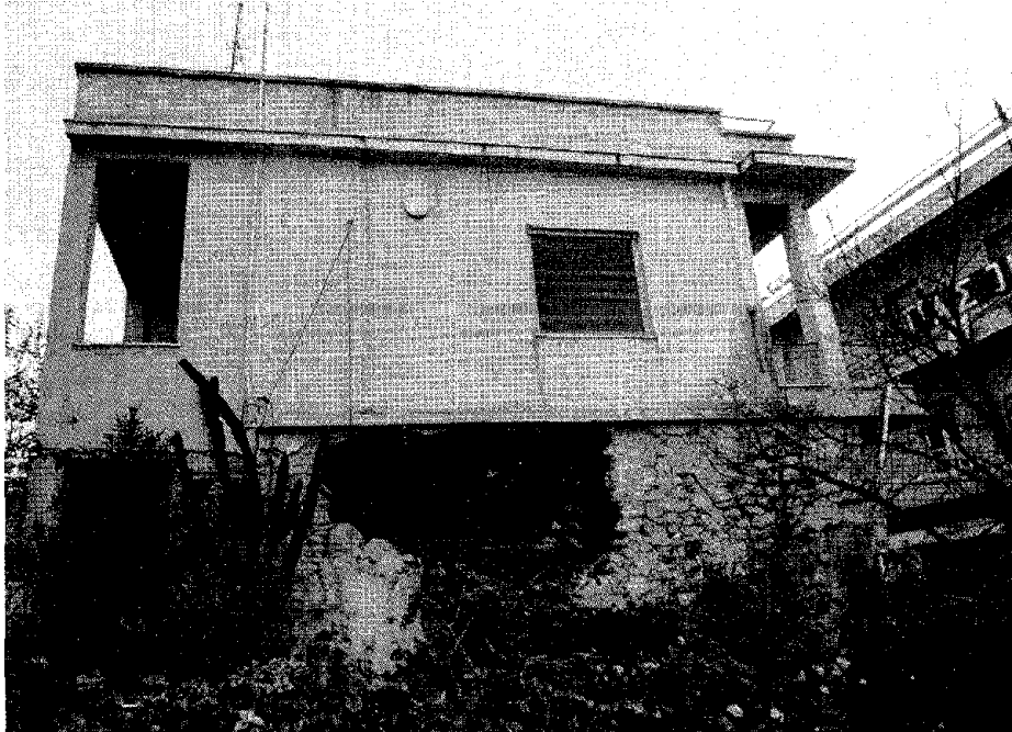
FIGURE 4.5 Addition to an existing stone masonry building (Megara).
