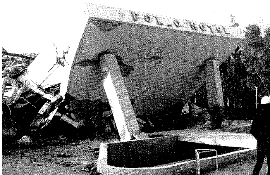
FIGURE 5.7 Collapse of Apollo Hotel in Loutraki.
