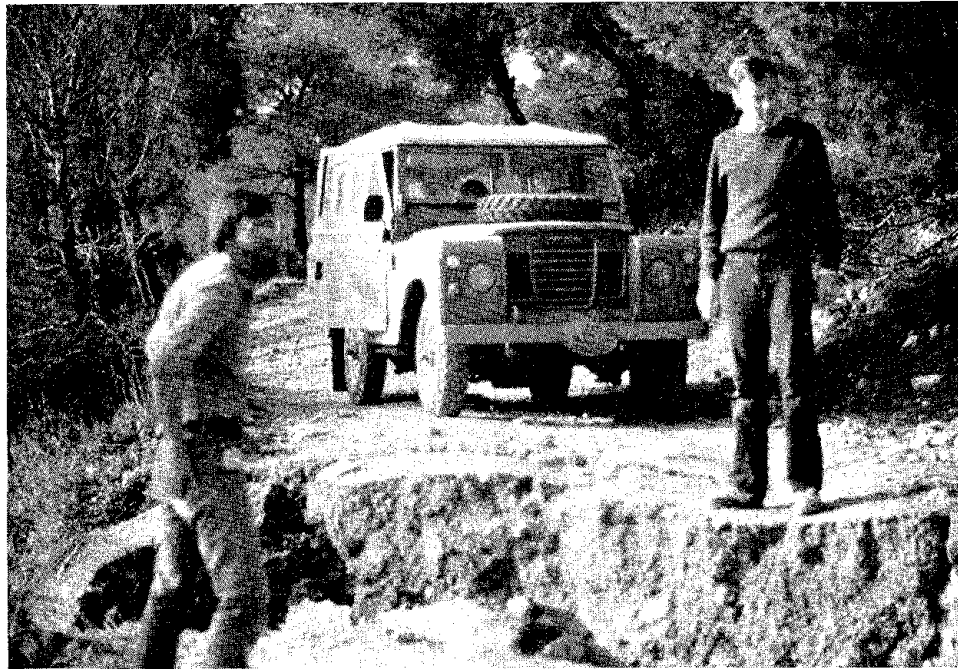
FIGURE 2.8 Vertical offset of road in the central part of the Kalamaki rupture trace.
