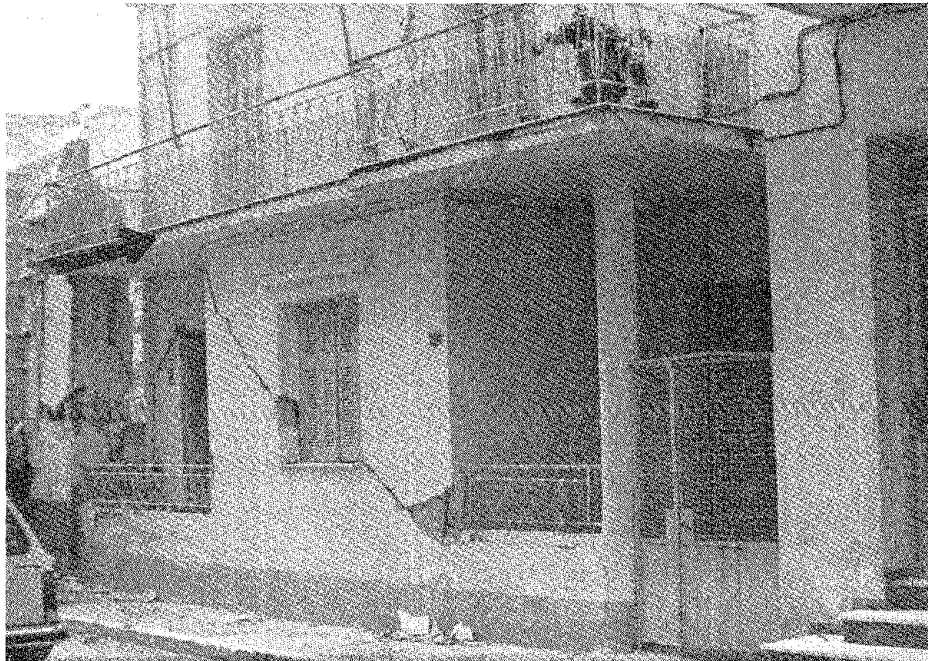
FIGURE 6.13 Contis Hotel in Loutraki. South view. A two-story building was located adjacent to the hotel. The arrow shows the excessive forces transmitted to this structure by the hotel during the rebound. Photograph courtesy A. Manis.
