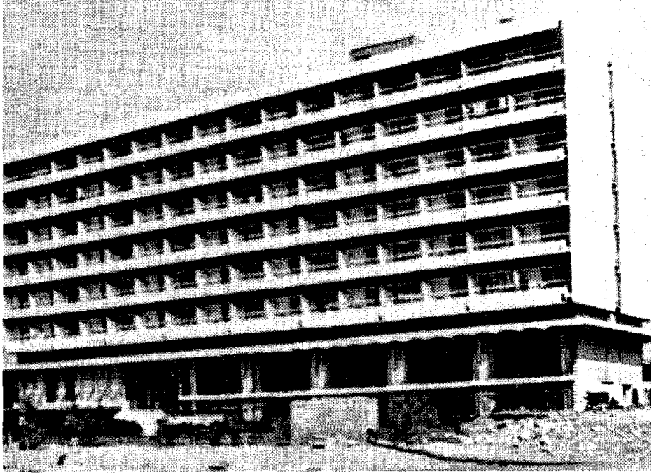
FIGURE 6.29 Apollo Hotel in Loutraki. View from the sea on the west side.
