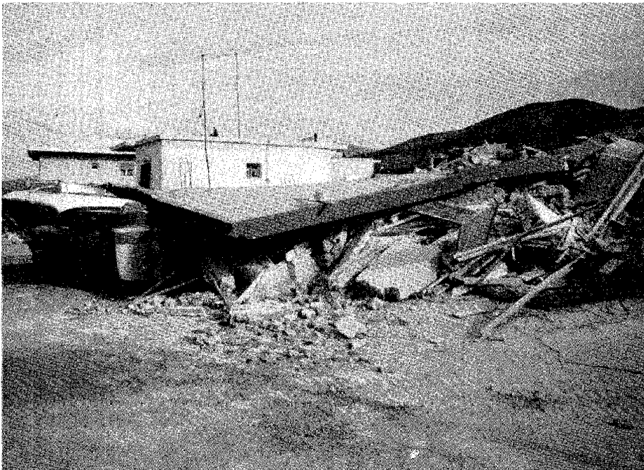
FIGURE 5.44 Building collapse on bus in Plataeae.
