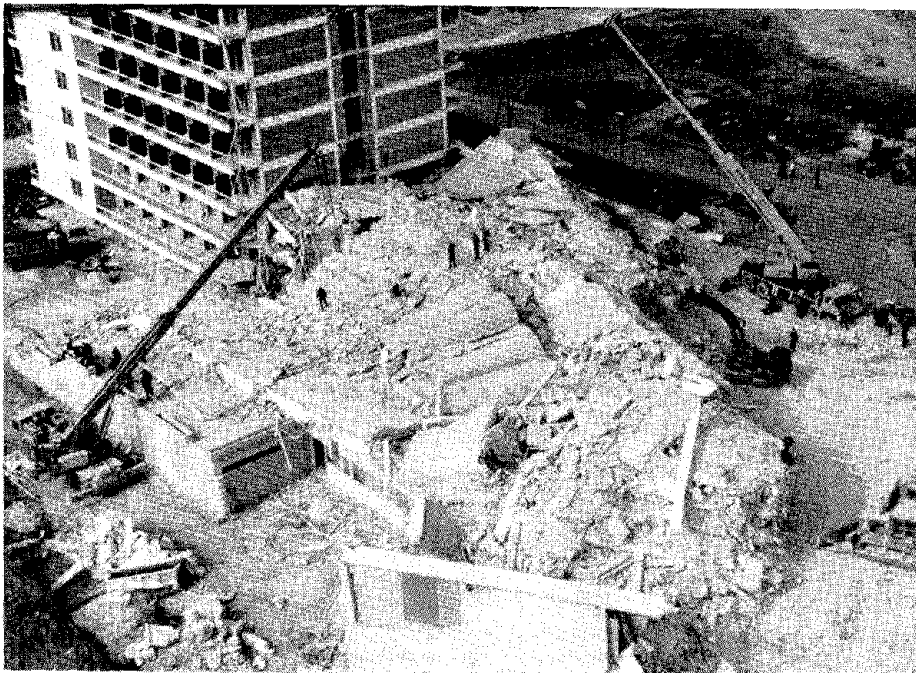
FIGURE 6.19 Galaxy Hotel in Vrahati. Aerial view from the south of the collapsed sections I and II (see Figure 6.14) a few days after the earthquake. Photograph courtesy Tachydromos magazine.
