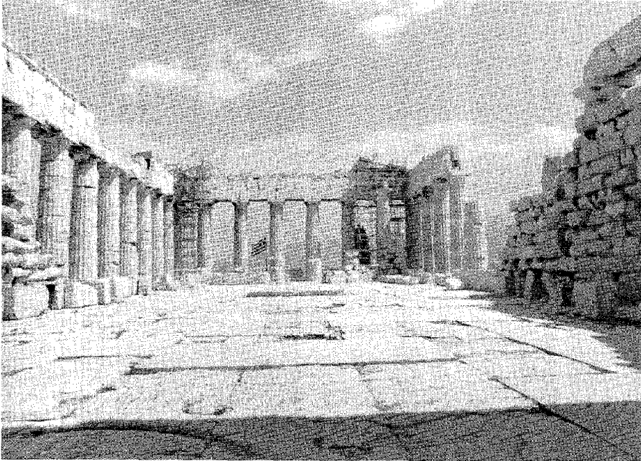
FIGURE 6.45 East side of the Parthenon viewed from the inside. The head beam is supported horizontally only at its two ends. The most damage was concentrated around these two points. Source: Dontas (1981).
